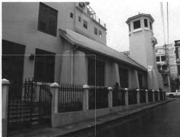
Fig. 10 Buttress on the West façade
