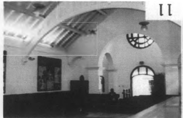
Fig. 3 Recent photograph central arch
