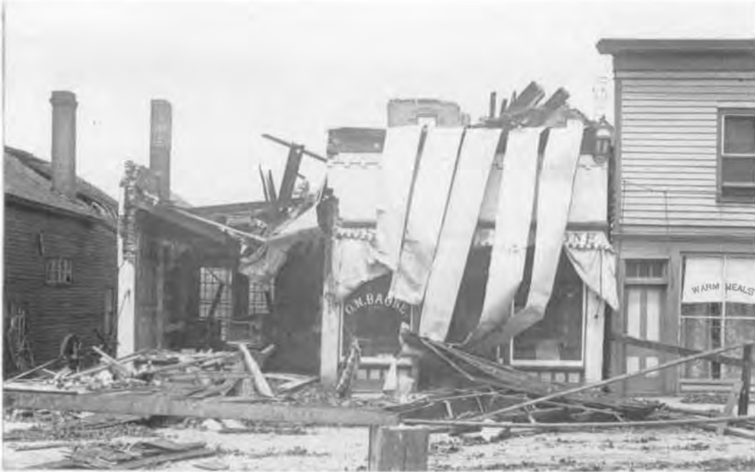
Figure 3 Water Street damage from the 1908 tornado is seen here, with roofing from one building blown atop another and one building completely demolished. This appears to be toward the west end of the district. Porter House Collection.
