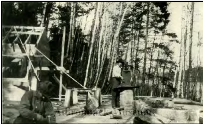
Figure 10. Construction of Banghart Camp, circa 1912; Thomas Lahey and Dinwood Parker building the fireplace. (Adirondack Museum)
