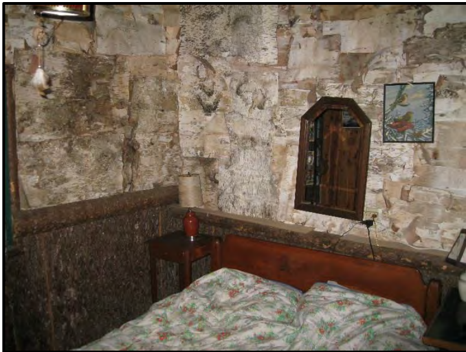
Figure 5. First floor bedroom, 2016.
