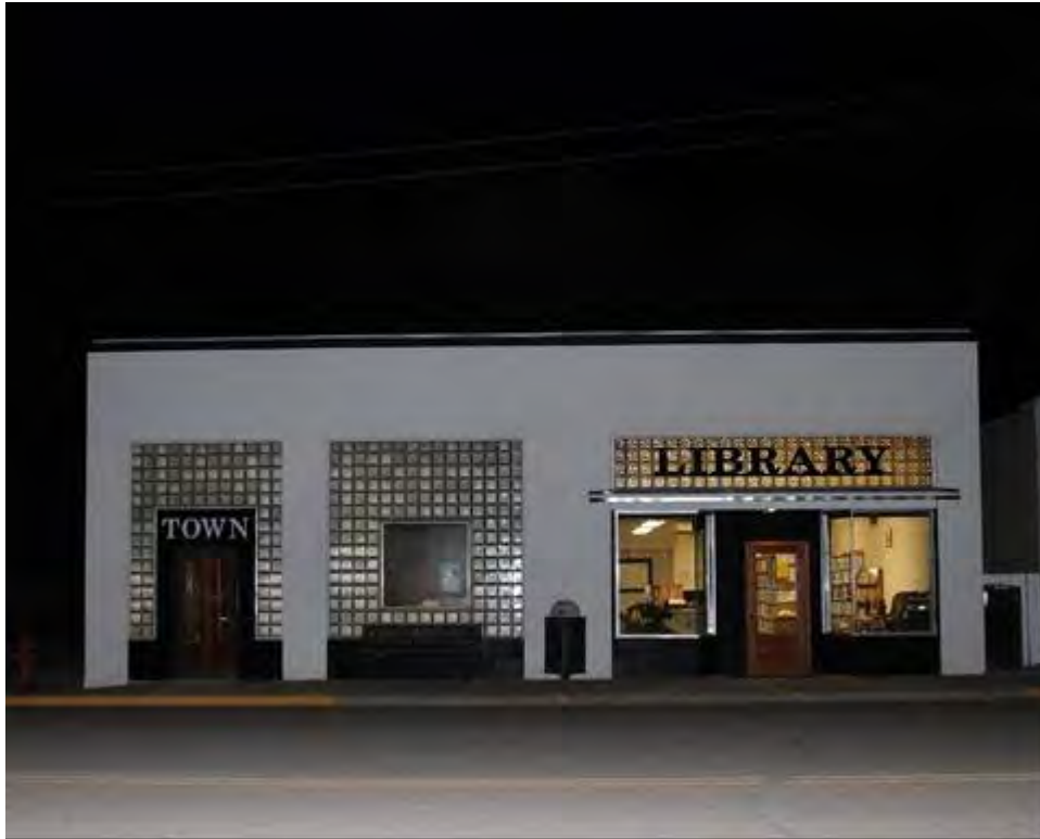
Description of Photograph: South Elevation at night, view to the North. Photo No. MT_CarterCounty_FirstNationalBankOfEkalakaAnd RickardHardwareStoreBuilding_0010
