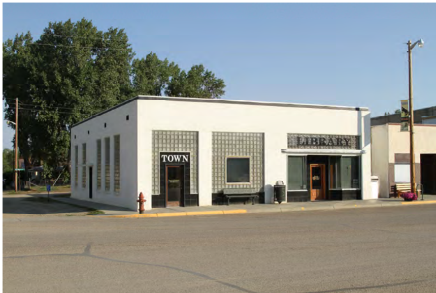
Description of Photograph: South Elevation, view to the North.
