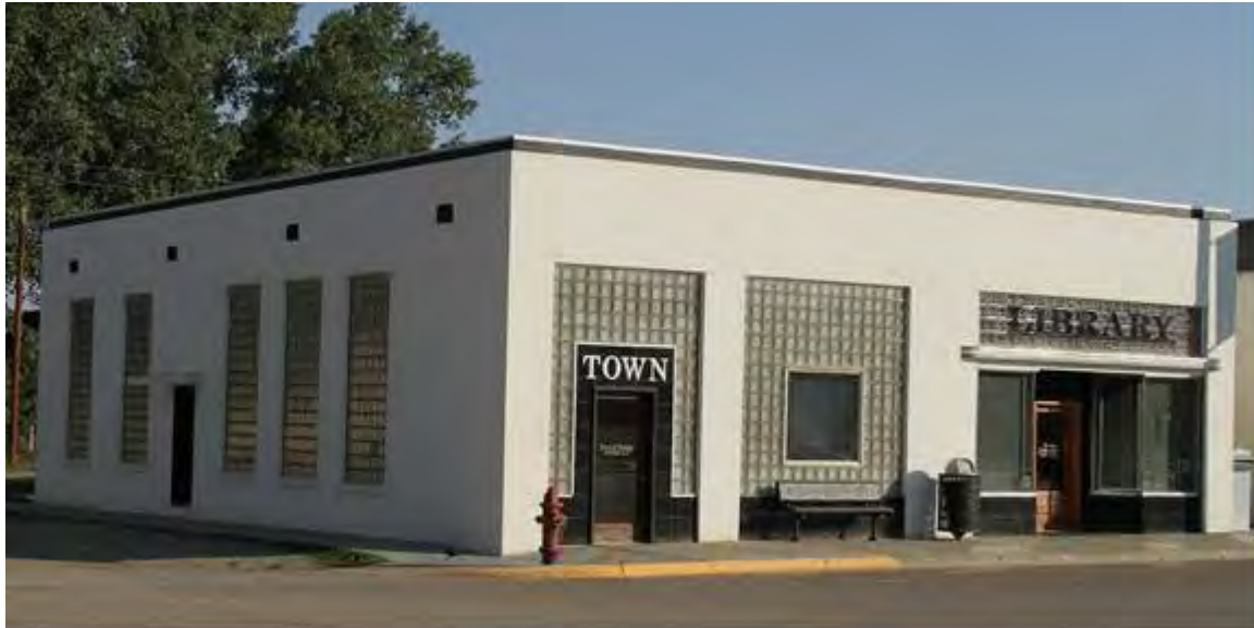
Description of Photograph: West and South Elevations, view to the North.
