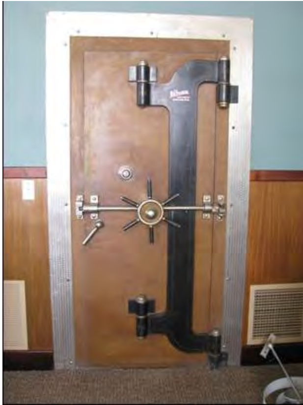
Description of Photograph: Close up of Interior of historic bank (now townhall) showing National Vault.
