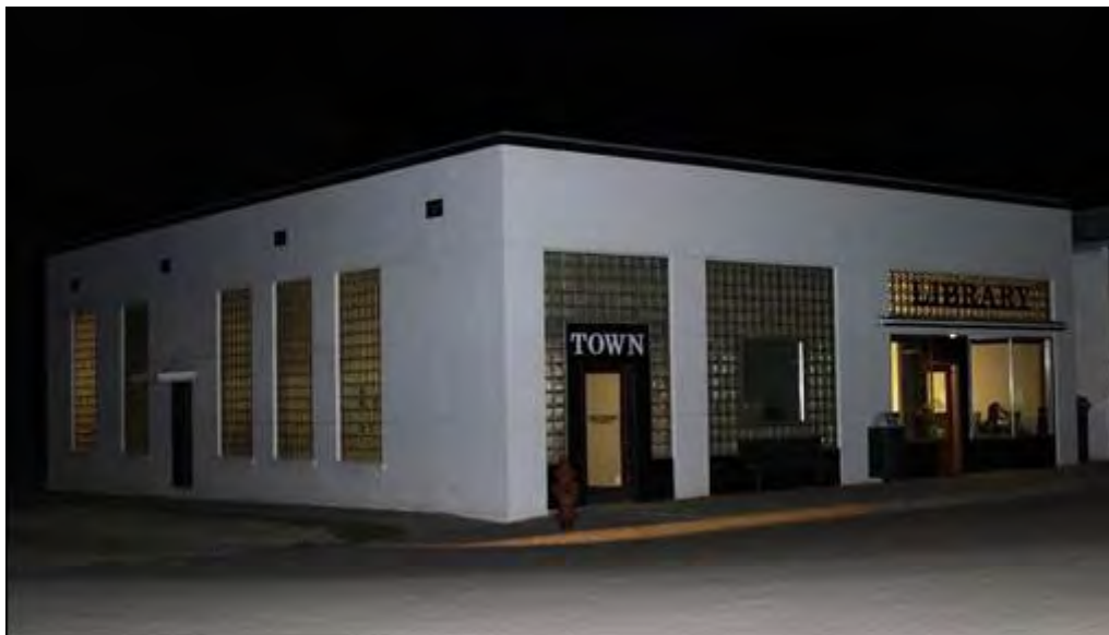
Description of Photograph: West and South Elevations at night, view to the North. Photo No. MT_CarterCounty_FirstNationalBankOfEkalakaAnd RickardHardwareStoreBuilding_0005
