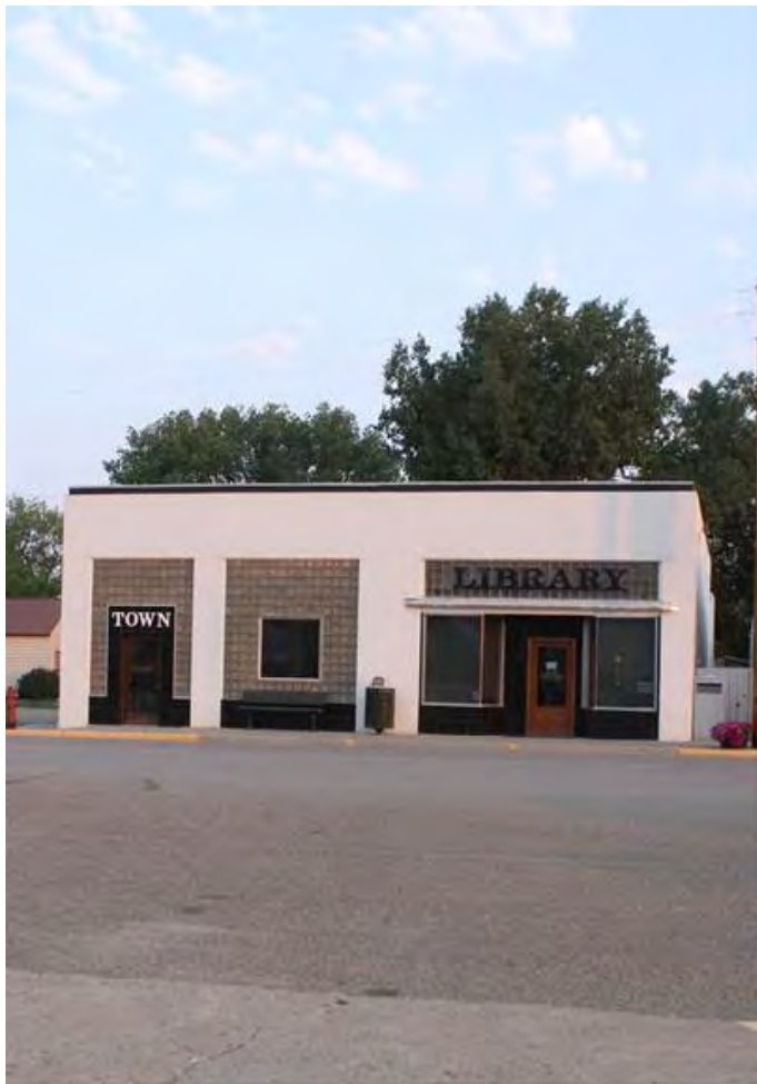
Description of Photograph: South Elevation, view to the Northwest. Photo No. MT_CarterCounty_FirstNationalBankOfEkalakaAnd RickardHardwareStoreBuilding_0001
