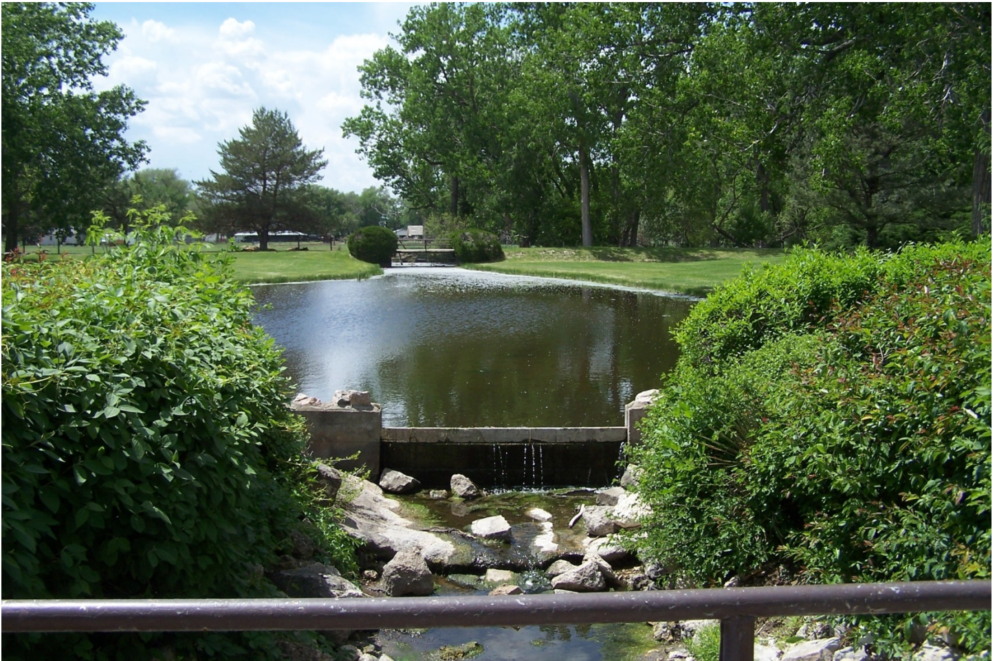
SCOUT'S REST RANCH HEADQUARTERS, North Platte, Nebraska Diversion Dam and Diversion Pond Photo by Hannah Braun, May 2014
