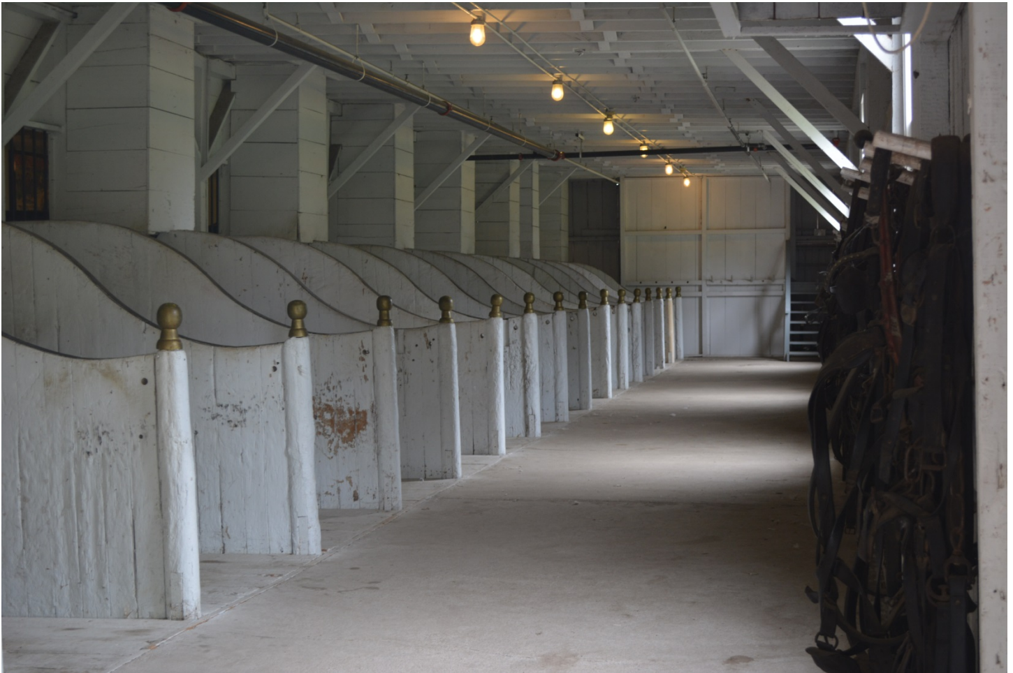
SCOUT'S REST RANCH HEADQUARTERS, North Platte, Nebraska Horse Barn first floor interior, horse stalls Photo by Hannah Braun, June 2015
