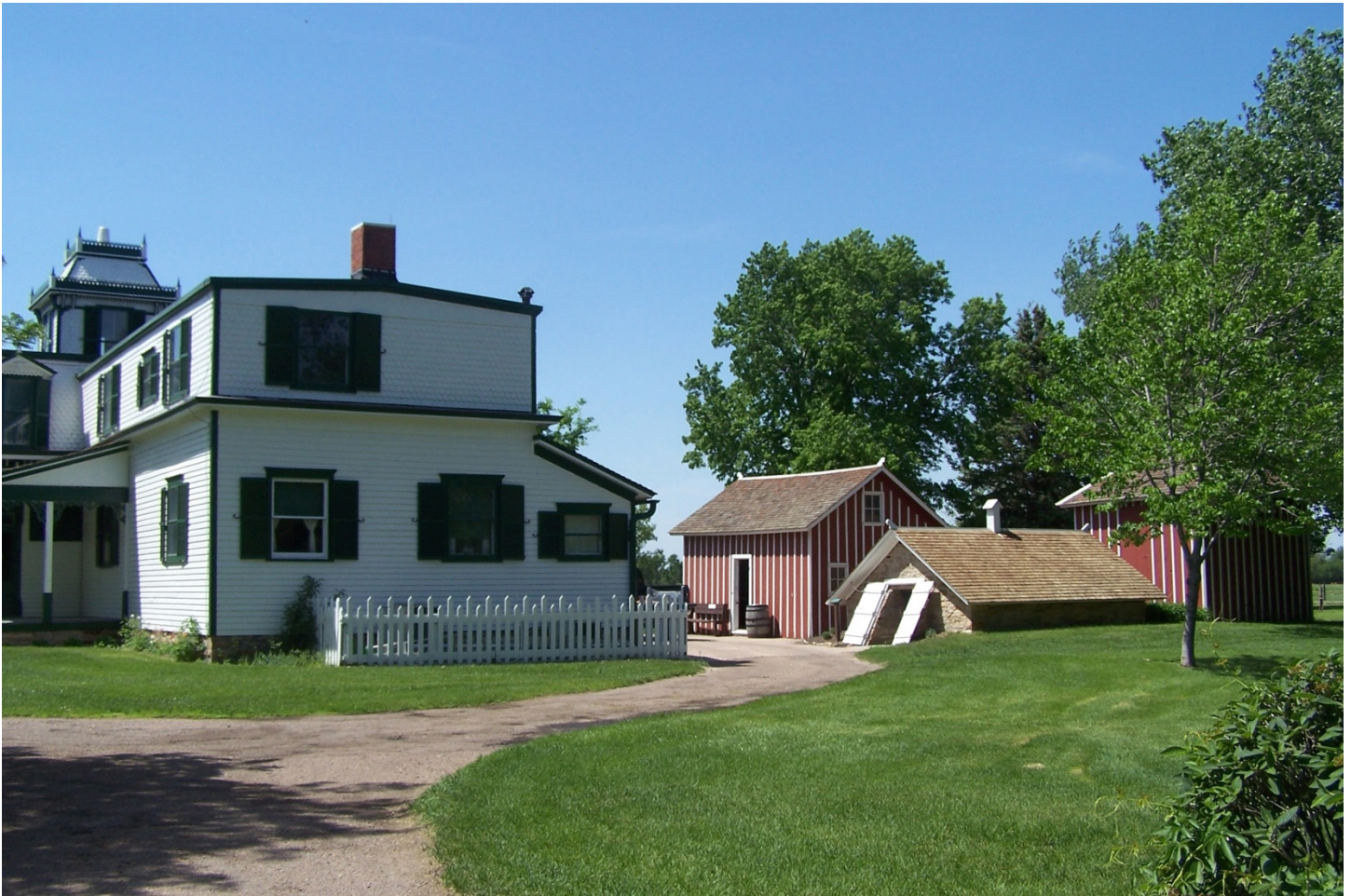
SCOUT'S REST RANCH HEADQUARTERS, North Platte, Nebraska Left to right: Ranch House north (rear) elevation; Cob House; Springhouse/Cellar and Ice House Photo by Hannah Braun, May 2014
