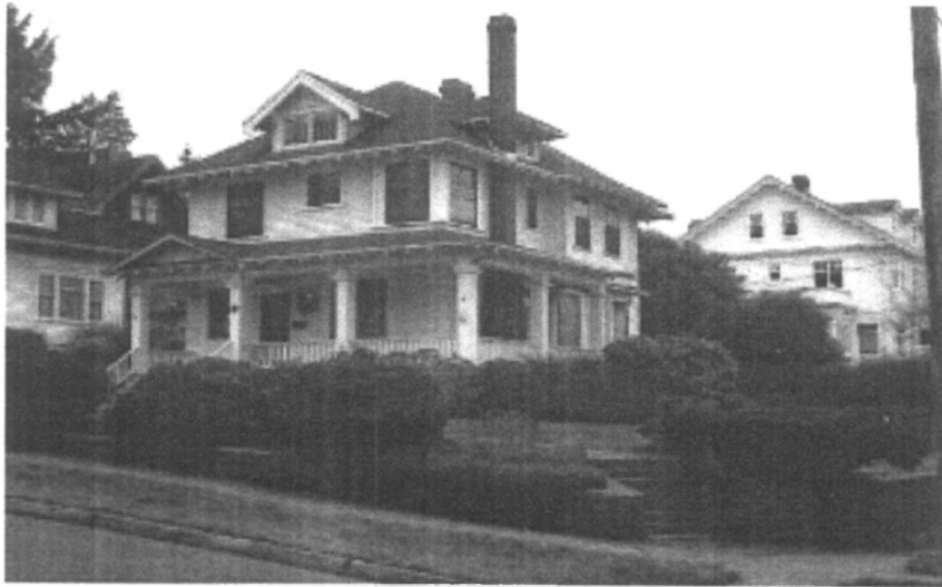
A) Norris Staples residence ca. 1908.
