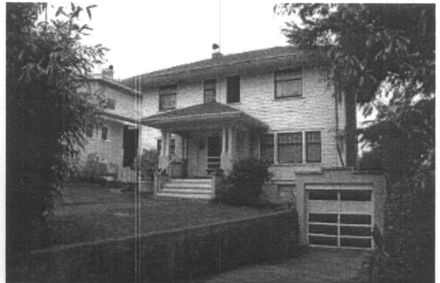
John E. Wicks designed this house in 1921 for Charles Wirkkala.
