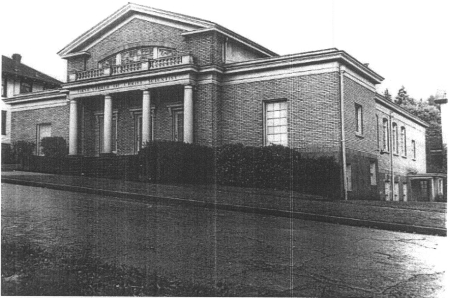
The First Church of Christ Scientist was designed in 1922. (photo courtesy of Clatsop County Historical Society) Fig. 19
