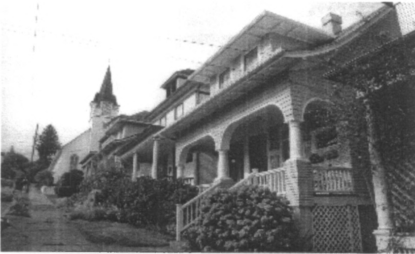
B) Alexander Gilbert rowhouses were constructed in 1905. St. Mary's Catholic Church (1901) is in the background. Fig. 18
