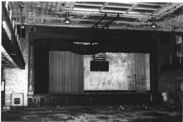
New Jersey Morris County River Street School Photo #9 of 9
