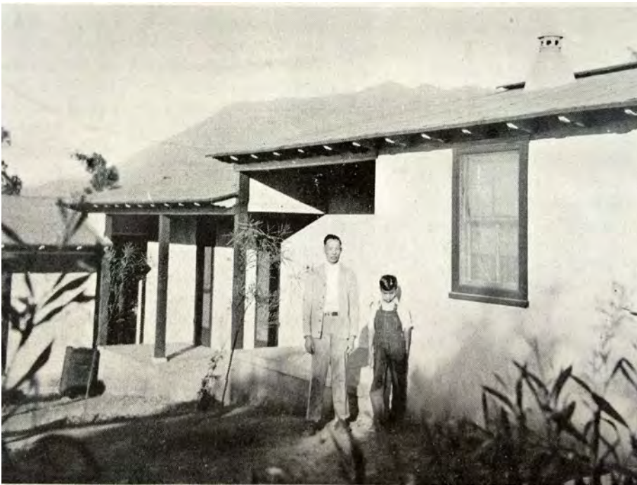
The newly-completed Chinese Quarters, now known as the Health Center. View looking west, 1932. Source: The Thacher Notes .
