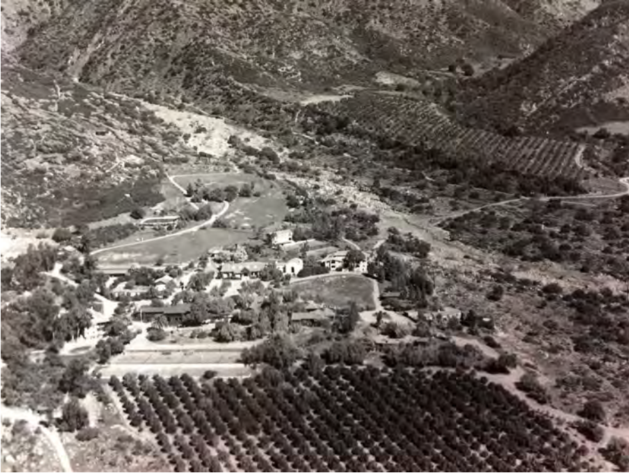
Aerial view looking north across campus, 1940. Courtesy of the Thacher School.
