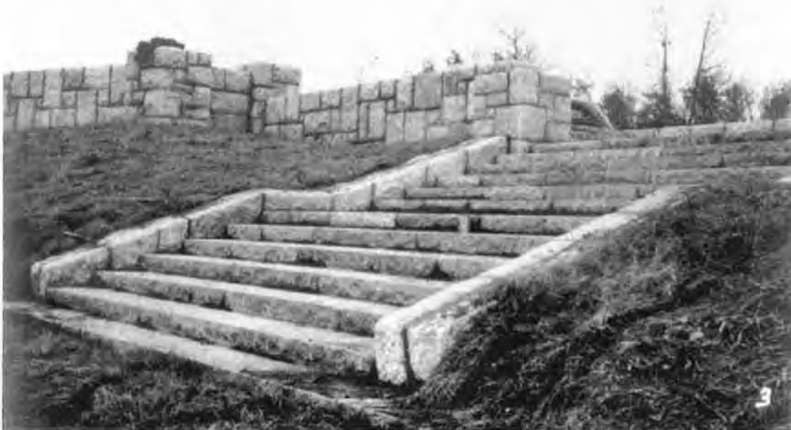
Figure 4. The granite staircase descending to the lakeshore. The photo was taken before the site was planted (1939 photo by the Minnesota Dept. of Highways, A. R. Nichols photo album, Vol. 5, Site Development Unit, MnDOT, St. Paul).
