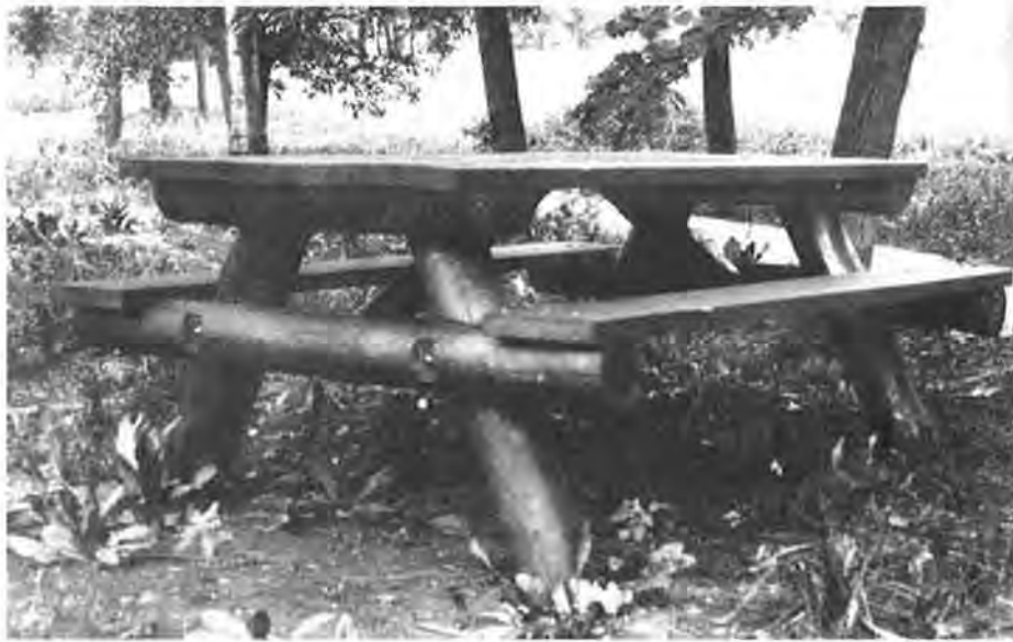
Figure 7. Standard log and plank picnic table used by the Minnesota Department of Highways Roadside Development Division on state highway wayside rests of the 1930s. Two or three of these tables were probably placed at Kenney Lake Overlook. Most of the tables were built for the Division by the National Youth Administration (circa 1940 photo by the Minnesota Dept. of Highways, location unknown, Site Development Unit, MnDOT, St. Paul.
