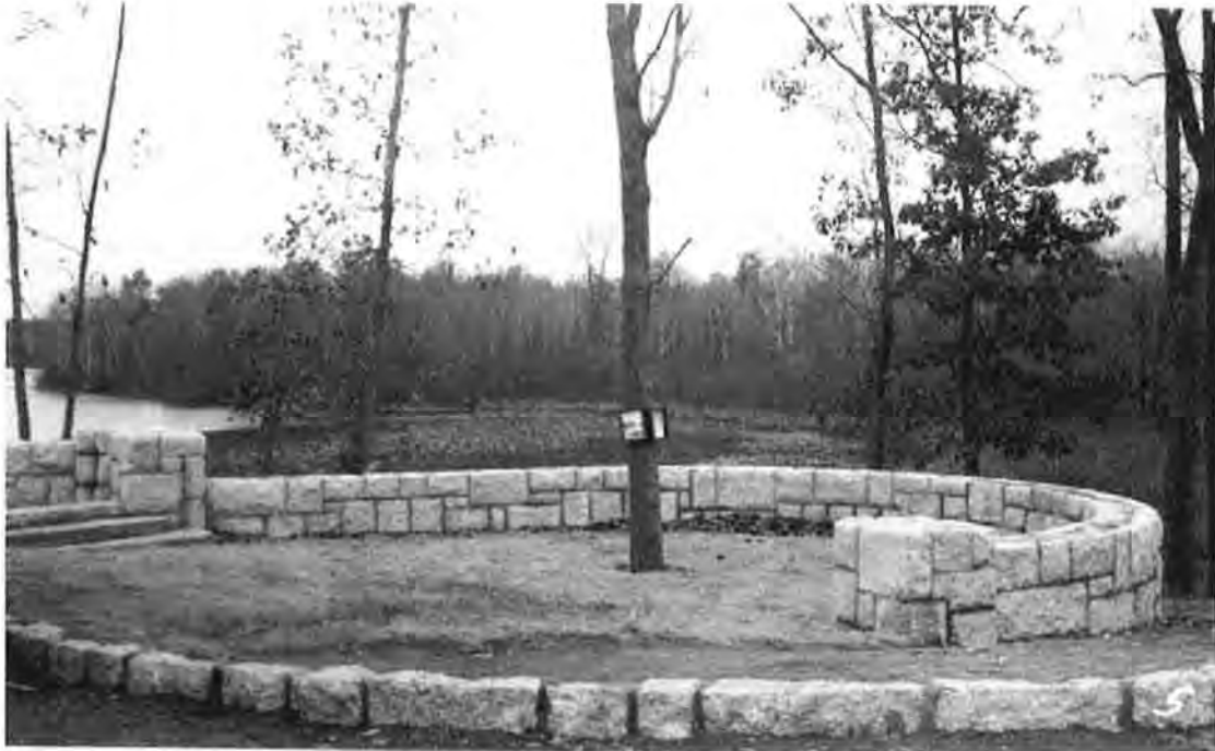
Figure 5. The niche at the northwest end of the overlook wall. The original plans specify preservation of the 10-inch-diameter oak tree in the center of the niche. In the foreground is the granite curbing along the parking area (circa November 1939 photo by the Minnesota Dept. of Highways, Harold E. Olson photo album, Vol. 1, Site Development Unit, MnDOT, St. Paul).
