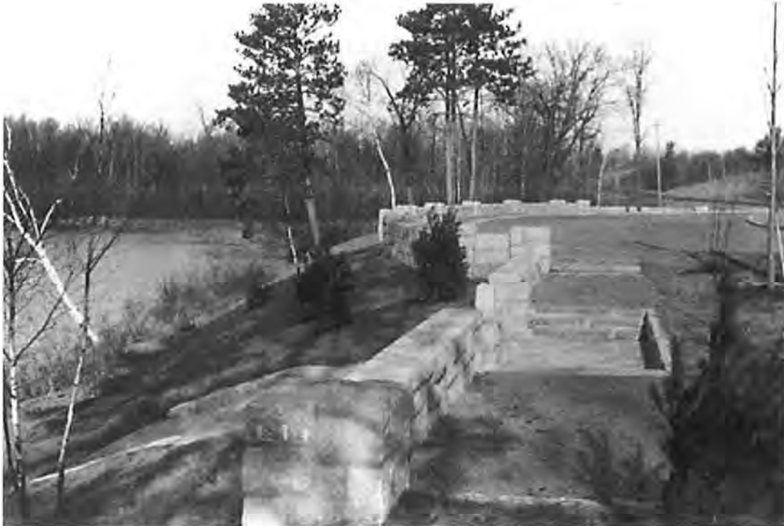
Figure 3. Kenney Lake Overlook nearing completion, probably taken in November 1939. In the photo the walkway and parking area appear to be surfaced with gravel, perhaps not yet covered with the tarvia treatment specified on the original plans, or the tarvia was never applied. The photo shows what appears to be an elm tree on the traffic island, as well as clumps of birches near the picnic area (center right), both specified on the original plans. The photo shows what appears to be a pine (lower right) where the plan specifies a spruce. The photo also shows some new trees and shrubs not drawn on the plans including several conifers (probably pines) on the lake side of the wall and a deciduous tree (probably an elm) near the new birches (center right). The clump of birches at lower left may also be newly planted (circa November 1939 photo by the Minnesota Dept. of Highways, A. R. Nichols photo album, Vol. 7, Site Development Unit, MnDOT, St. Paul).
