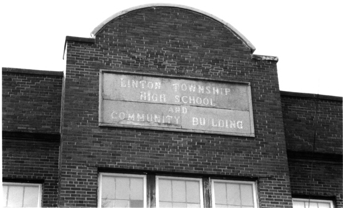
Linton Township High School and Community Building Vigo County, Indiana
