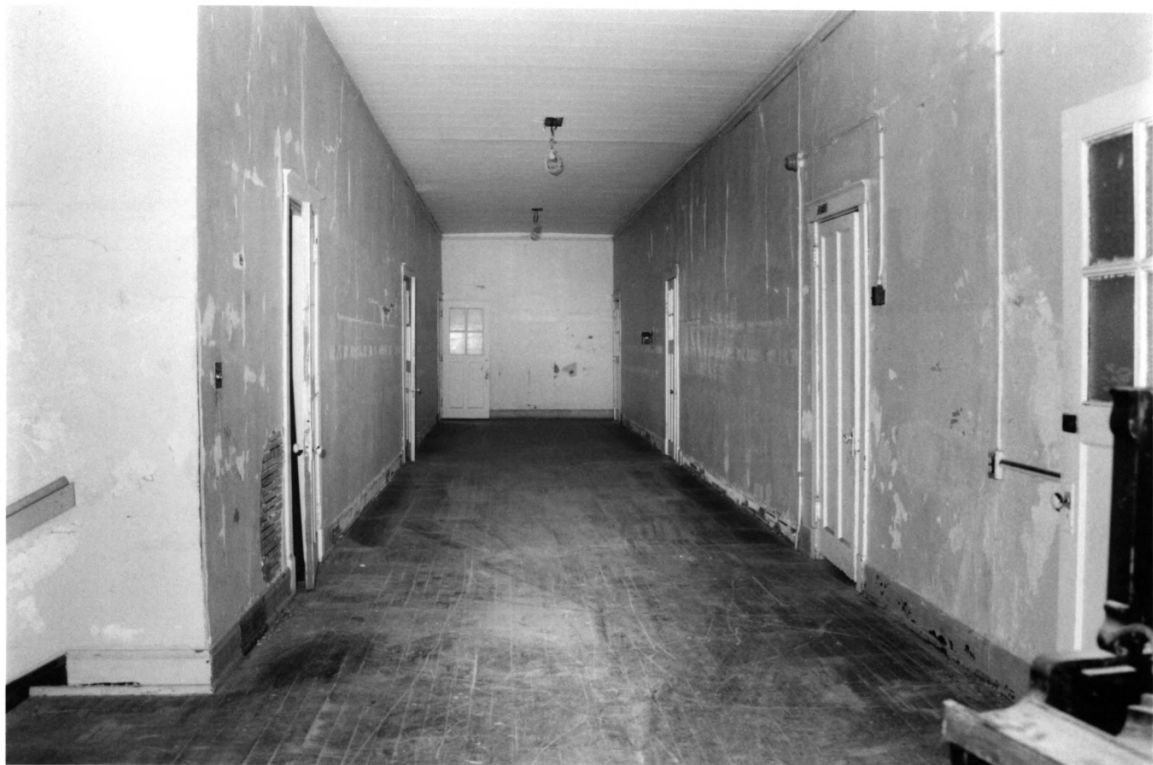
Linton Township High School and Community Building Vigo County, Indiana
