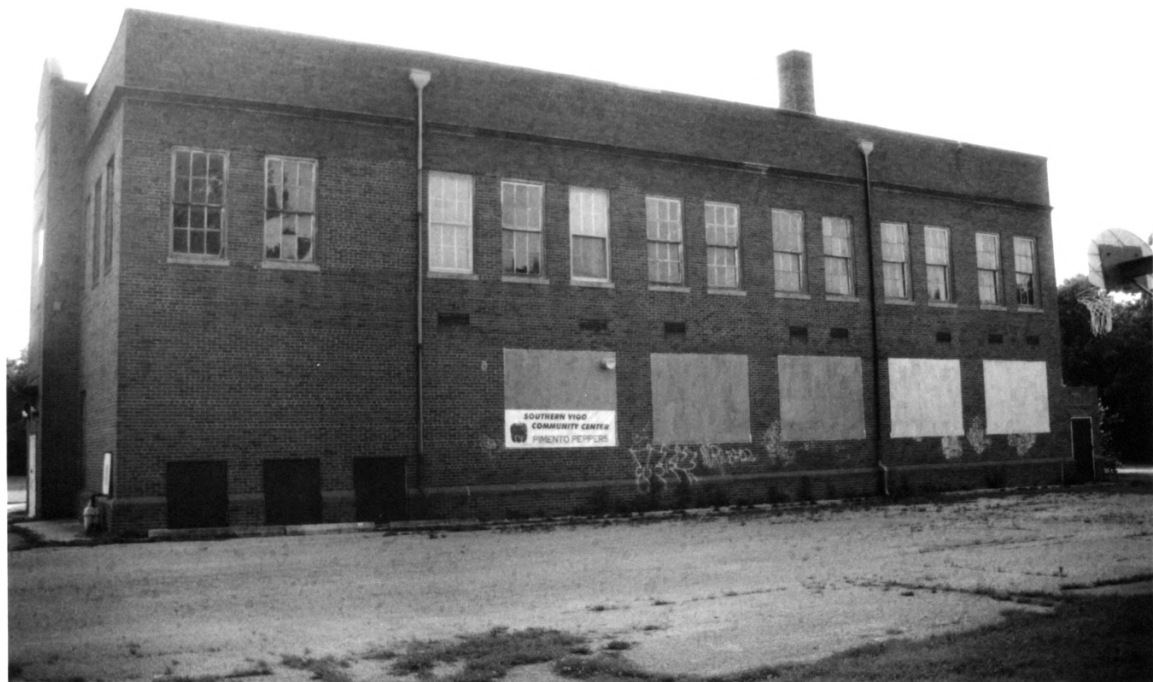
Linton Township High School and Community Building Vigo County, Indiana
