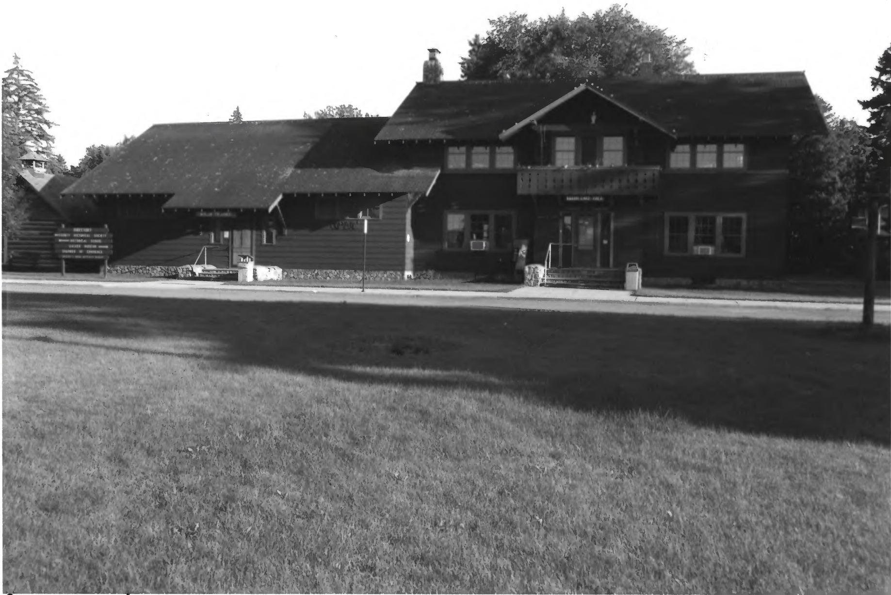
Conservation Building Cass Co., Mn 014391-18
