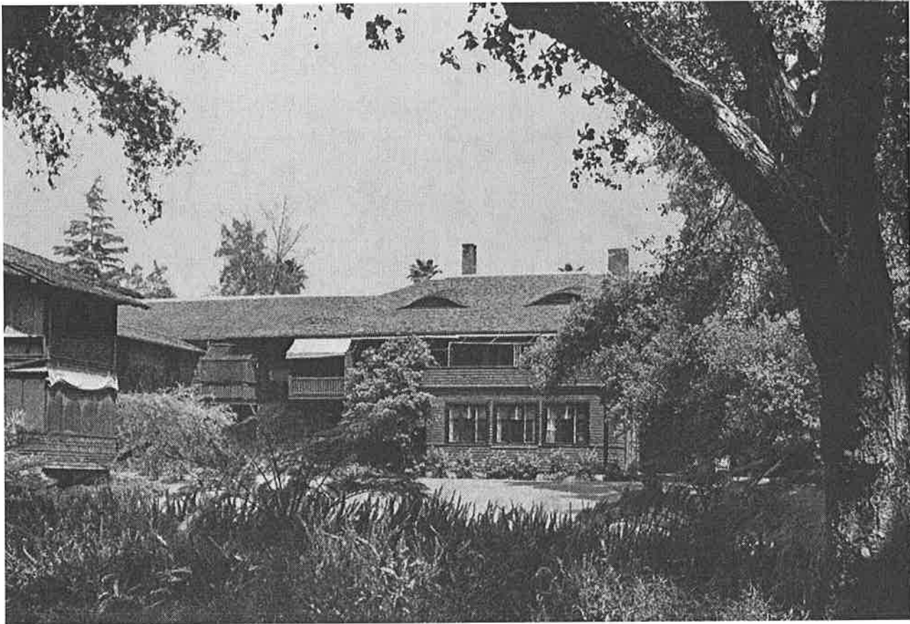
Figure 3. South elevation, with 1917 south wing addition on left, Southern California Sanitarium (date unknown). Source: Las Encinas Hospital.
