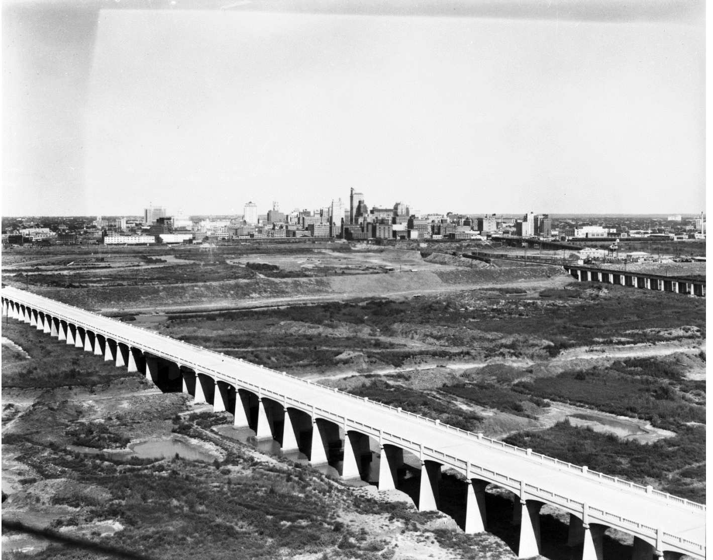
Lamar-McKinney Bridge (foreground) under construction, c.1930 Source: Dallas Public Library
