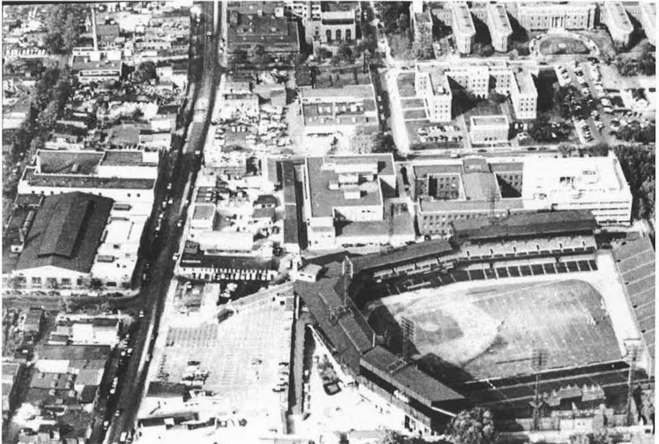
Aerial Image of Griffith Stadium showing WRECO Garage at center left in photo across from stadium
