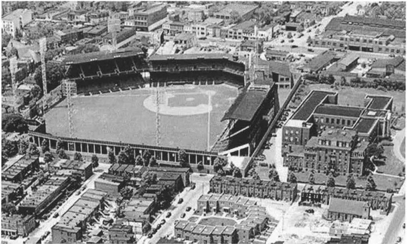
Aerial photo showing Griffith Stadium with WRECO Bus Garage in upper right hand corner of image, 1941
