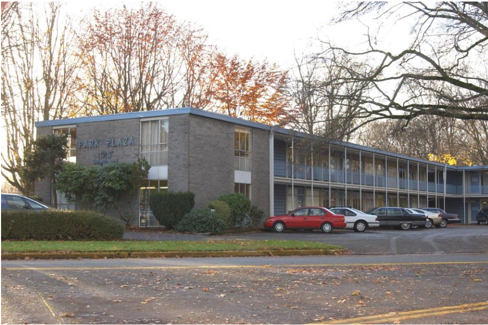
Figure 13. Park Plaza office building before remodel. Photograph by M. Houser, November 2006.
