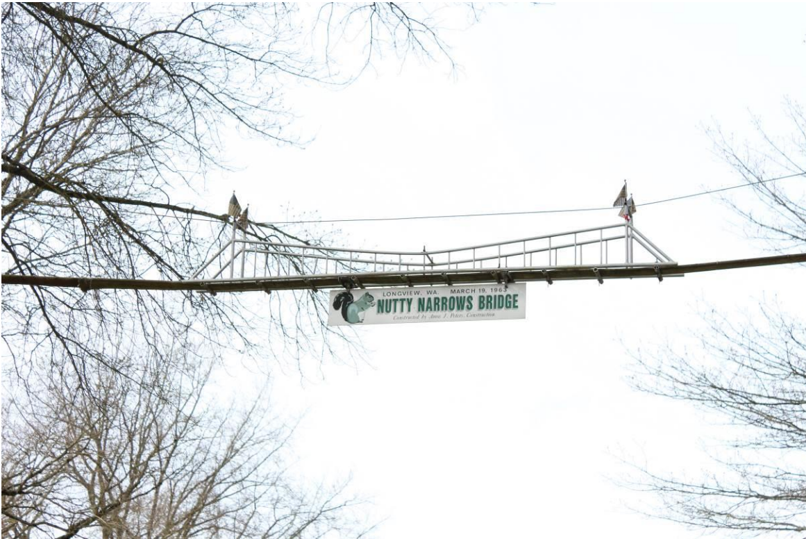
2 of 7: Looking northwest at Bridge
