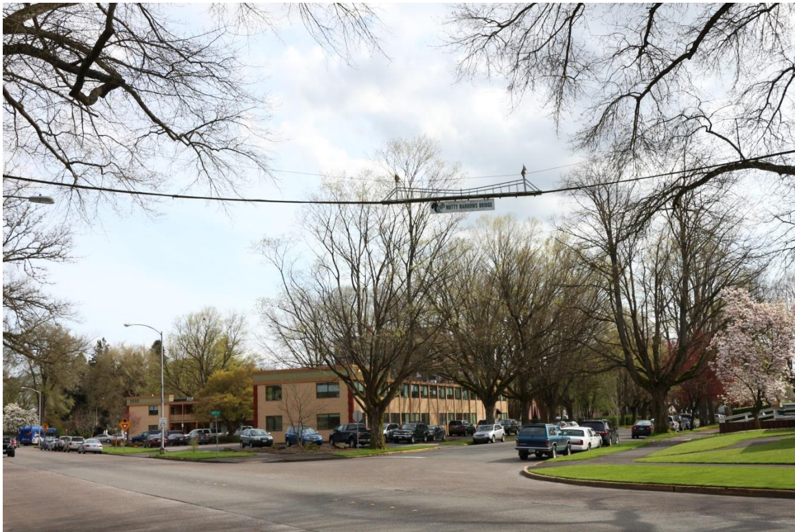
1 of 7: Looking south-southeast at Nutty Narrows Bridge and Park Plaza Building
