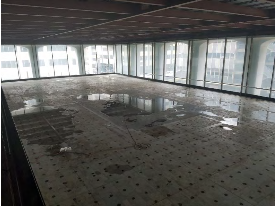
Photo 31 Original Bank lobby at level 4 – camera facing northeast from level 5
