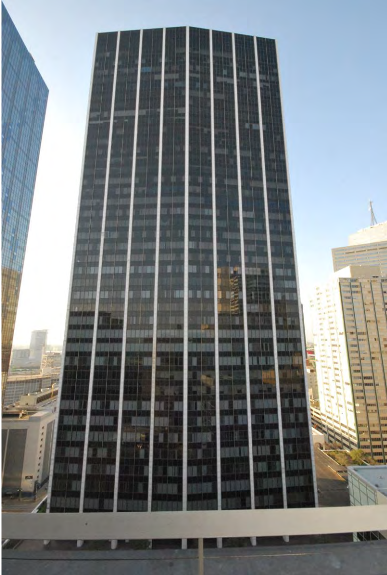
Photo 7 South tower elevation – camera facing north
