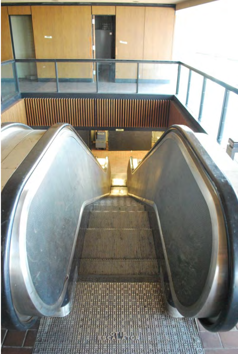
Photo 37 49 th /50 th floor escalators – camera facing east
