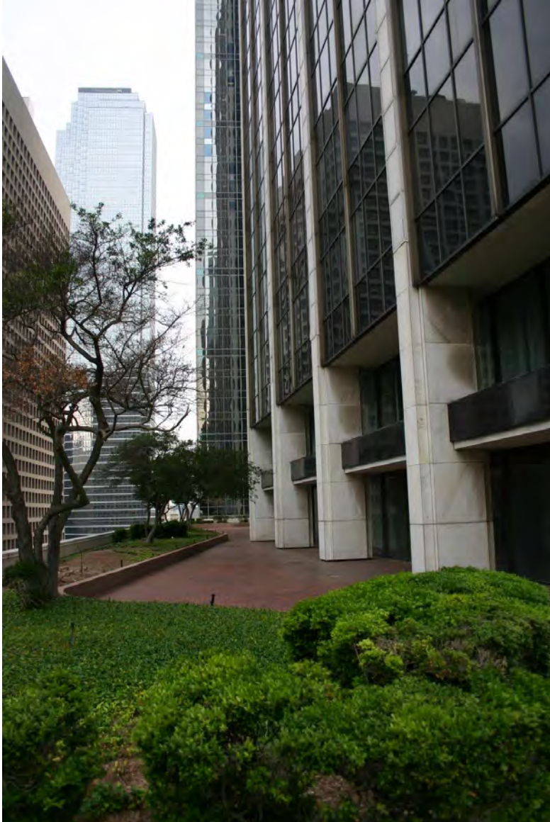
Photo 19 9 th floor terrace south elevation – camera facing west
