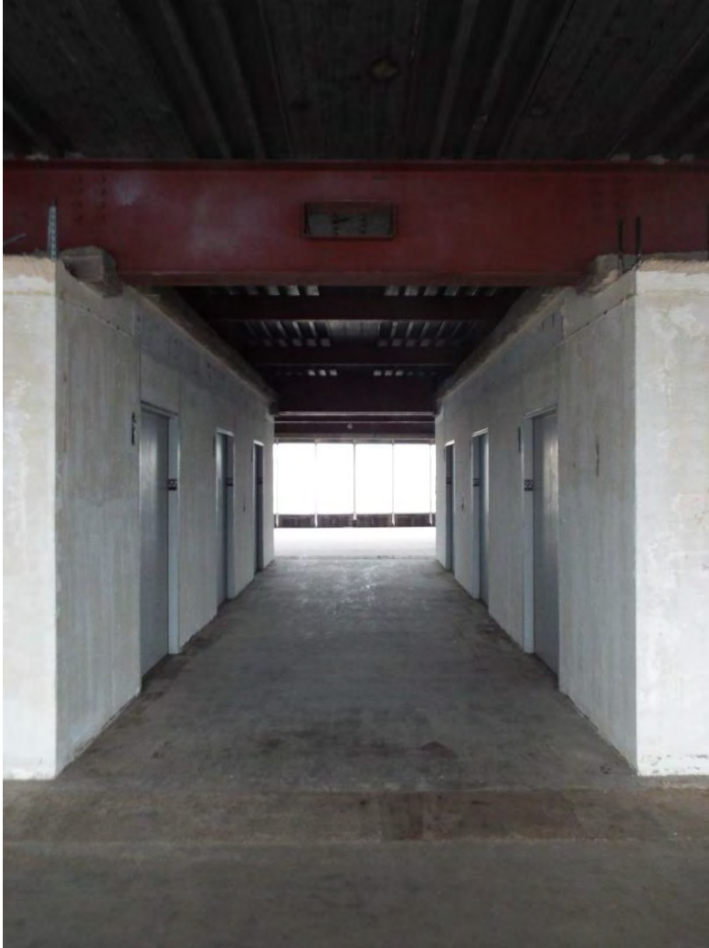
Photo 32 Typical tower elevator lobby
