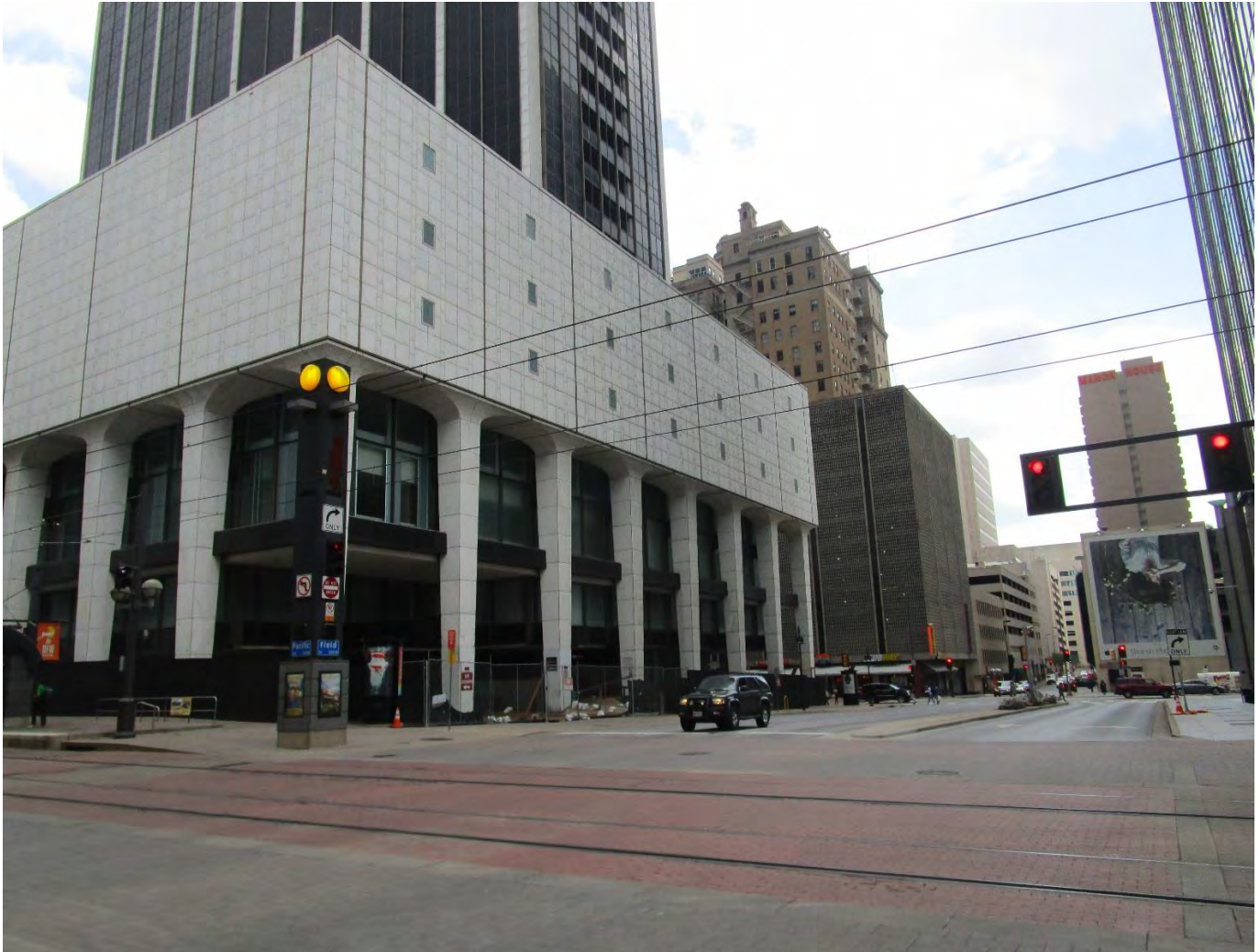
Photo 6 Northwest corner – camera facing southeast
