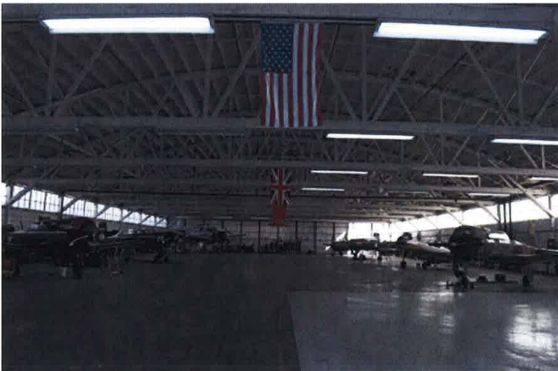
Photograph 10. West Hangar, interior
