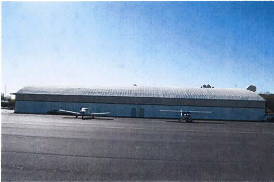
Photograph 3. East Hangar, north facade
