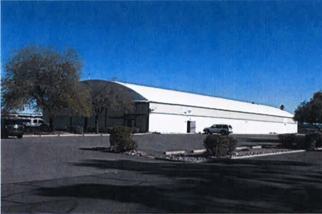
Photograph 5. East Hangar, west and south facades
