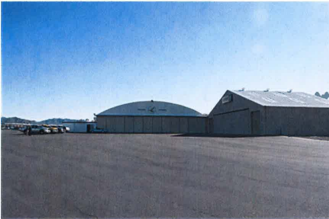
Photograph 7. West Hangar, west facade
