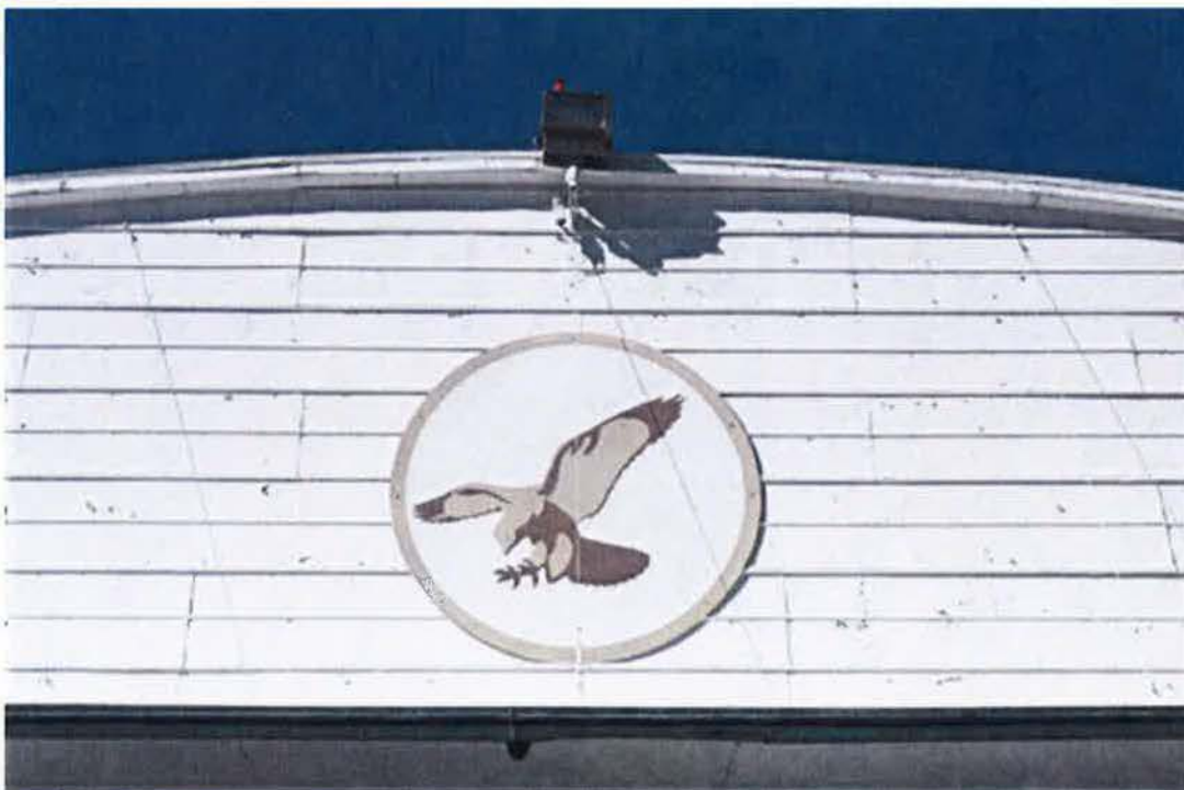
Photograph 2. East Hangar, east façade, detail
