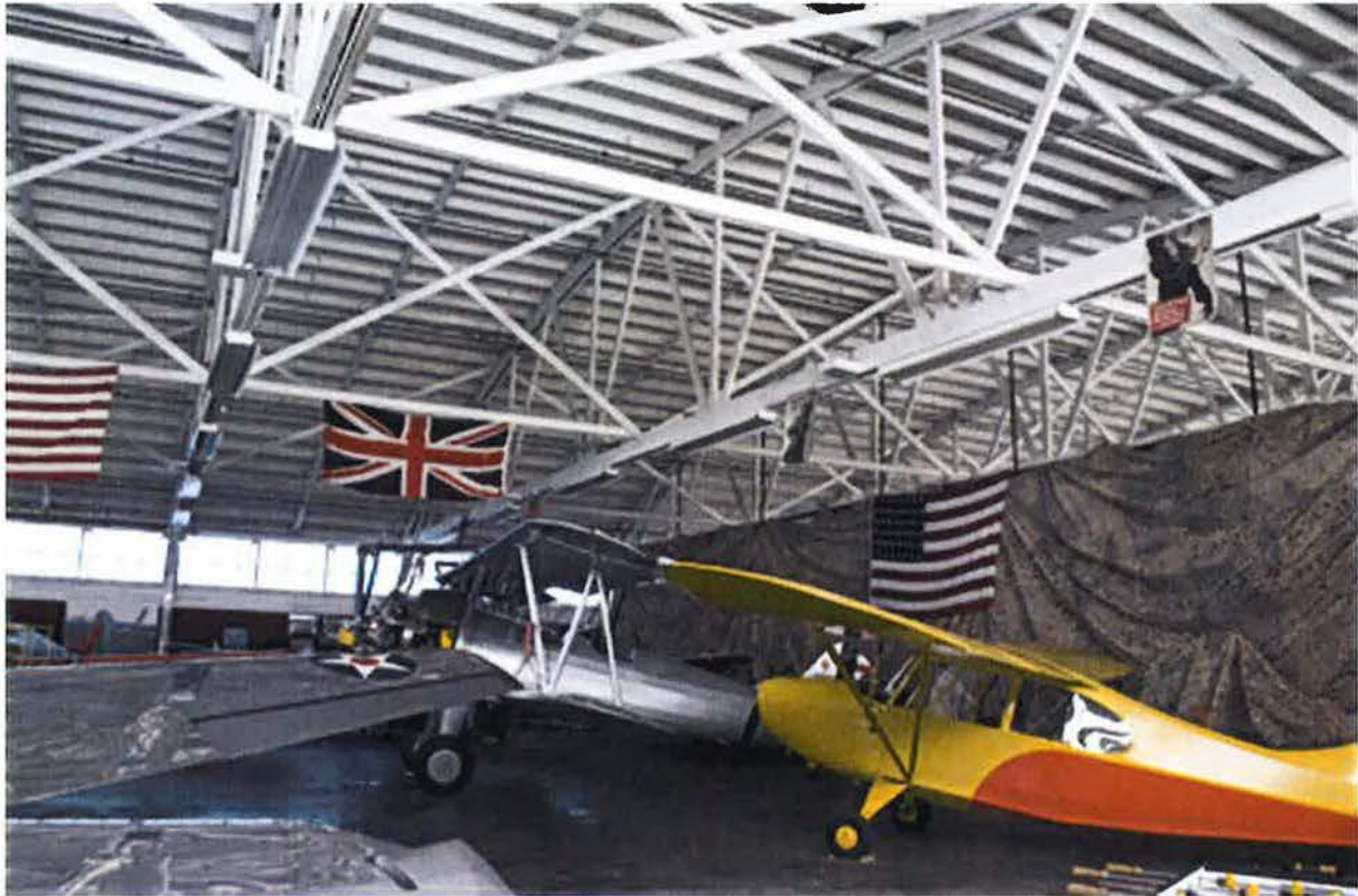
Figure 6. Interior view of East Hangar showing the integrity of the building's primary features, including its bow string trusses, barrel vault and window placement. Photo by Eric Vondy, State Historic Preservation Office, 2016.
