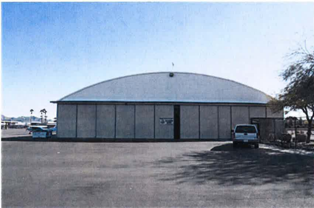
Photograph 4. East Hangar, west facade
