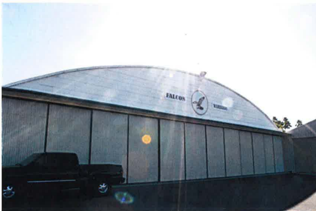
Photograph 8. West Hangar, west facade
