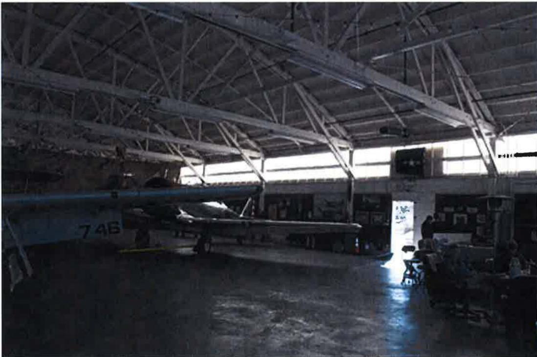
Photograph 6. East Hangar. Interior
