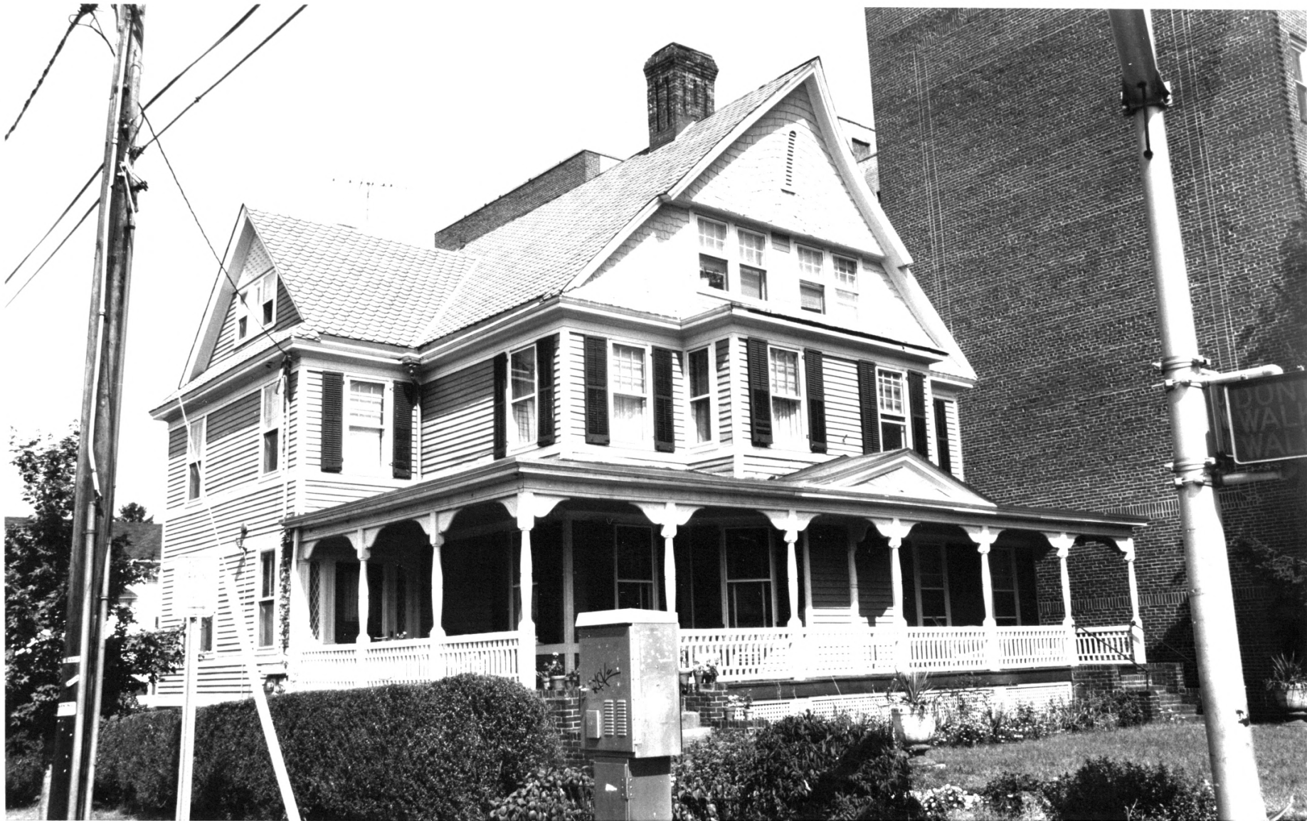
New Jersey Middlesex County Livingston Avenue Historic District Photograph 13 of 22
