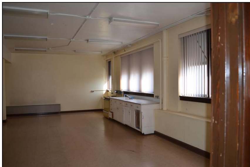
Photo #17 (WI_Eau Claire County_Eau Claire Vocational School_0017) Second floor room 203. Former dormitory area of vocational school.
