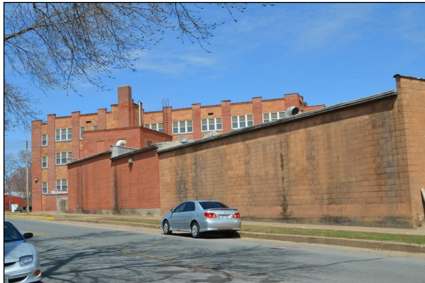
Photo #5 (WI_Eau Claire County_Eau Claire Vocational School_0005) West façade, camera facing northeast.
