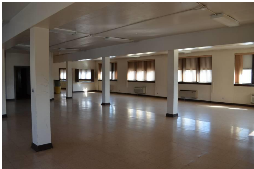
Photo #16 (WI_Eau Claire County_Eau Claire Vocational School_0016) Second floor room 204. Former dining hall and lounge area of vocational school.
