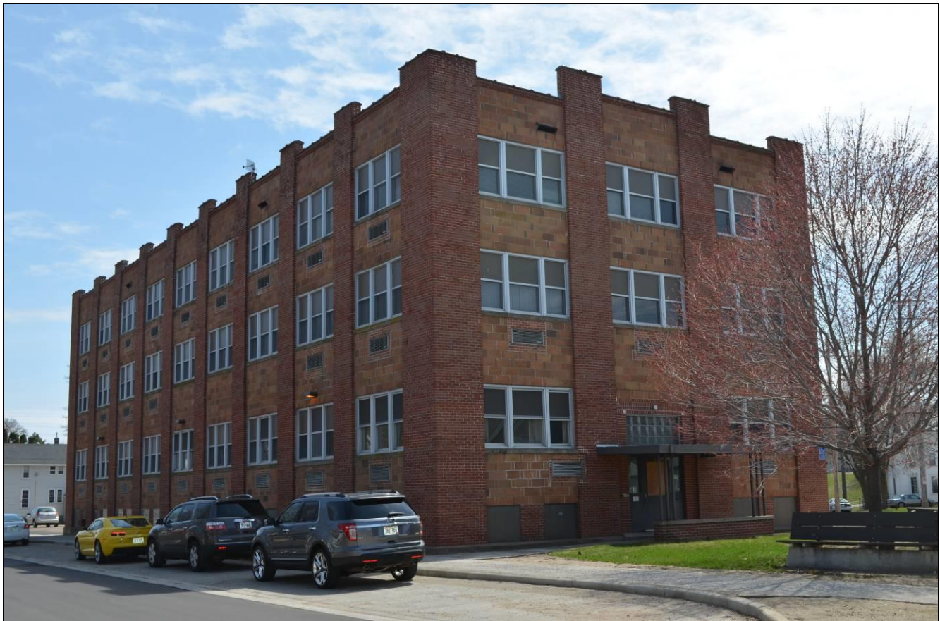
Photo #1 (WI_Eau Claire County_Eau Claire Vocational School_0001) North façade (right) and east elevation (left), camera facing southwest.
