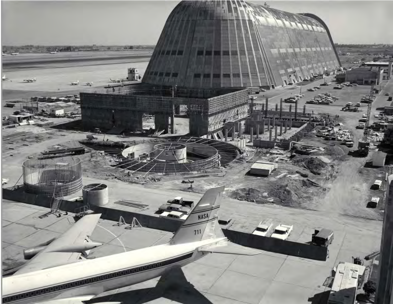
Figure 3. Building N-243 under construction, October 4, 1965
