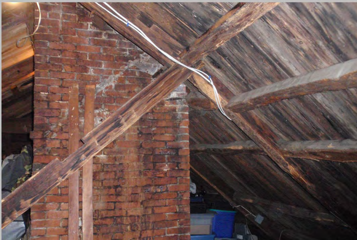
23. Attic, facing southeast
