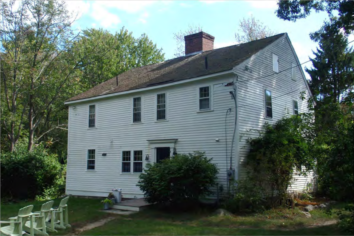
4. North (rear) and west (side) elevations, facing southeast
