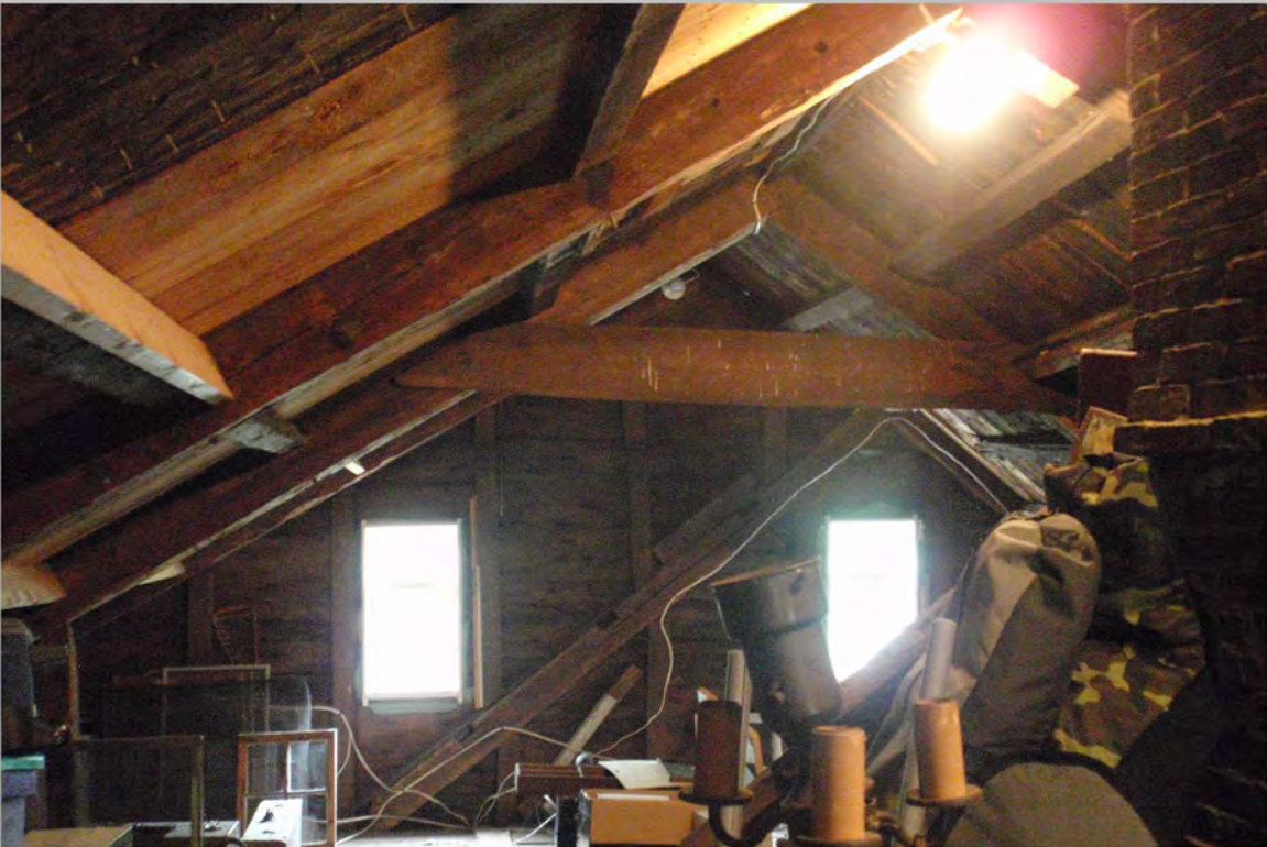
21. Attic, facing east
