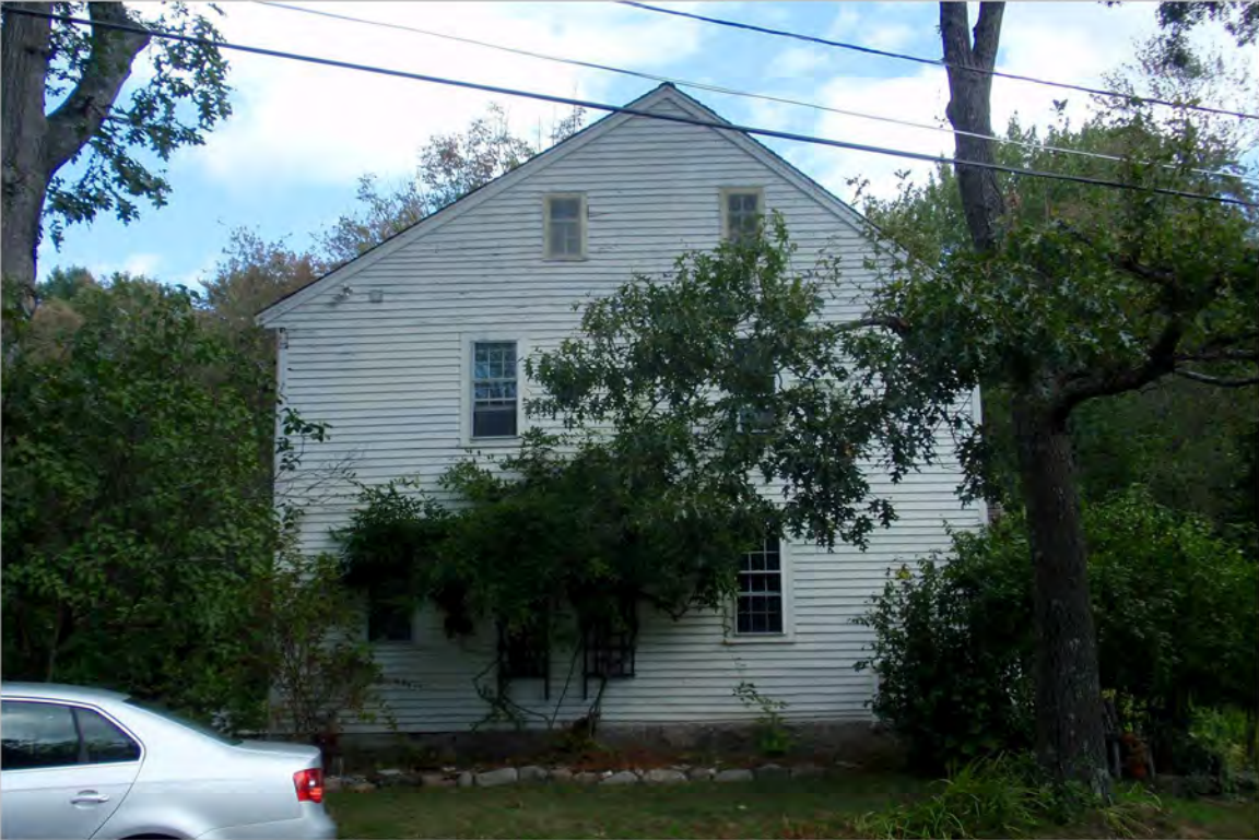
3. West elevation, facing east
