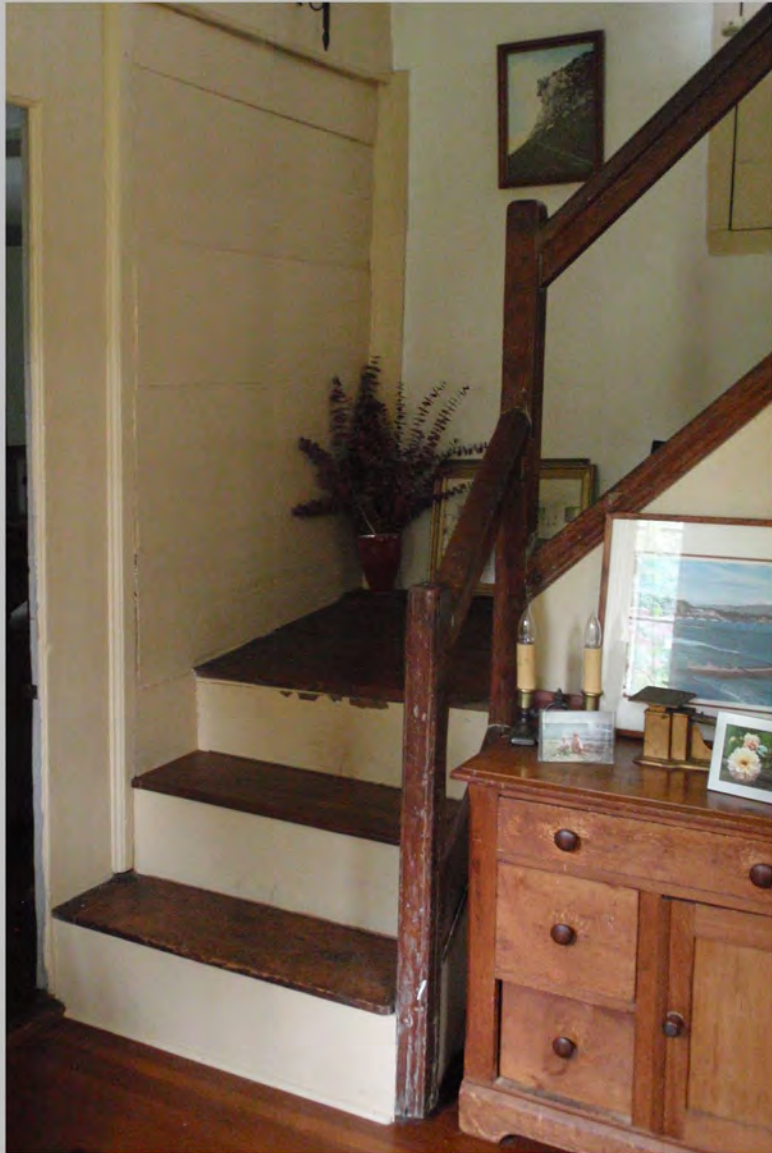
9. Main stairs, facing northwest
