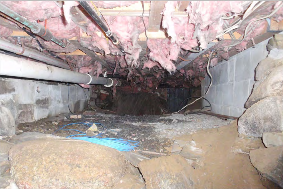
8. Basement, chimney stack to the right, facing east
