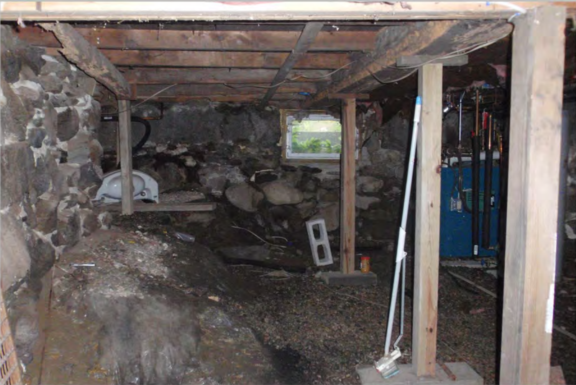
7. Basement, chimney stack to the left facing south
