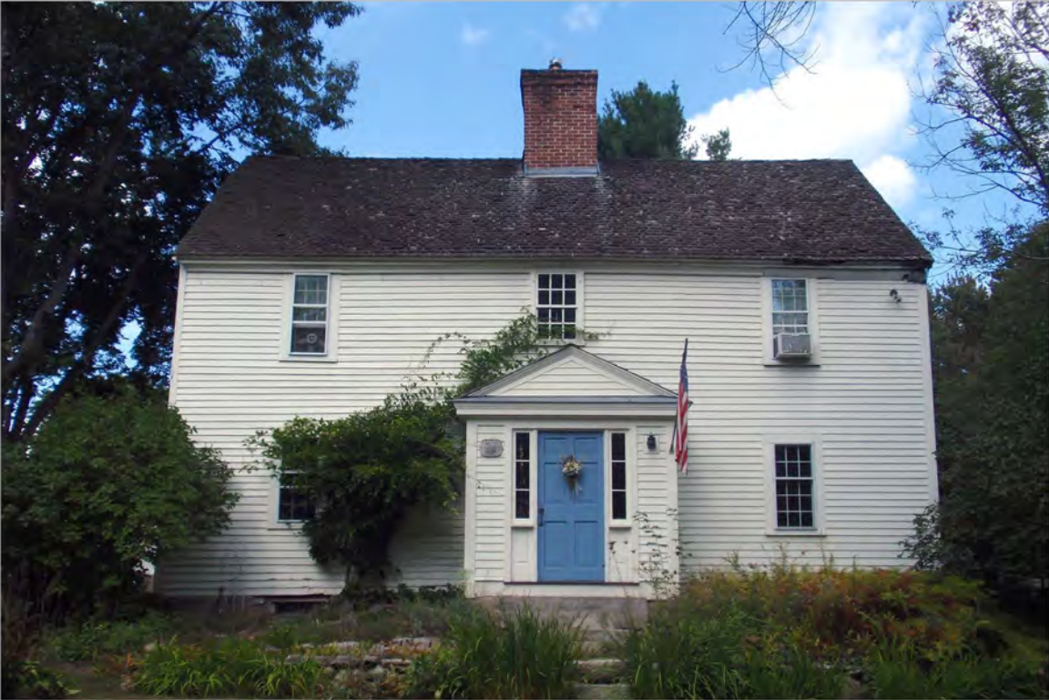
1. South (façade) elevation, facing north
