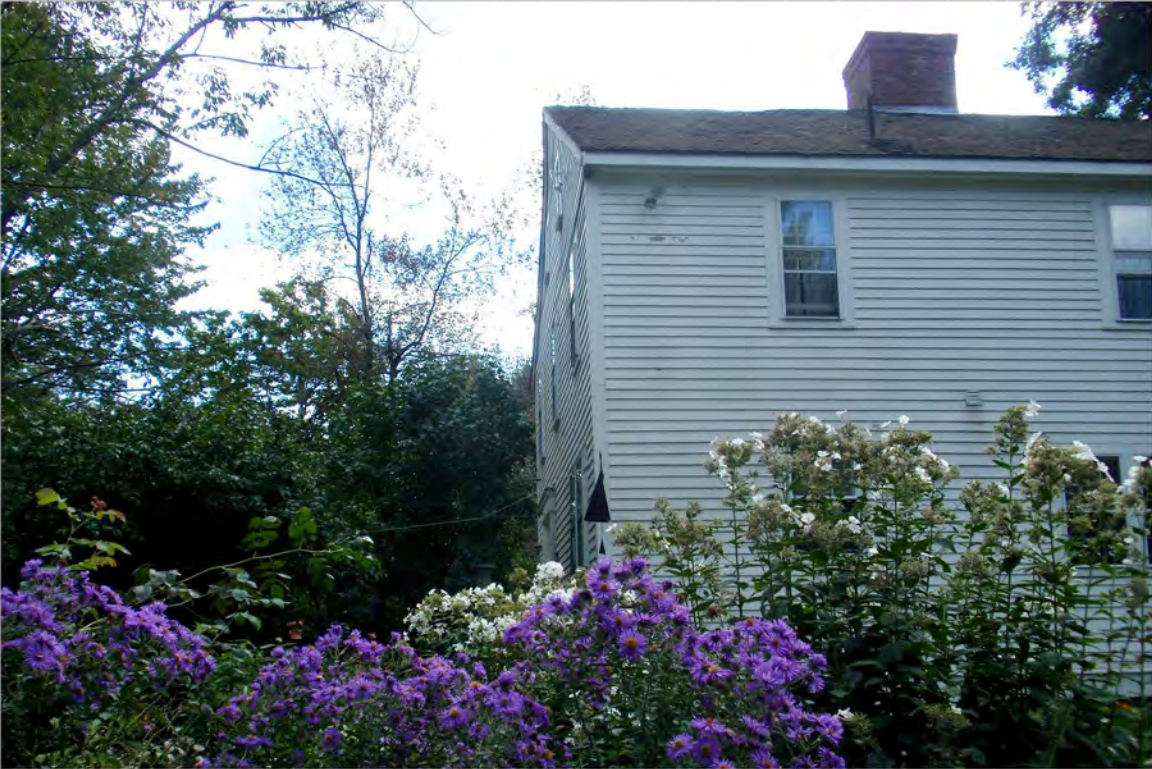
5. North (rear) and east (side) elevations, facing south
