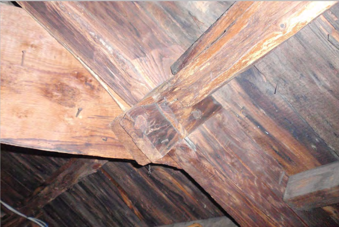
22. Attic, facing southeast
