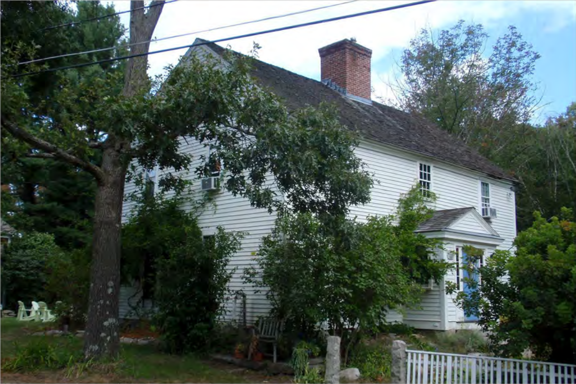
2. South (façade) and west (side) elevations, facing northeast
