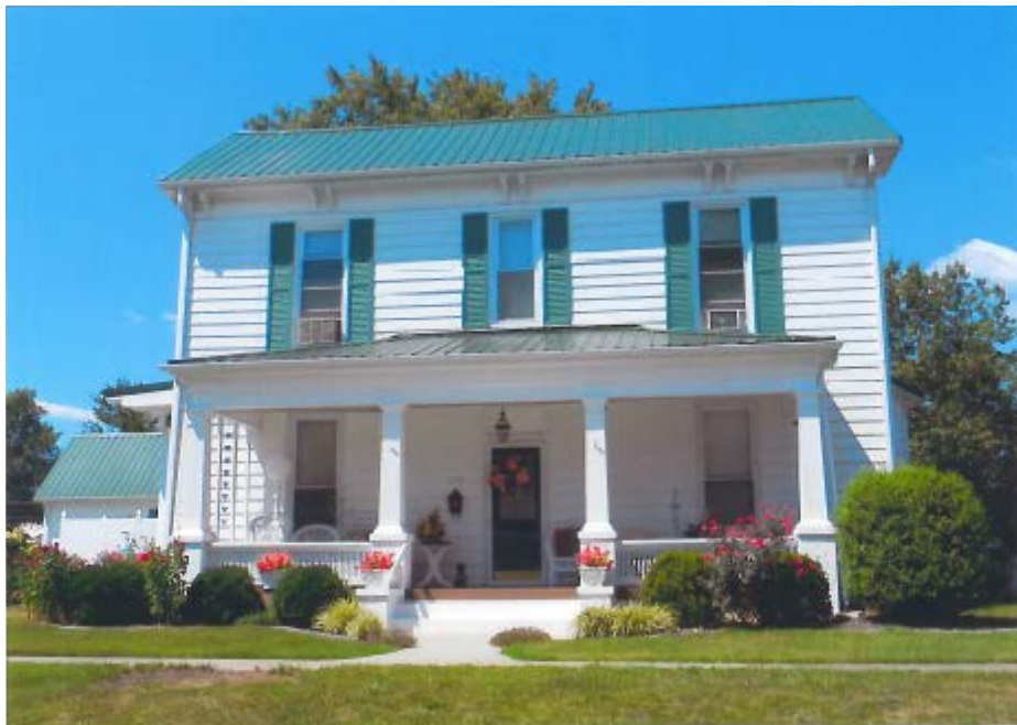
Figure 15: Survey Update Photo of 309 Third, Fairfield, IL, 2017
