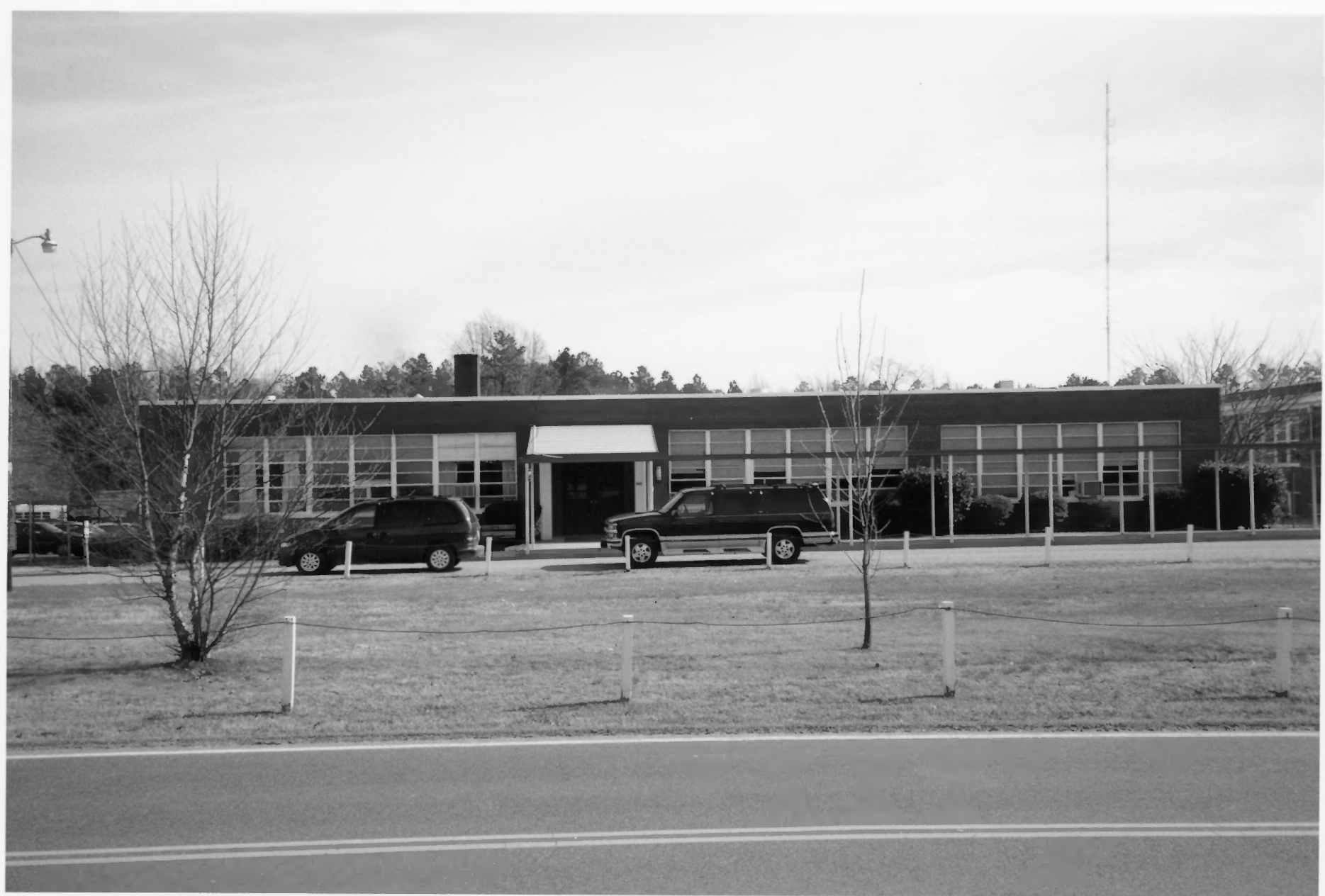
Figure 3. New Kent School 1954 Building, Front Elevation
