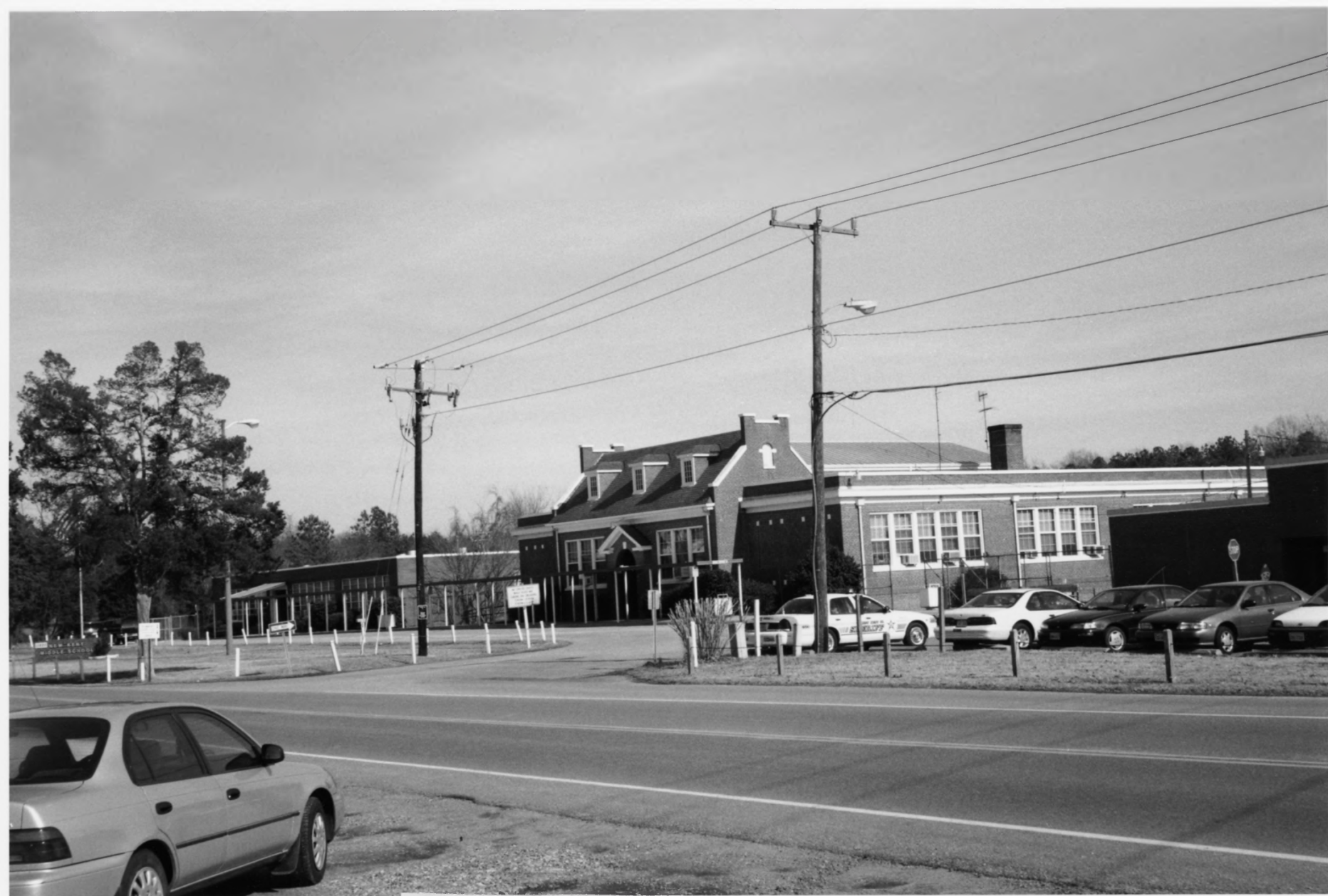
Figure 1. New Kent School Front and West Elevations
