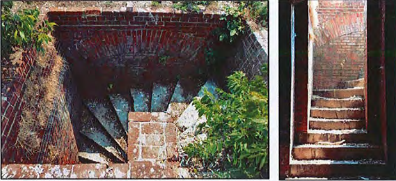
Stairwells: (spiral typical on both ends of Front 4)
