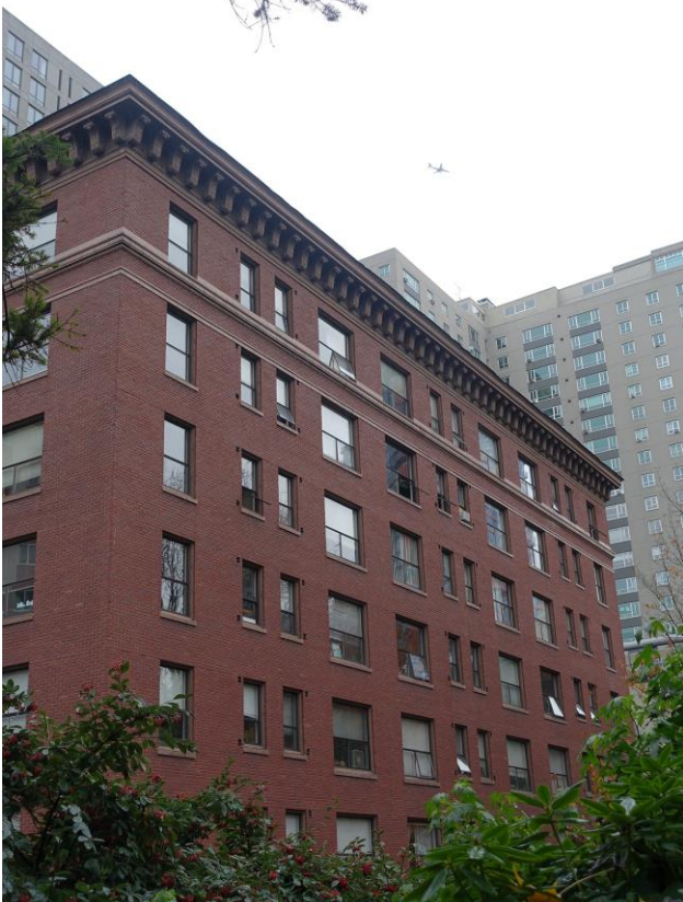
0005. General site view and context, west elevation looking southeast.
