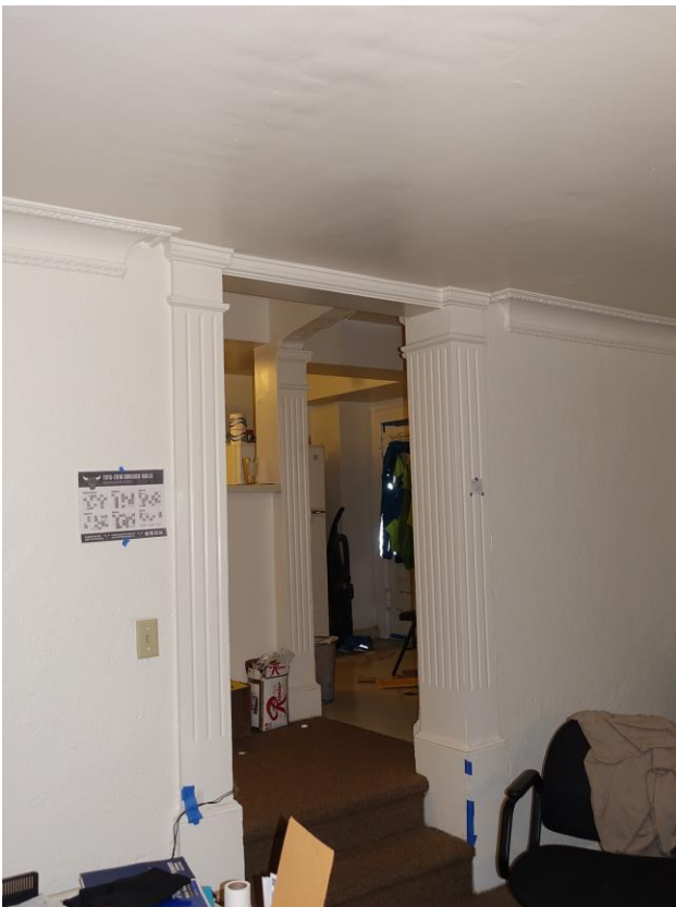
0027. Interior, view of Manager's unit (former Tea Room).
