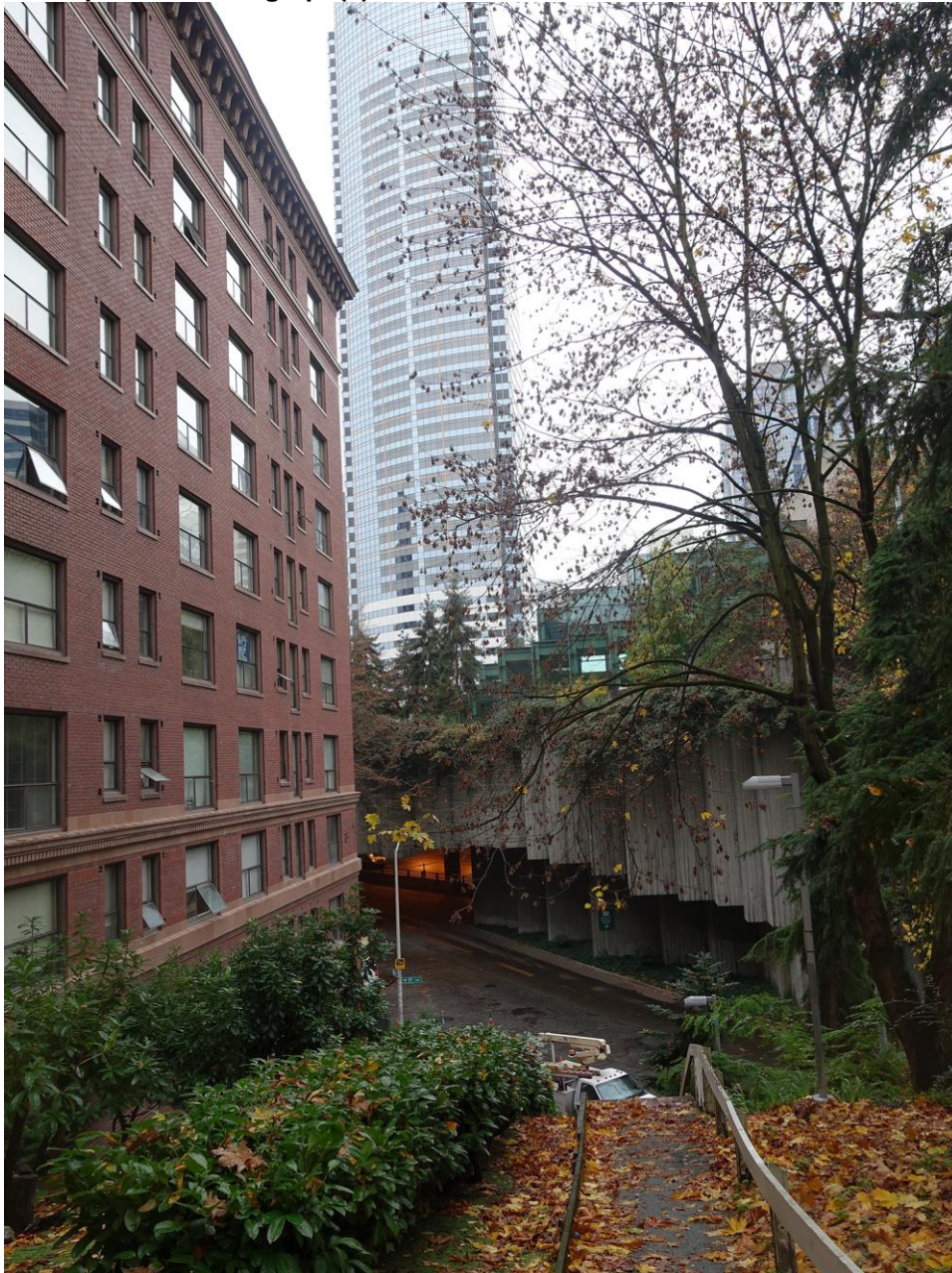
01. General site view and context, north elevation, looking west on Union Street stairs
