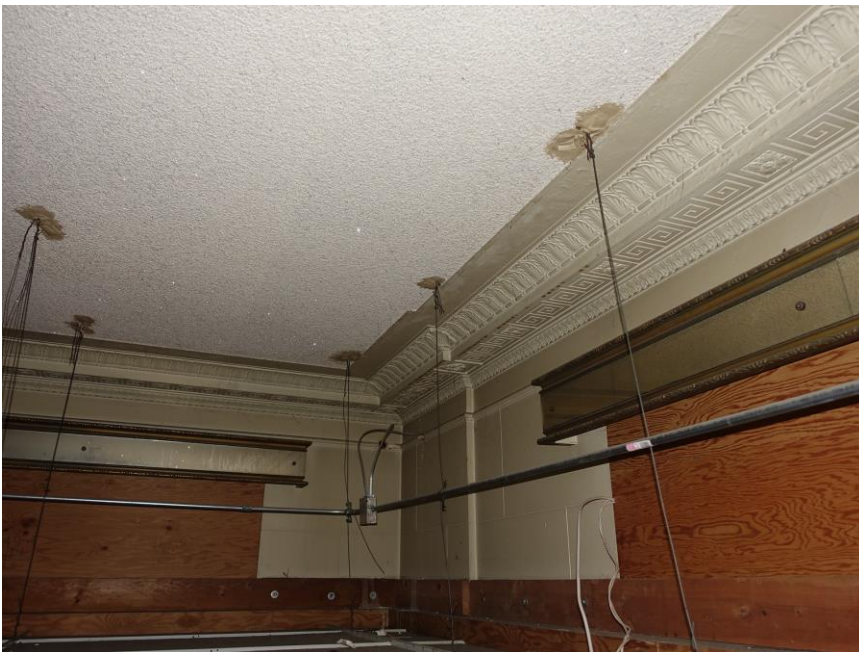
0017. Interior, Lobby ceiling view (in Office, above acoustic ceiling).
