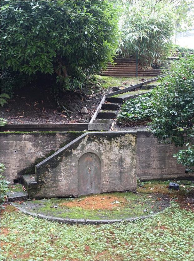
0006. Courtyard view, looking southeast.
