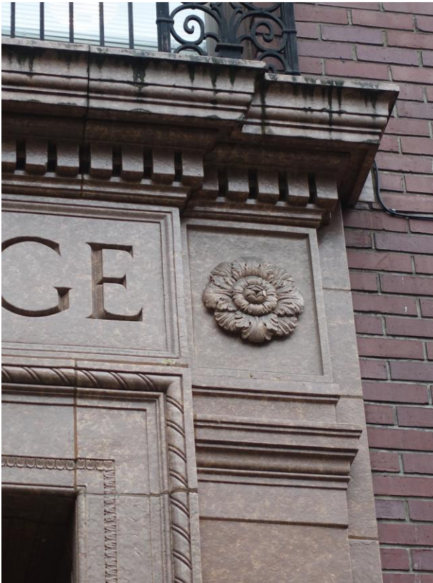
0010. Detail view of primary entry terra cotta surround & rosette, north elevation.
