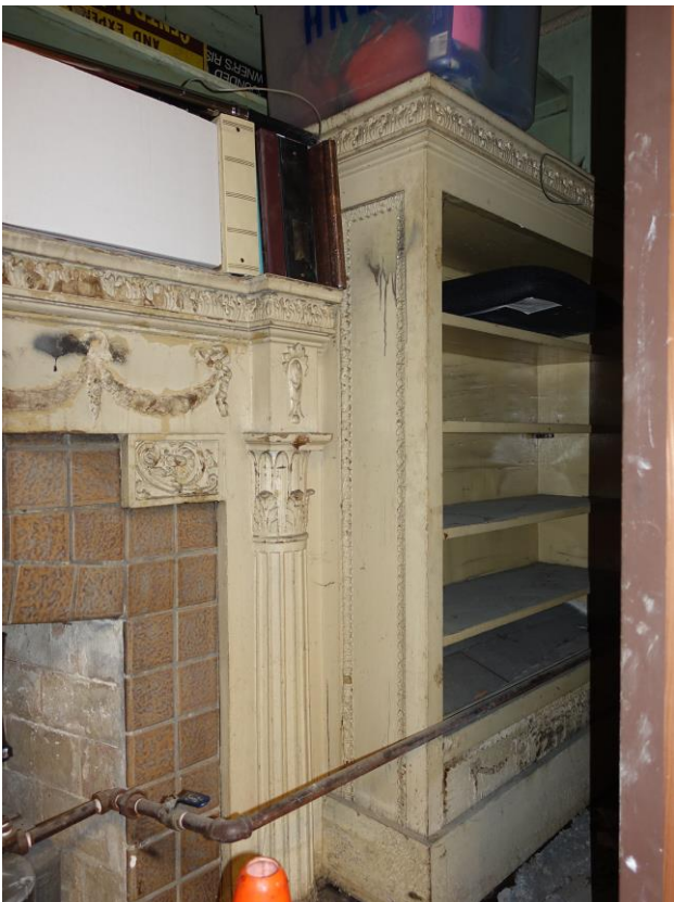
0019. Interior, view of Radio Room fireplace & cabinets (in office closet).
