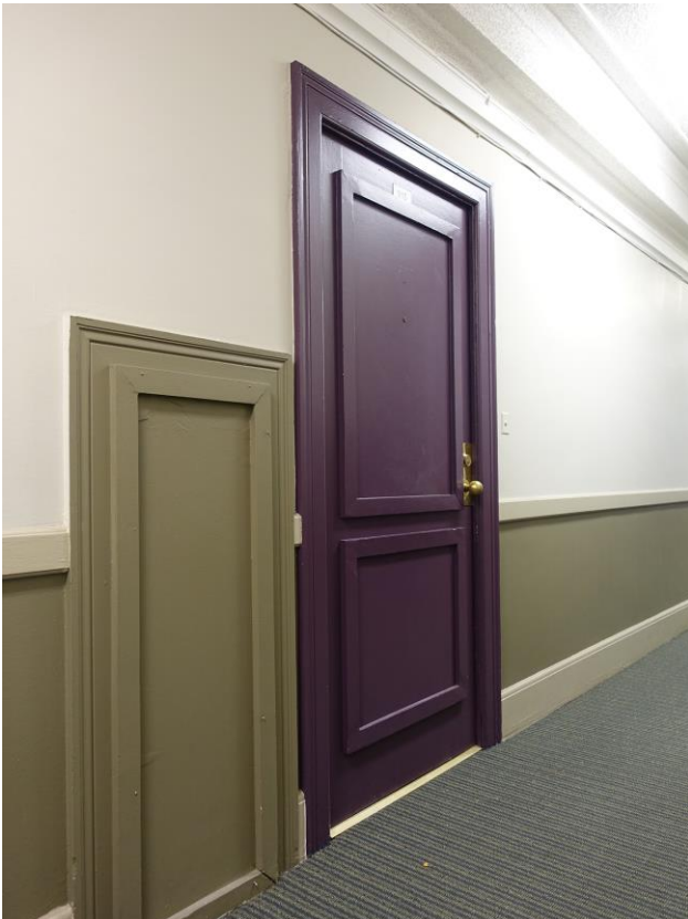
0023. Interior, detail view of unit door & delivery cabinet, typical residential Corridor.
