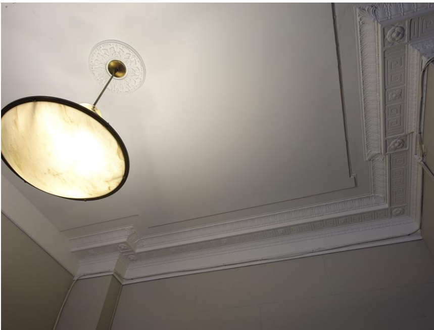
0015. Interior, detail view of ceiling at building lobby.
