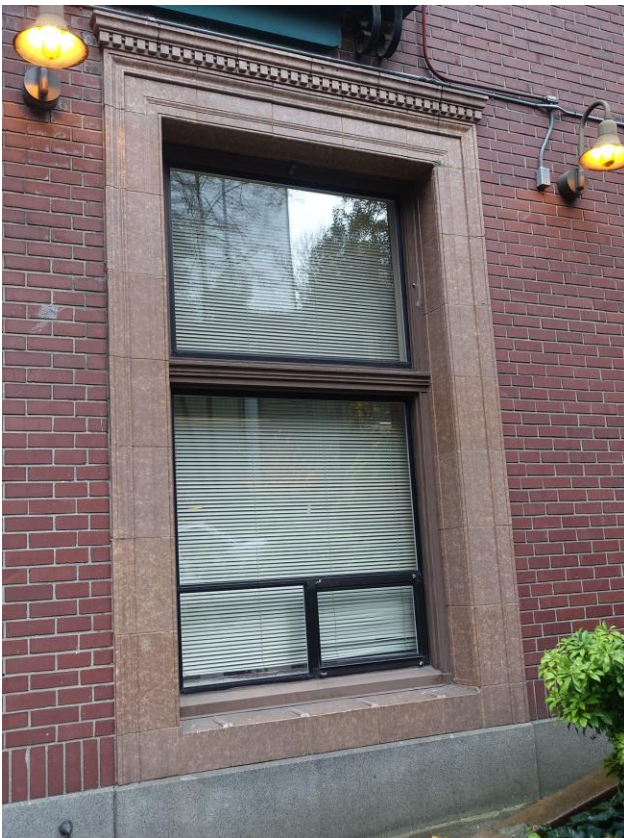
0009. Detail view of first floor window terra cotta surround, north elevation.
