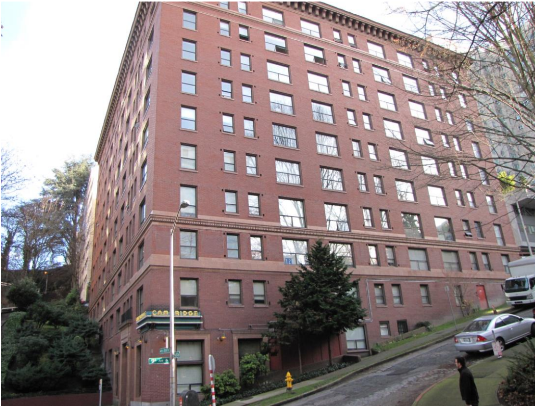
0004. General site view and context, northwest corner from across street looking east.
