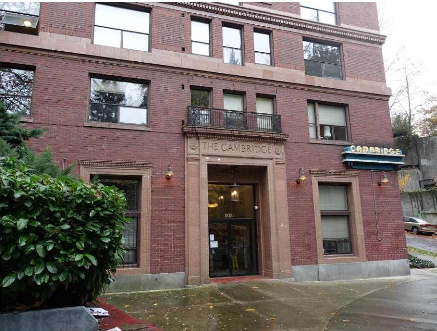
0007. Primary entry, north elevation looking south.
