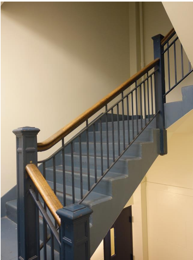
0021. Interior, typical flight of stairs, central stair.
