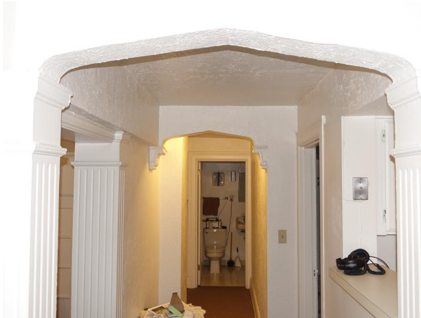
0028. Interior, view of Manager's unit & kitchen (former Tea Room).
