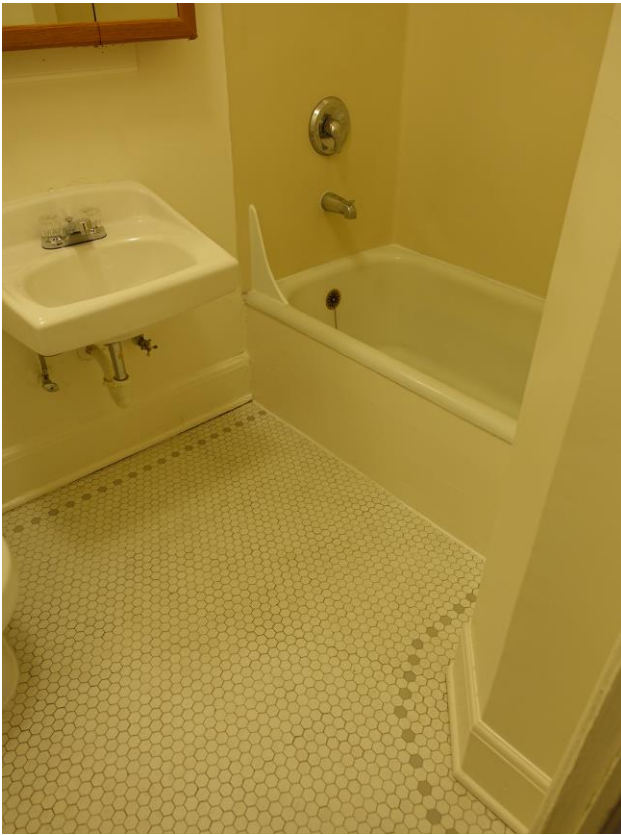
0026. Interior, typical residential bath & tile floor.
