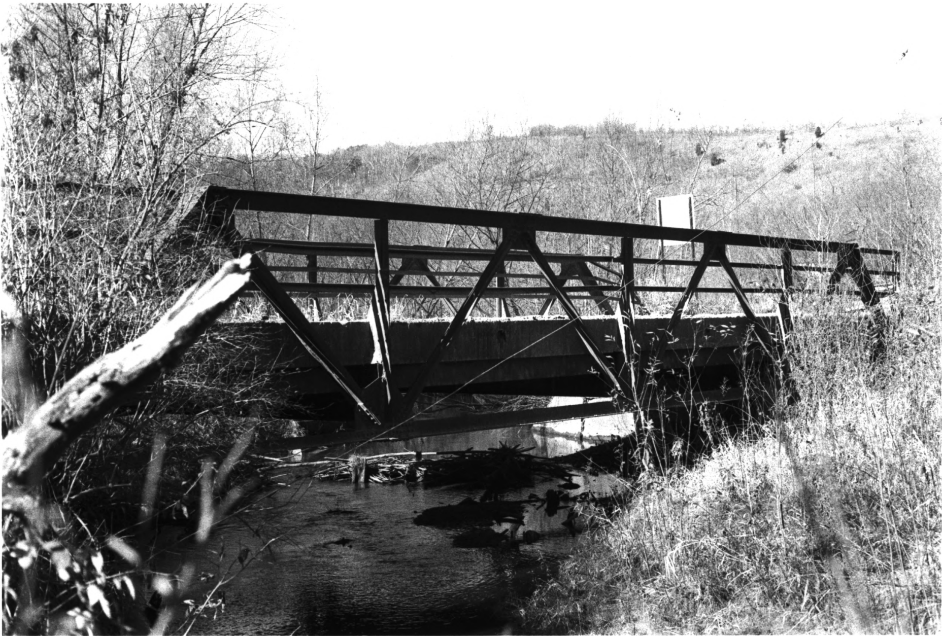
BRIDGE No. 12 GOODHUE CO., MN PHOTO I.D. 09140 #19
