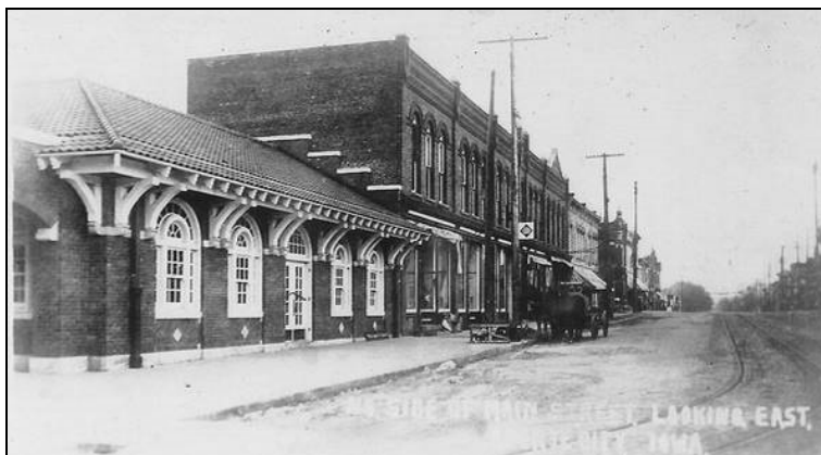
Post 1912 photograph of the WCF&N La Porte City Depot at left. Copy obtained from flickrriver.com , 2017.
