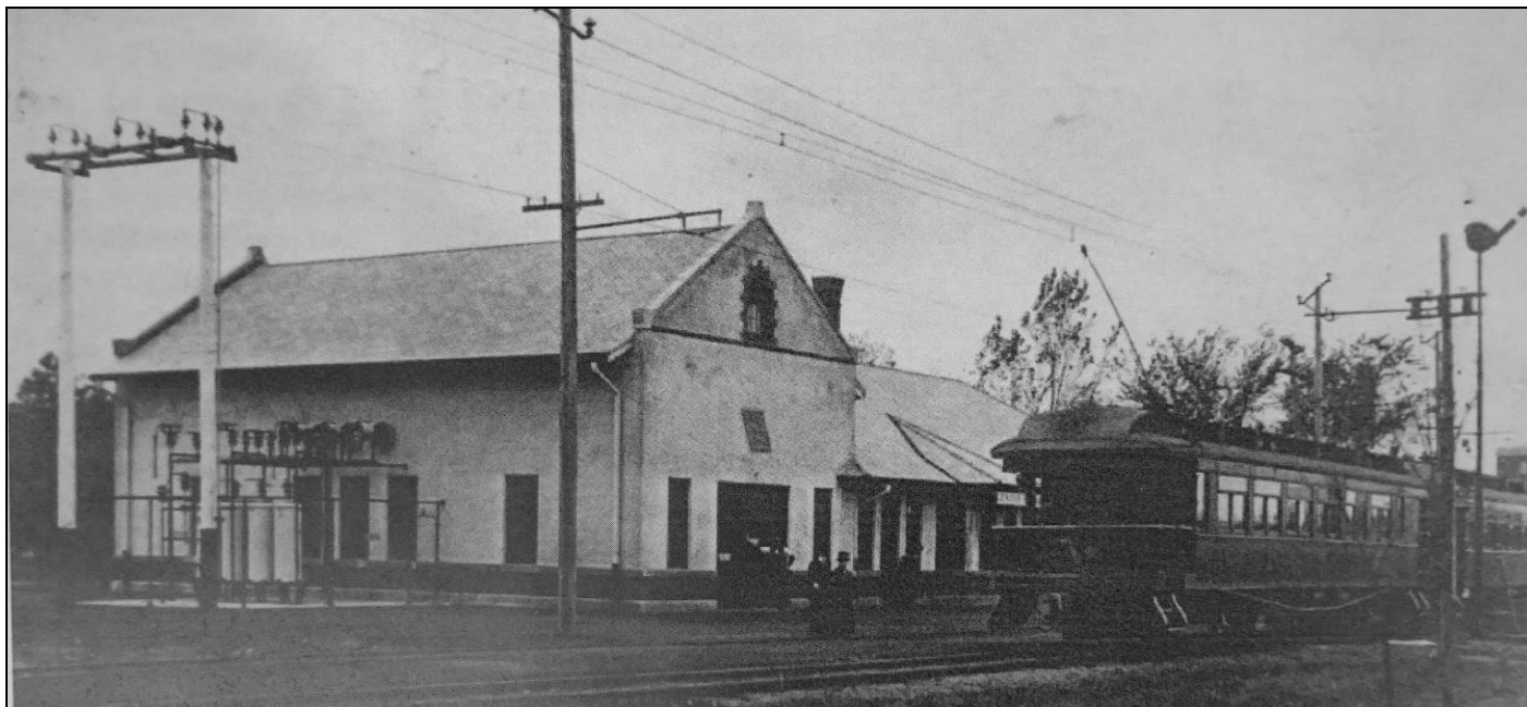
Undated photograph of the WCF&N Center Point Depot looking NW and showing the electrical lines and transfer superstructure off the south wall of the substation.
