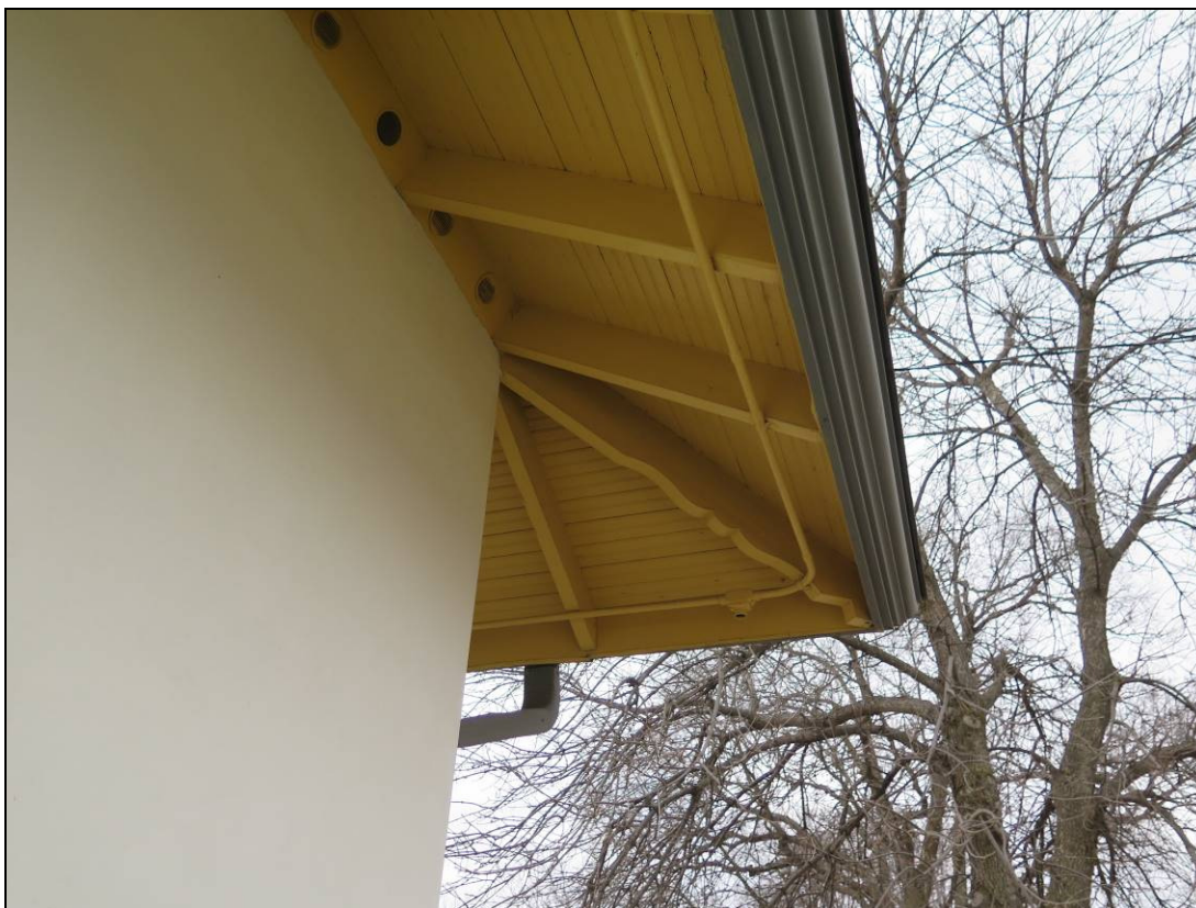
Detail of beaded-board soffit, plain, shaped exposed rafter ends, and ventilation holes in frieze board at the NW corner of the Center Point Depot building. Photograph taken by Leah Rogers, December 31, 2016.
