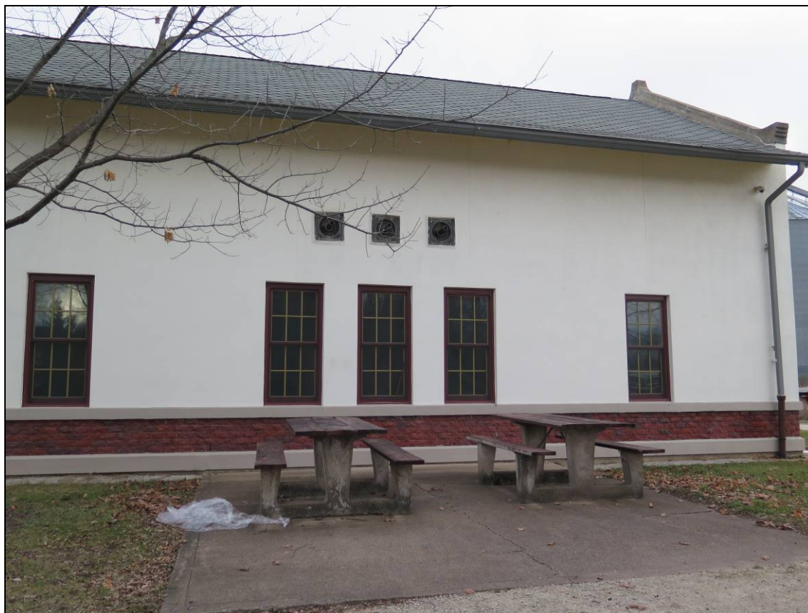
Photograph of the south side of the Center Point Depot showing the concrete pad (in foreground with two picnic tables on top) where the electrical transfer superstructure once stood next to the substation.
