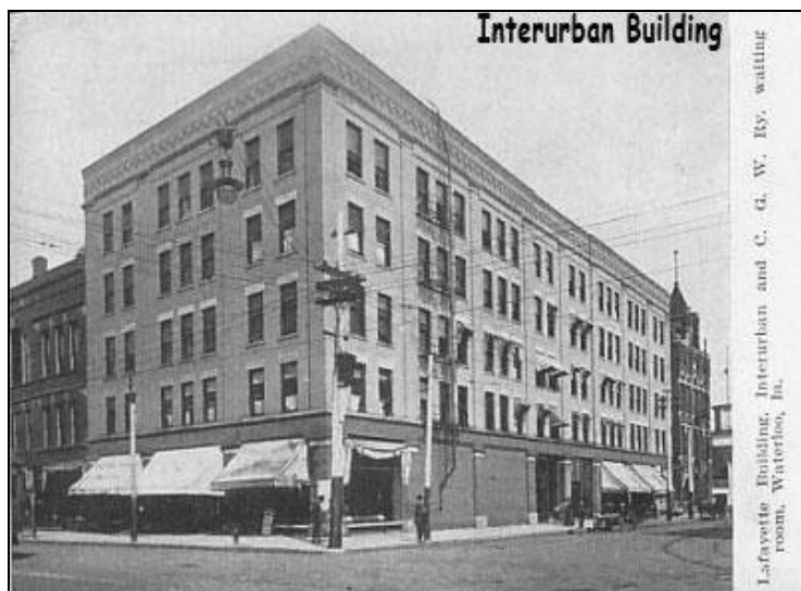
Lafayette Building “Interurban and C.G.W. Ry. waiting room, Waterloo, Ia” [non-extant]
