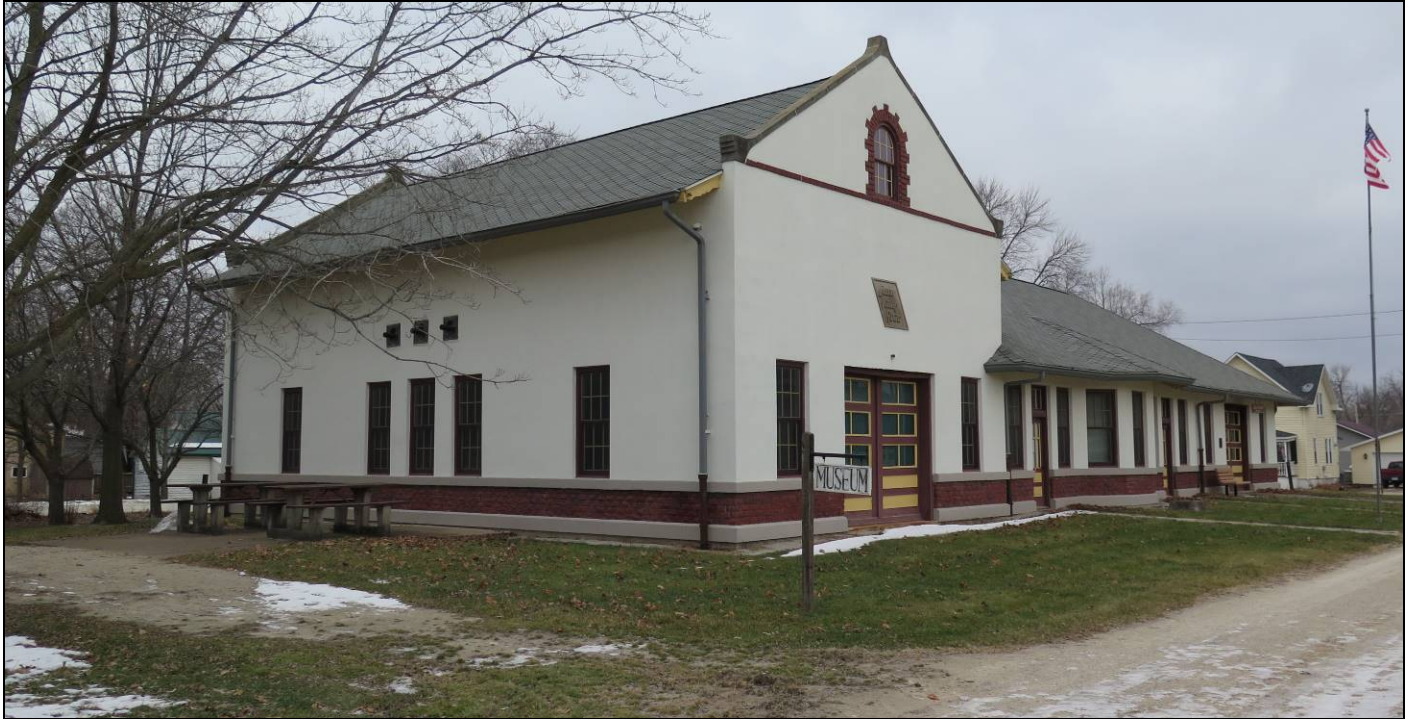
WCF&N Center Point Depot and Substation looking NW. Photograph taken by Leah Rogers, December 31, 2016.
