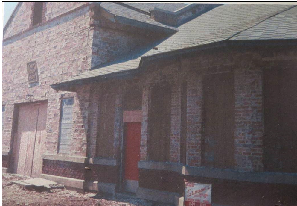
Photograph from the 1980s rehabilitation showing the stucco removed from the exterior of the Center Point Depot. Photograph on file Center Point Depot Museum collections, Center Point Historical Society, Center Point, Iowa.
