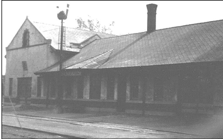
WCF&N Center Point Depot, Center Point in 1952. Photo obtained from Digital.lib.uiowa.edu_railroadiana , 2017
