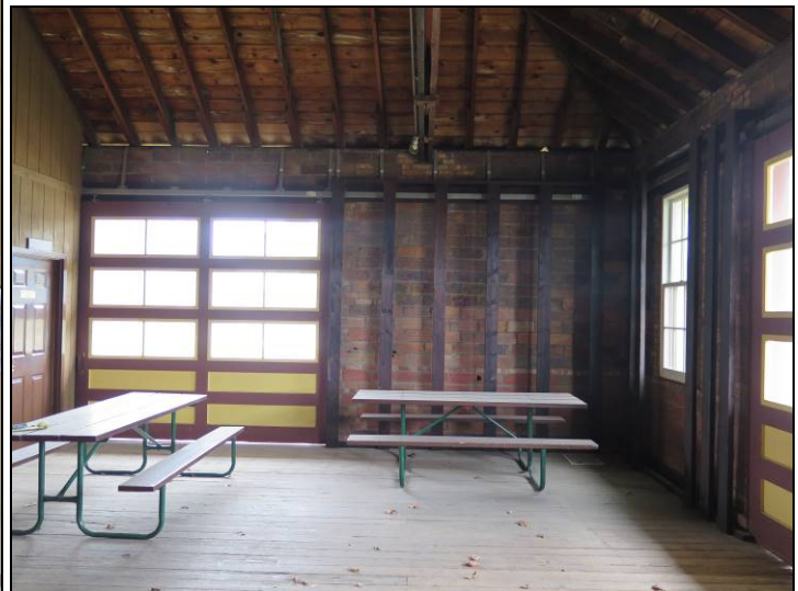
Interior of freight room looking SSE at tile block wall and roof truss and rafters. Interior of freight room looking NNW at sliding doors. Photographs taken by Leah Rogers, March 18, 2017.
