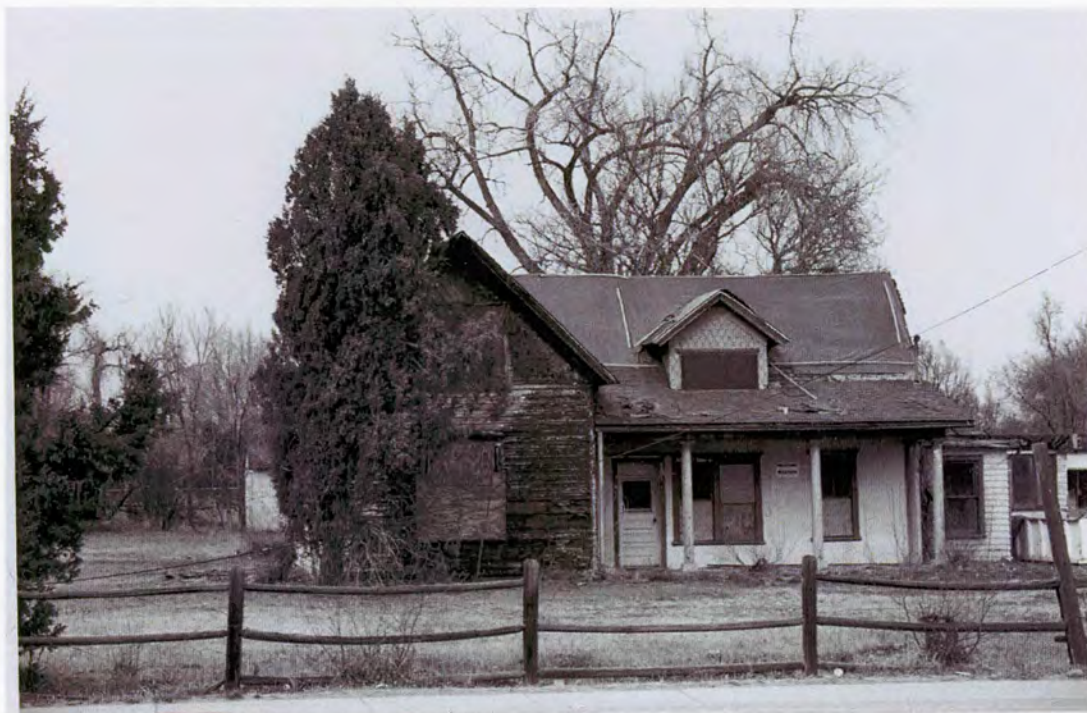
Figure 3: Baugh House, 1999, on file with the Office of Archaeology and Historic Preservation, Denver, Colorado
