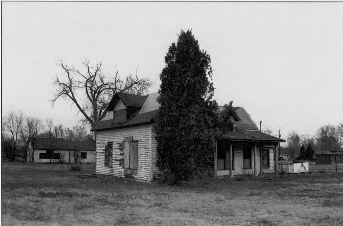
Figure 4: Baugh House, 1999, on file with the Office of Archaeology and Historic Preservation, Denver, Colorado
