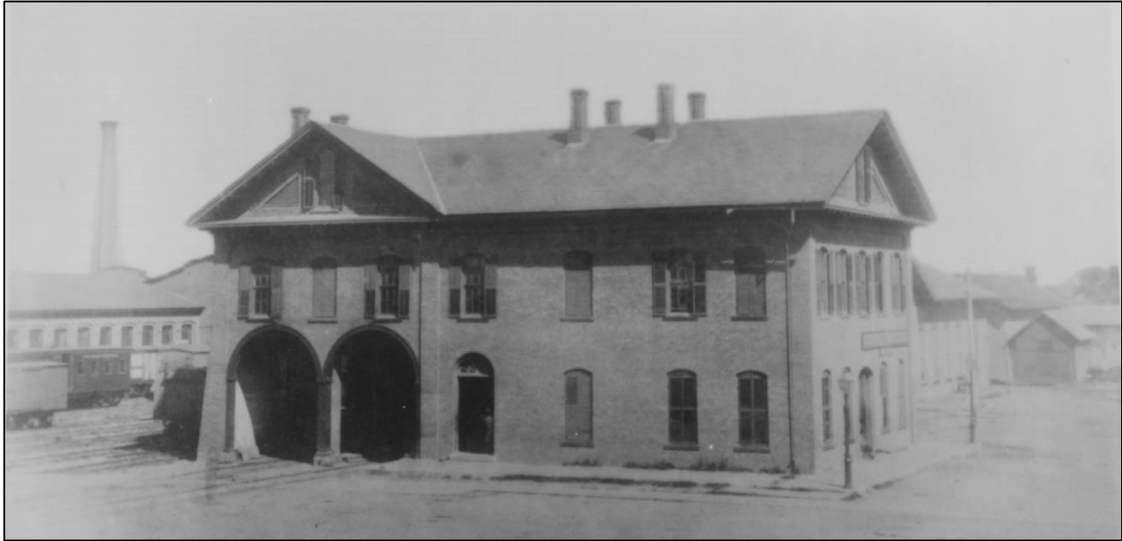
Fig. 3 c. 1863 view of first St. Albans station with new Machine Shop (HD # 4) in background. This structure was replaced with the larger train shed in 1865-1867. [Courtesy Collection of Jim Murphy]
