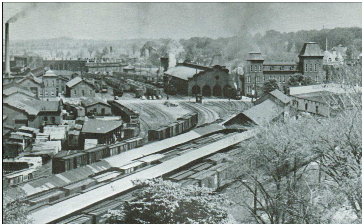
Fig. 17 1940 view looking north of Vermont Central's St. Albans complex with (l. to r.) Car Shop (HD #8) and Storage building (HD #12) in foreground on left, Machine Shop in background (HD #4), Maintenance Shop (HD #5), roundhouse complex in far background (HD #6), Yard Office (HD #3), train shed, headquarters office building (HD #1) and in foreground the freight house and platforms (HD #7) Note: corner tower gone from train shed and chimneys gone from office building [From Jones, Vol. 4, p. 170, Collection of Jim Murphy]
