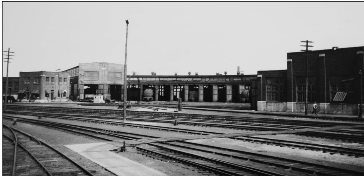
Fig. 12 c. 1925 view of new roundhouse and turntable facilities (HD # 6, 6a, & 6b), looking northeast [Courtesy Collection of Jim Murphy]
