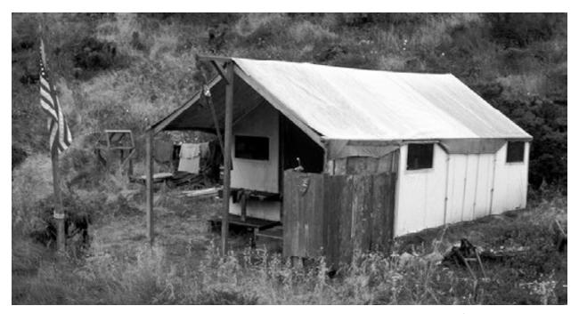
Figure 5-8. The rangers' tent in Nidever Canyon on San Miguel Island eventually was reinforced with wood but the occupants still regularly suffered from rain, wind, and mice. This led to the decision to use Conex boxes.
