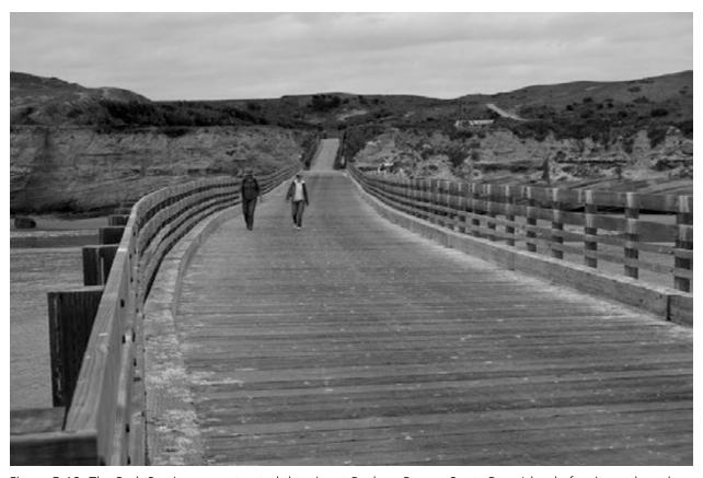
Figure 5-12. The Park Service reconstructed the pier at Bechers Bay on Santa Rosa Island after it purchased the island in 1986 and constructed an entirely new pier in 2011. It could handle entire herds of cattle as well as large trucks and heavy equipment.
