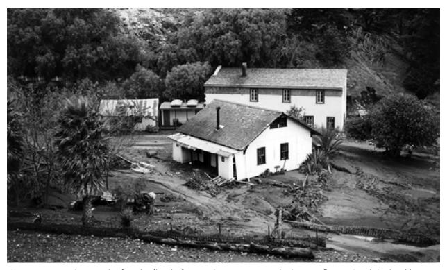
Figure 8-5. Scorpion Ranch after the flood of December 5–6, 1997. The intense flow twisted the bunkhouse off its foundation and wiped out the blacksmith shop.
