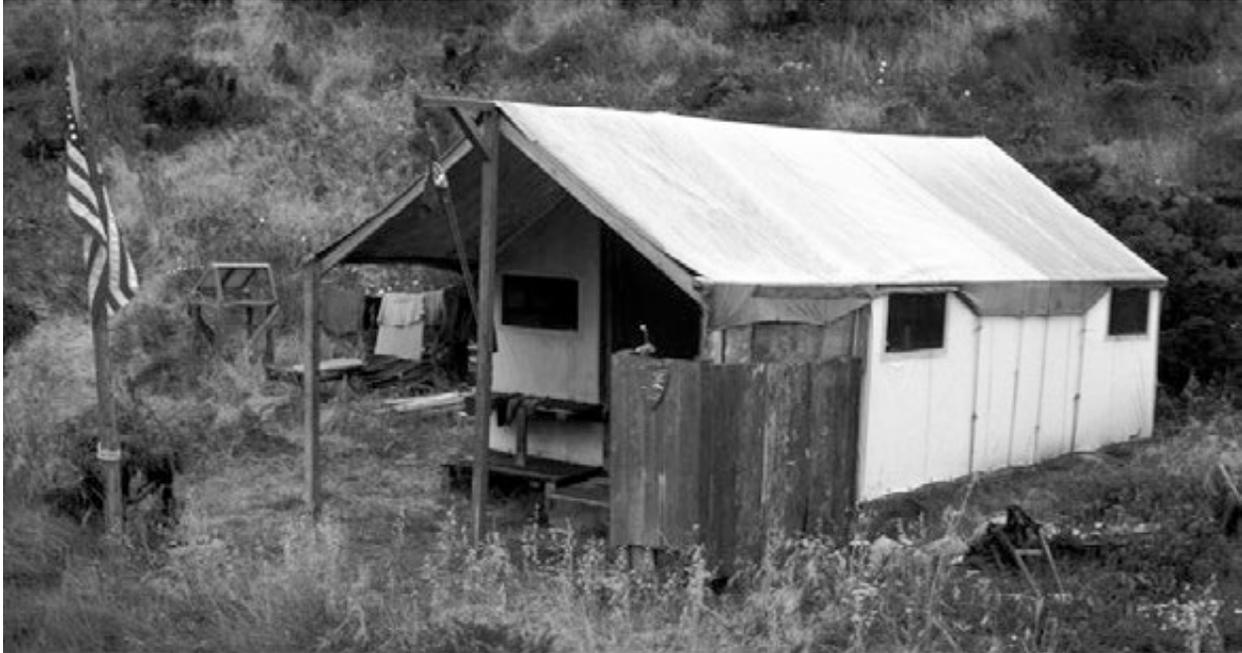
Figure 5-8. The rangers' tent in Nidever Canyon on San Miguel Island eventually was reinforced with wood but the occupants still regularly suffered from rain, wind, and mice. This led to the decision to use Conex boxes.
