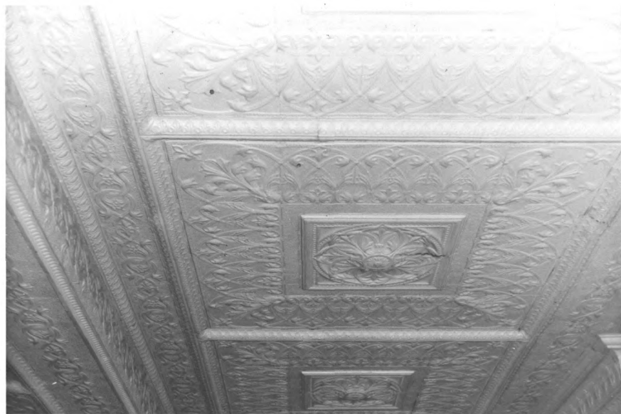
PRESSED METAL COURTROOM CEILING
