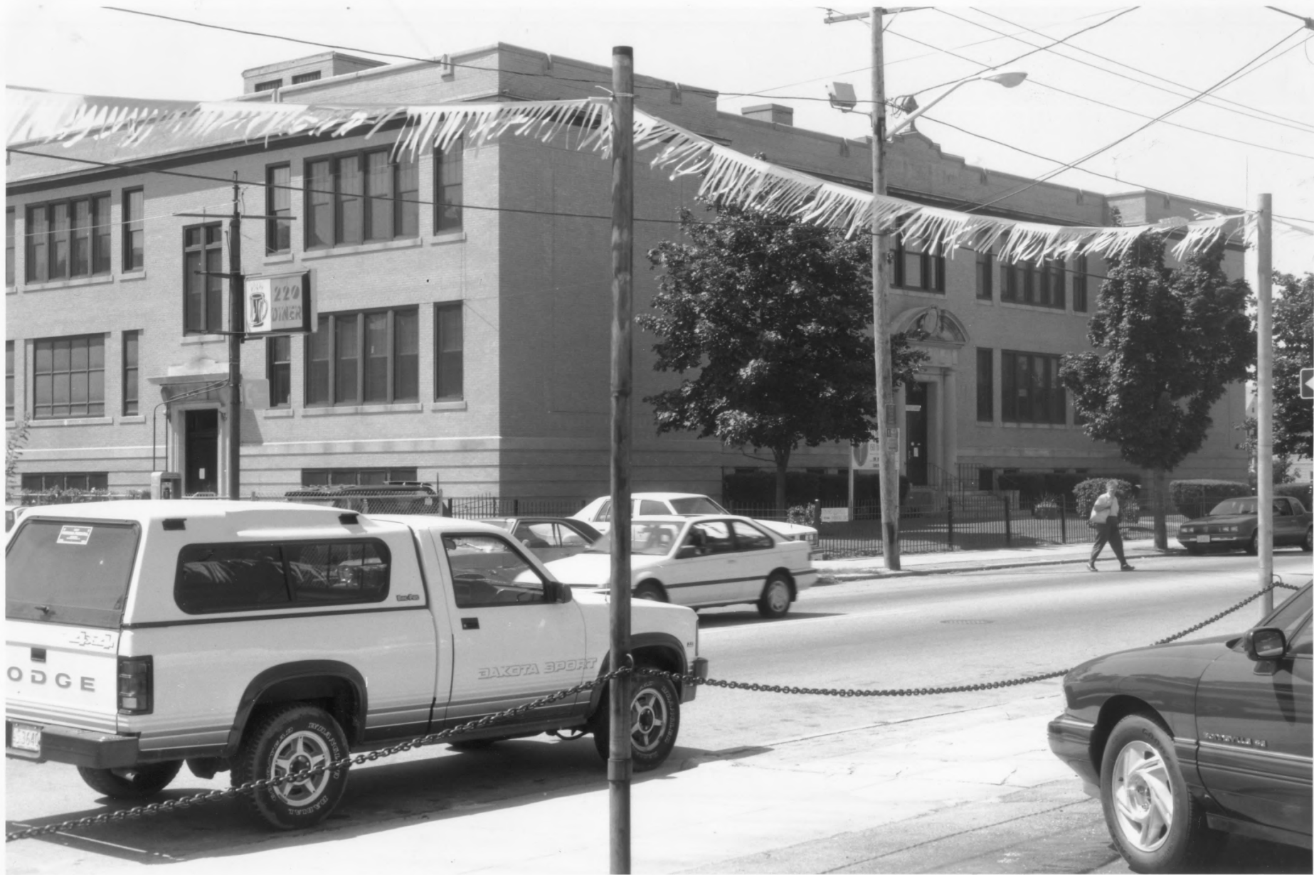
Smith Hill Historic District Providence County Providence, R.I. Photo #1 of 9
