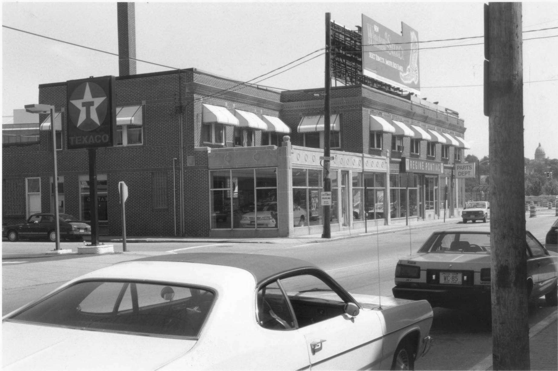
Smith Hill Historic District Providence County Providence, R.I. Photo #3 of 9
