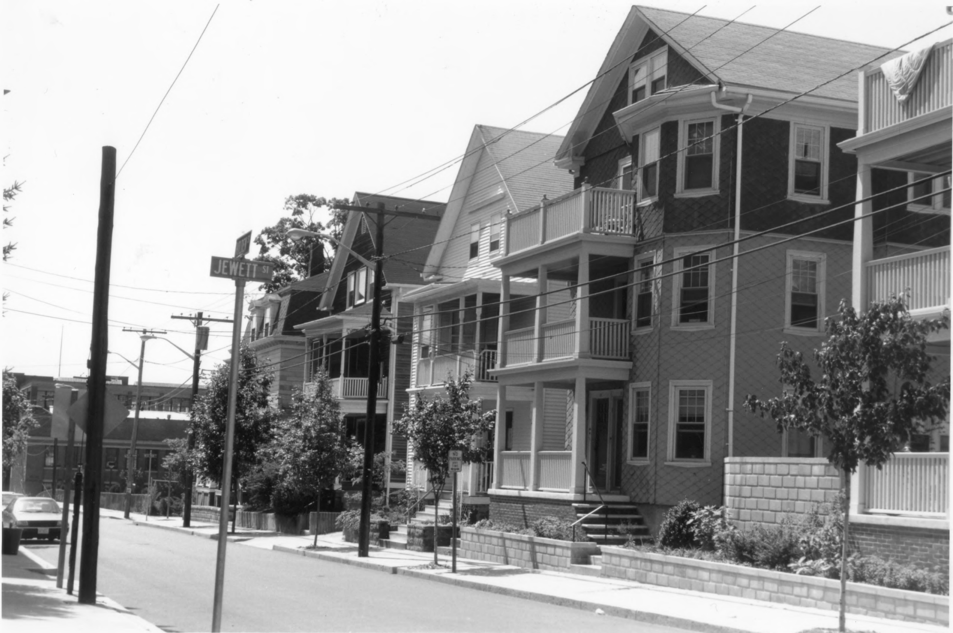
Smith Hill Historic District Providence County Providence, R.I. Photo # 4 of 9
