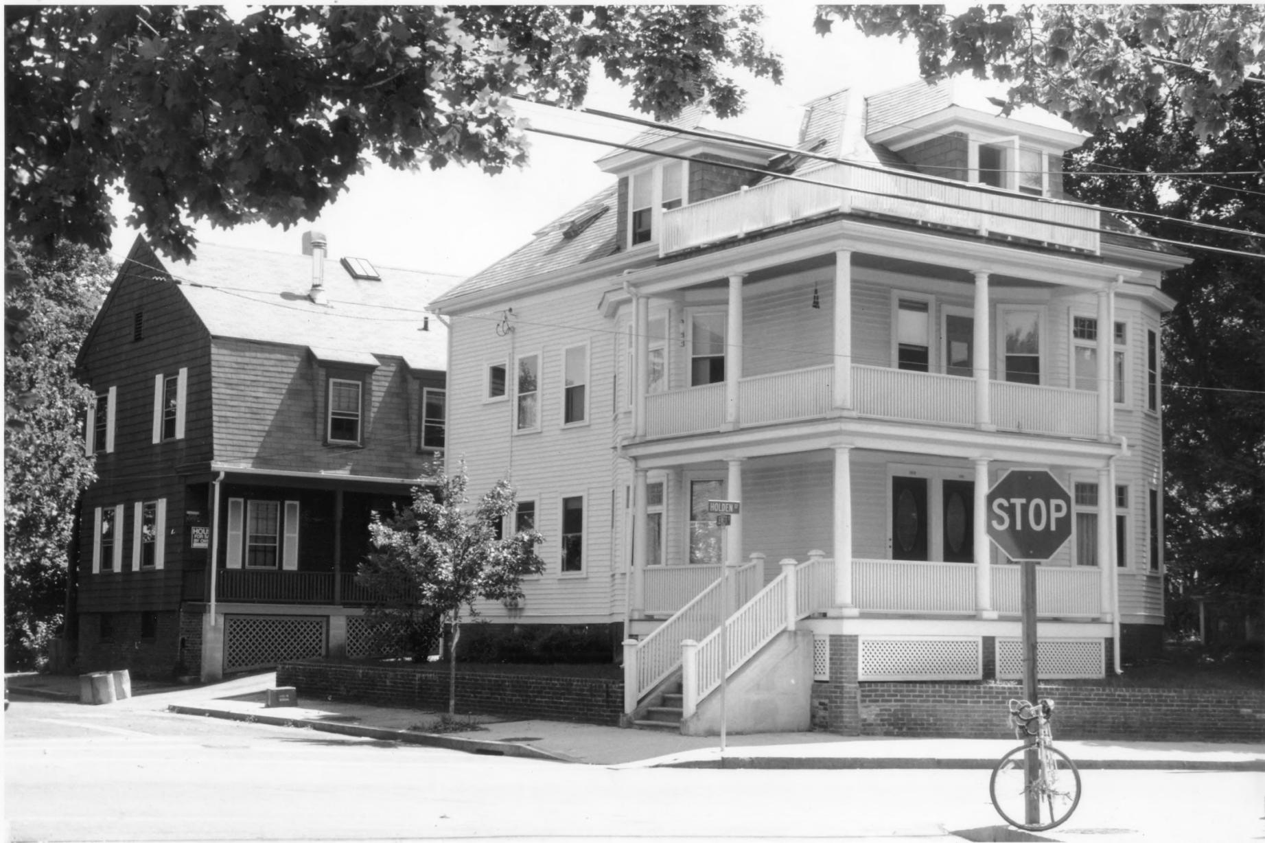
Smith Hill Historic District Providence County Providence, R.I. Photo #5 of 6
