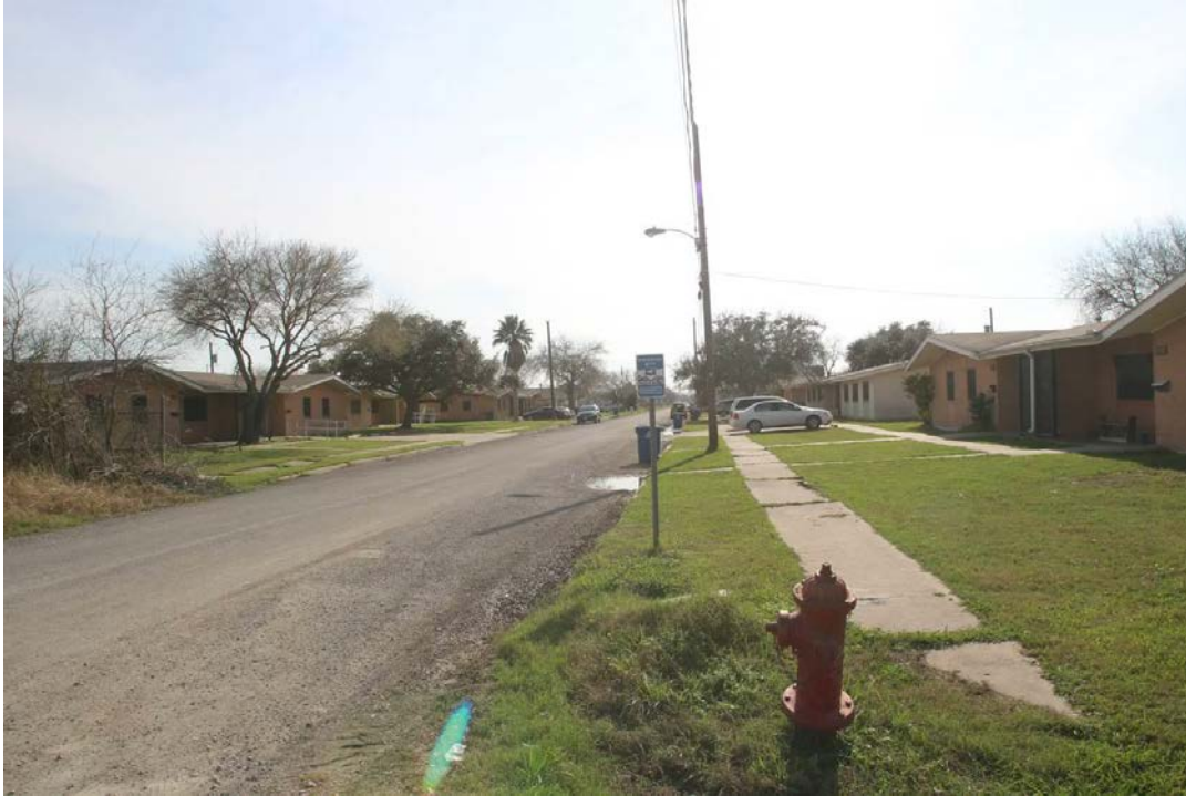
Photo 5 View of Industrial Street, looking south
