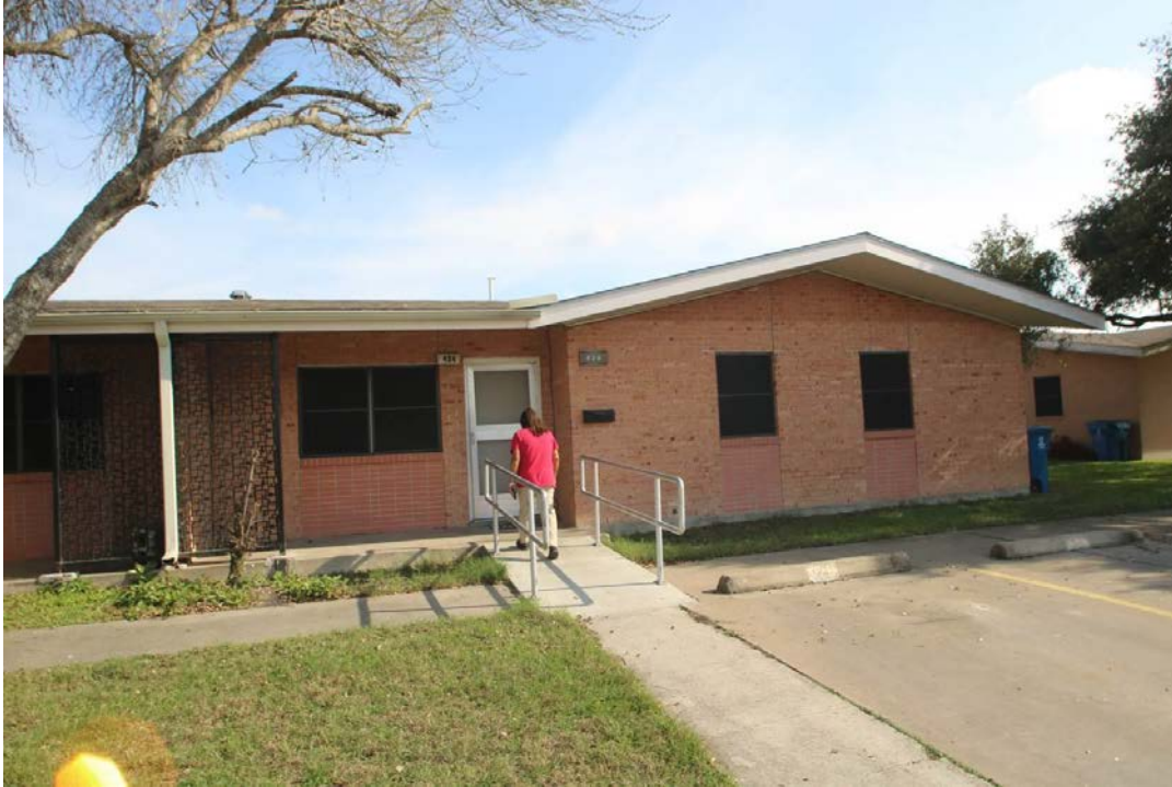
View of Building 1, looking southeast
