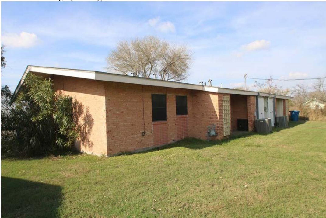
View of Building 1, looking northwest
