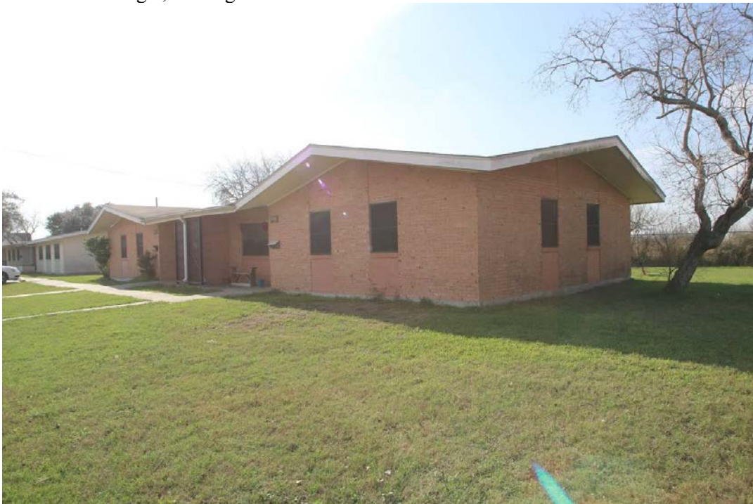
Photo 6 View of Building 6, looking southwest
