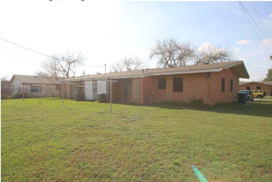
Photo 2 View of Building 3, looking southwest
