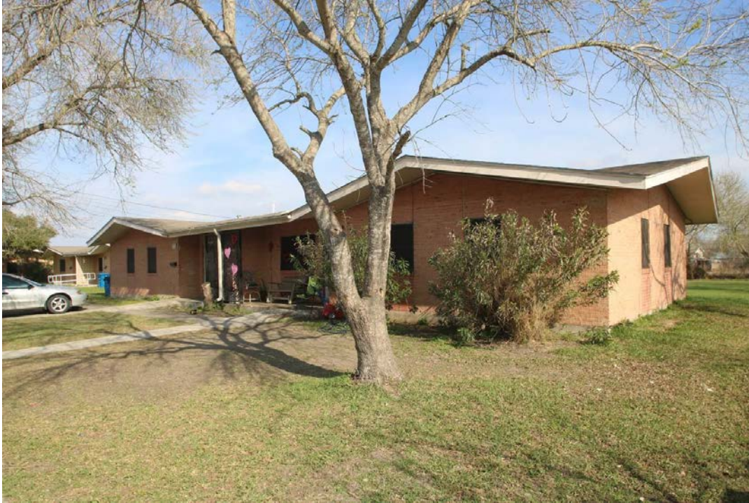
Photo 1 View of Building 3, looking northeast
