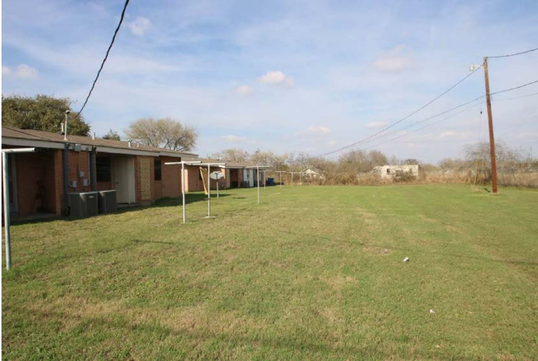
View of Rear Lawn with Building 2 (left) and Building 3 (right), looking northeast
