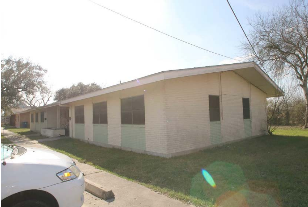
Photo 7 View of Building 5, looking southwest
