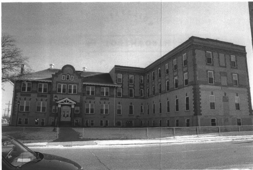
Photo #2. Holy Rosary Hospital west elevation. View to east.
