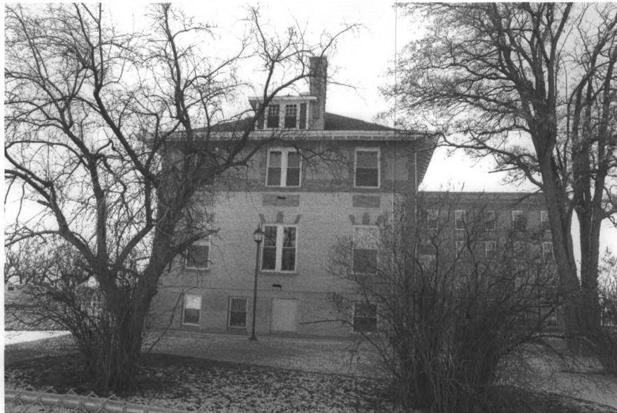
Photo #8. Holy Rosary Hospital north elevation. View to south.
