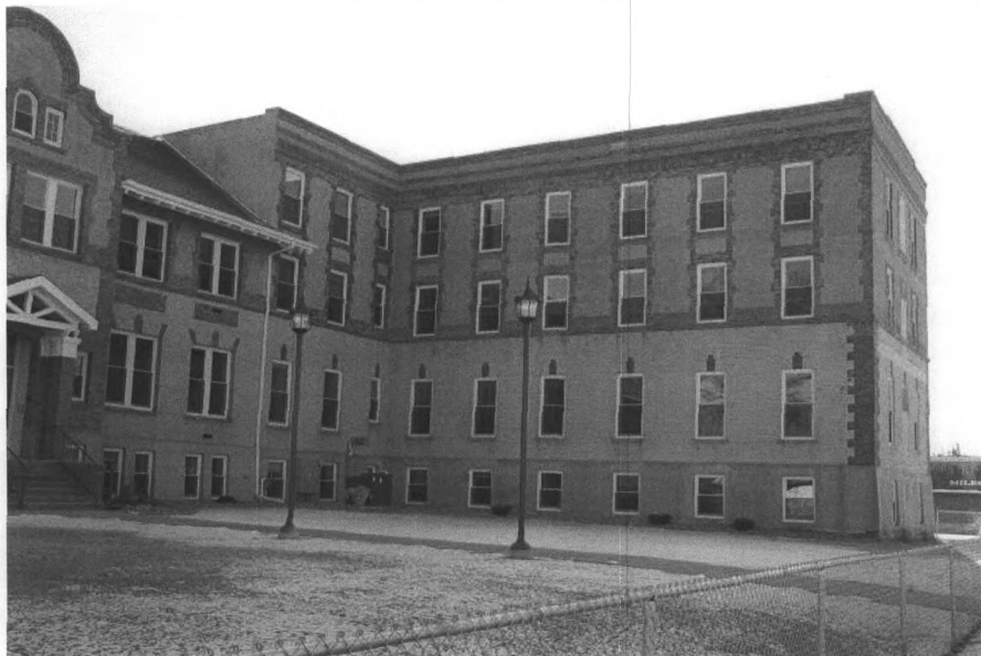
Photo #9. Holy Rosary Hospital, north elevation of 1922 annex. View to southeast.
