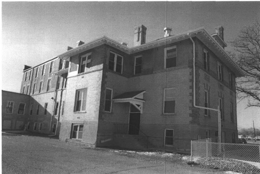
Photo #7. Holy Rosary Hospital, east and north elevations. View to southwest.
