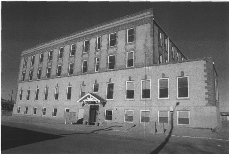
Photo #5. Holy Rosary Hospital, south elevation of 1922 annex. View to north-northwest.
