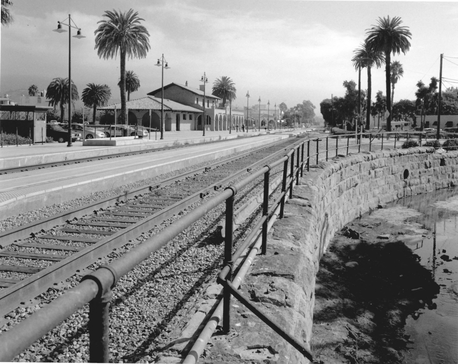
Southern Pacific Train Depot, Santa Barbara County, CA #12
