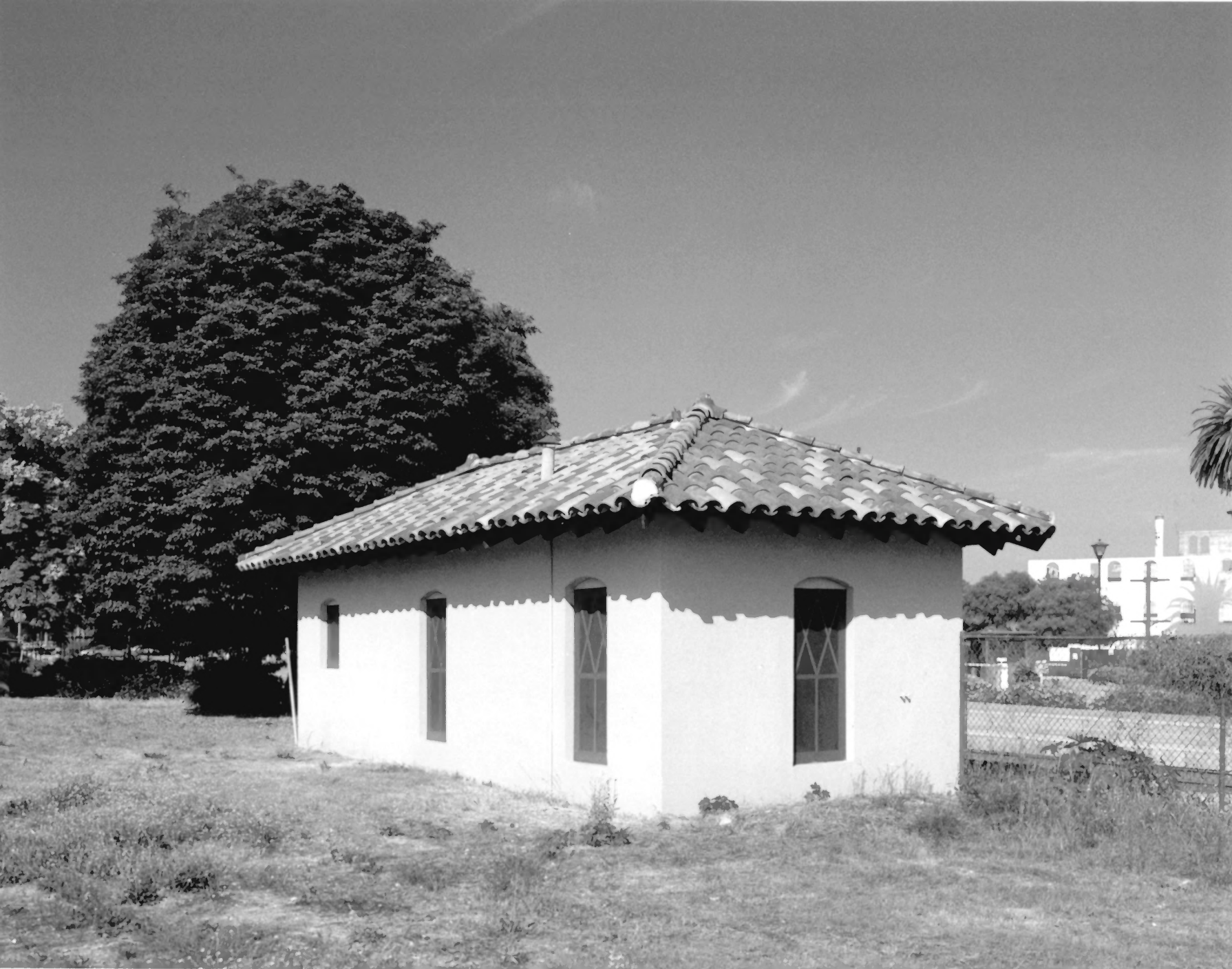
Southern Pacific Train Depot. Santa Barbara County, CA #5
