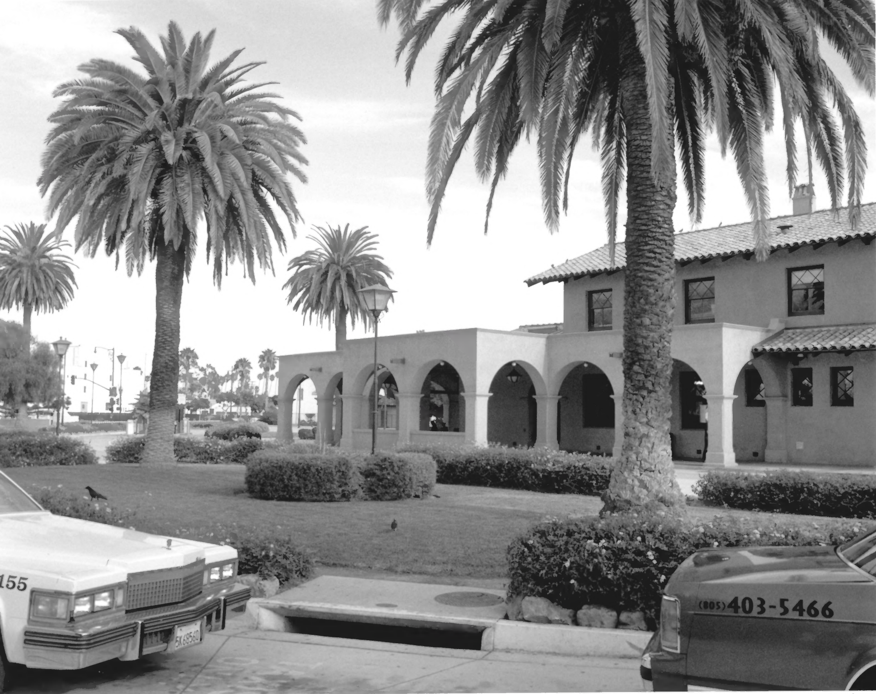
southern Pacific Train Depot. Santa Barbara County, CA #9
