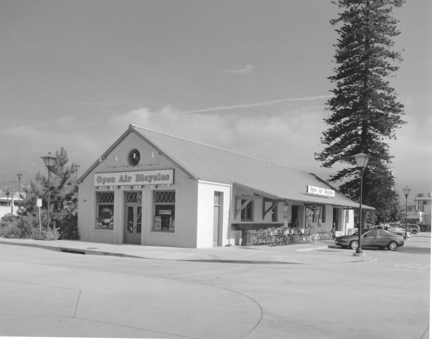
Southern Pacific Train Depot, Santa Barbara County, CA #4
