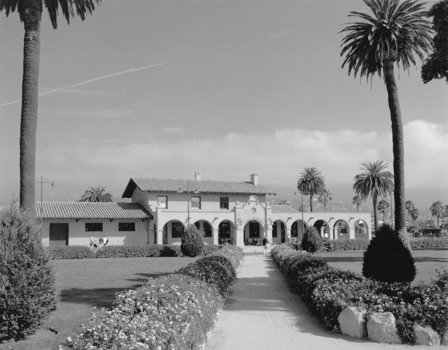
Southern Pacific Train Depot, Santa Barbara County, CA #6
