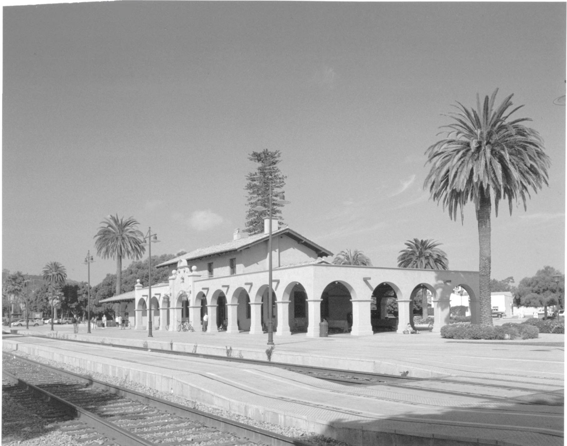
Southern Pacific Train Depot. Santa Barbara County, CA #1
