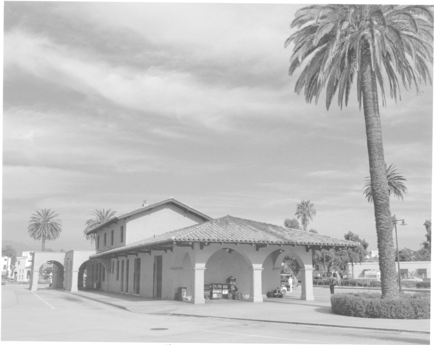
Southern Pacific Train Depot. Santa Barbara County, CA #2
