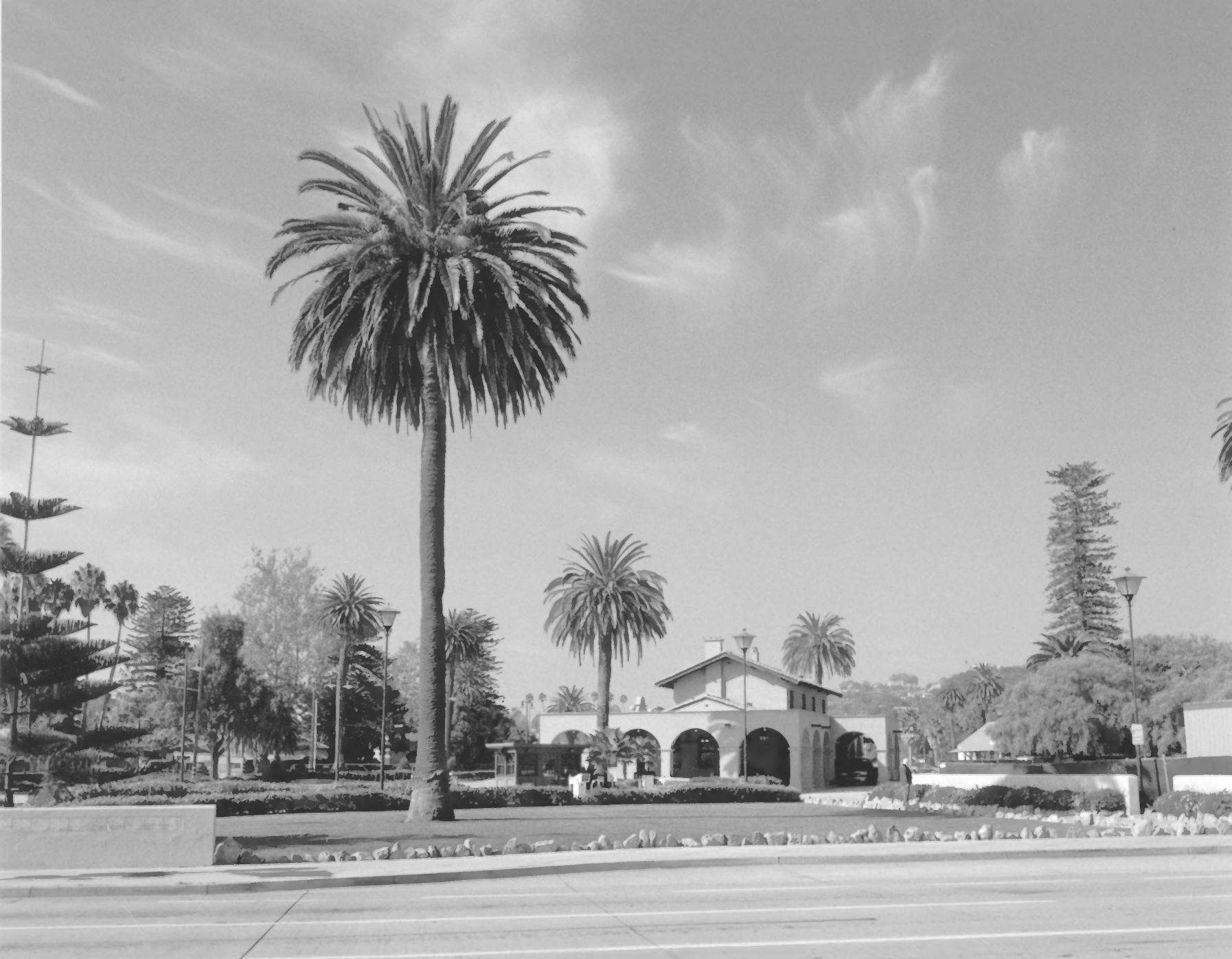
Southern Pacific Train Depot. Santa Barbara County, CA #8
