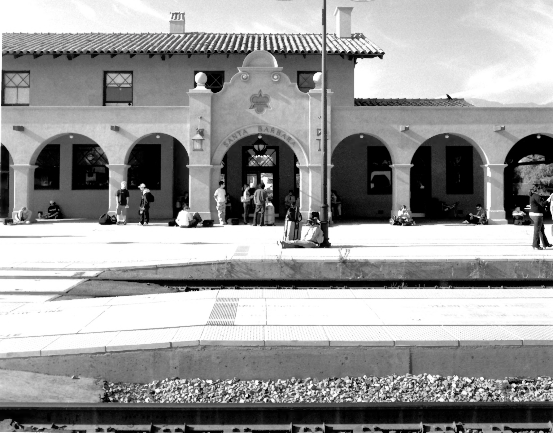
Southern Pacific Train Depot, Santa Barbara County, CA #3
