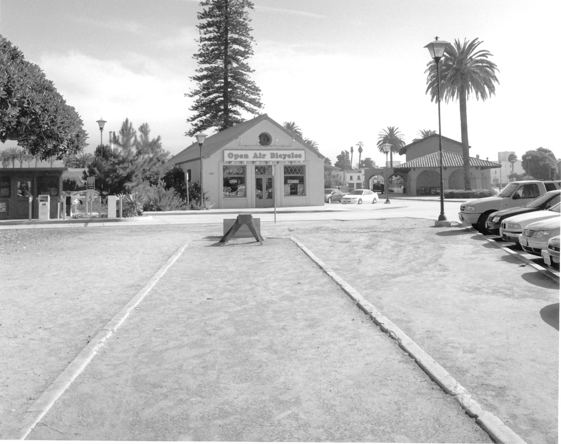
Southern Pacific Train Depot, Santa Barbara County, CA #11
