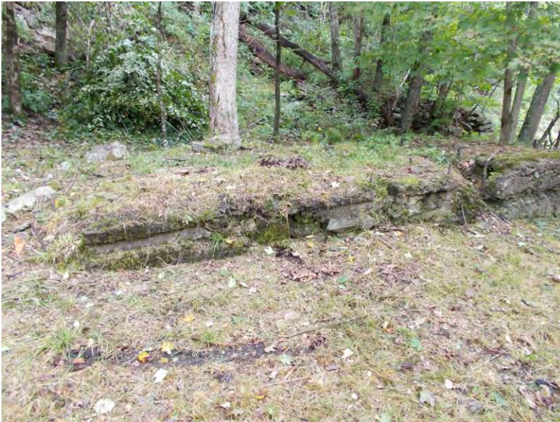
Photo 7: WV_RaleighCounty_BeckleyMillSite_0007 Engine mount, view facing north.
