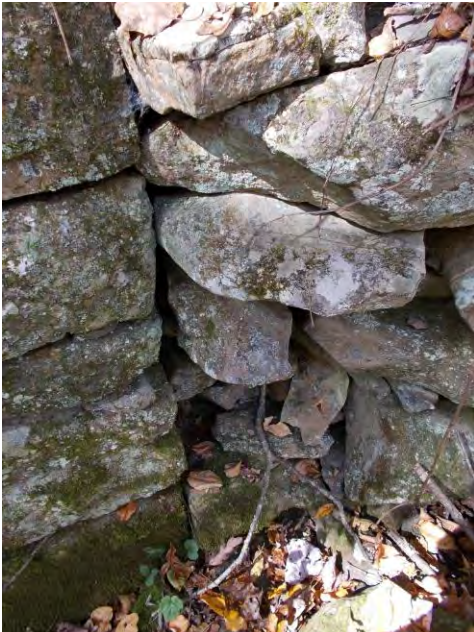
Photo 5: WV_RaleighCounty_BeckleyMillSite_0005 Detail of front of wheel well, view facing west.
