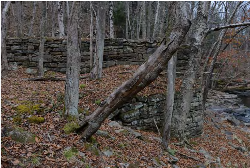
Photo 20: WV_RaleighCounty_BeckleyMillSite_0020 Looking north at the south wall of the bridge abutment.
