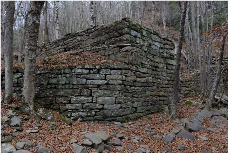
Photo 19: WV_RaleighCounty_BeckleyMillSite_0019 Looking northwest at the south and east walls of the bridge abutment.
