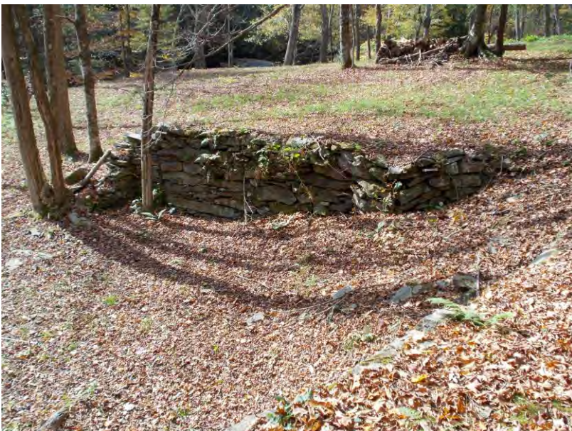
Photo 10: WV_RaleighCounty_BeckleyMillSite_0010 Building foundation, view facing west.
