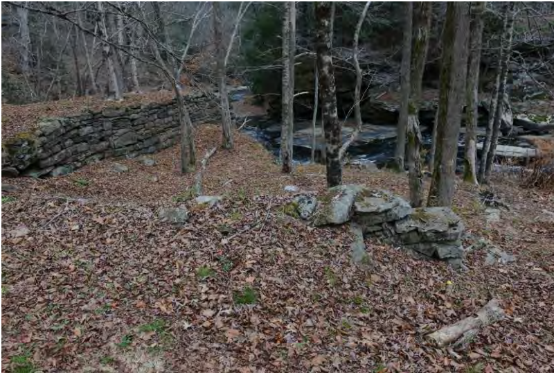
Photo 25: WV_RaleighCounty_BeckleyMillSite_0025 Looking east across the building foundation toward the bridge abutment and Piney Creek.
