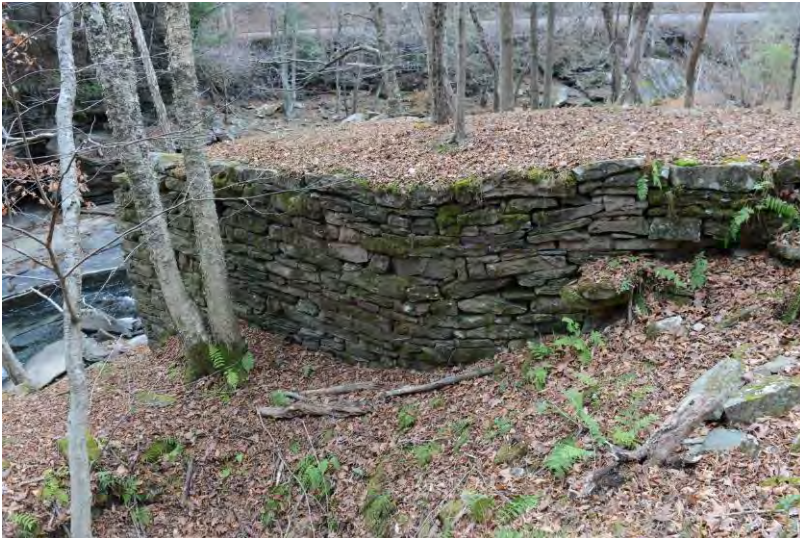
Photo 21: WV_RaleighCounty_BeckleyMillSite_0021 Looking south at the north wall of the bridge abutment.
