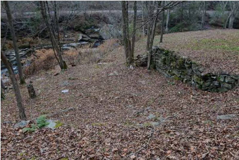
Photo 23: WV_RaleighCounty_BeckleyMillSite_0023 Looking south at the building foundation (on right).
