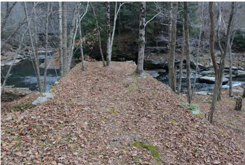
Photo 22: WV_RaleighCounty_BeckleyMillSite_0022 Looking east across the top of the bridge abutment.
