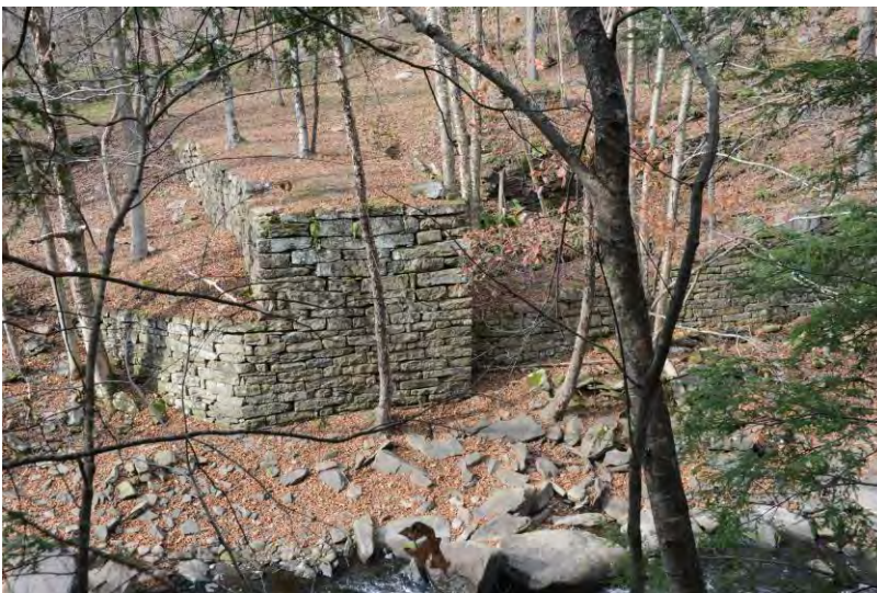
Photo 8: WV_RaleighCounty_BeckleyMillSite_0008 Bridge abutment, view facing west.
