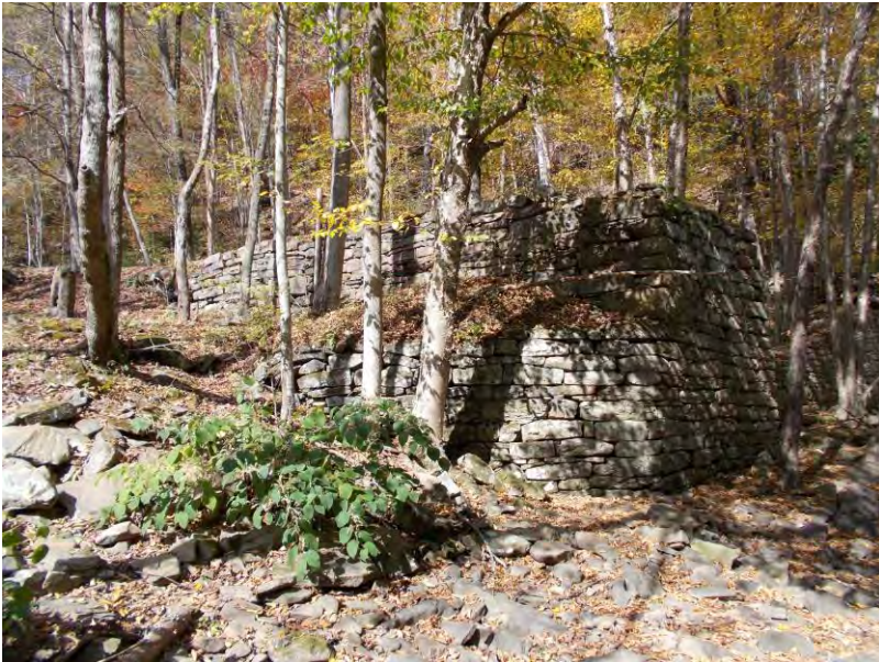
Photo 9: WV_RaleighCounty_BeckleyMillSite_0009 Bridge abutment retaining wall, view facing north.
