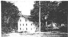
Bogert's Mill, corner of Bogert's Mill Road and Starling Green, Harrington Park, opposite the residence of John J. Bogert, first mayor of the Borough, 1884 to 1886. The mill was torn down about 1915. See above 1888 plans and see N. the home of Mr. and Mrs. Firdes Condit.
