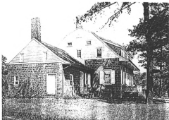
End elevation of the Demarest House (see below).
