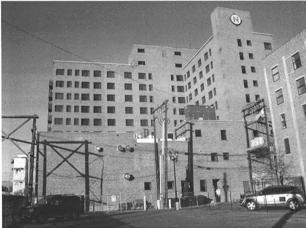
0006 of 0010. East and south sides, view to west
