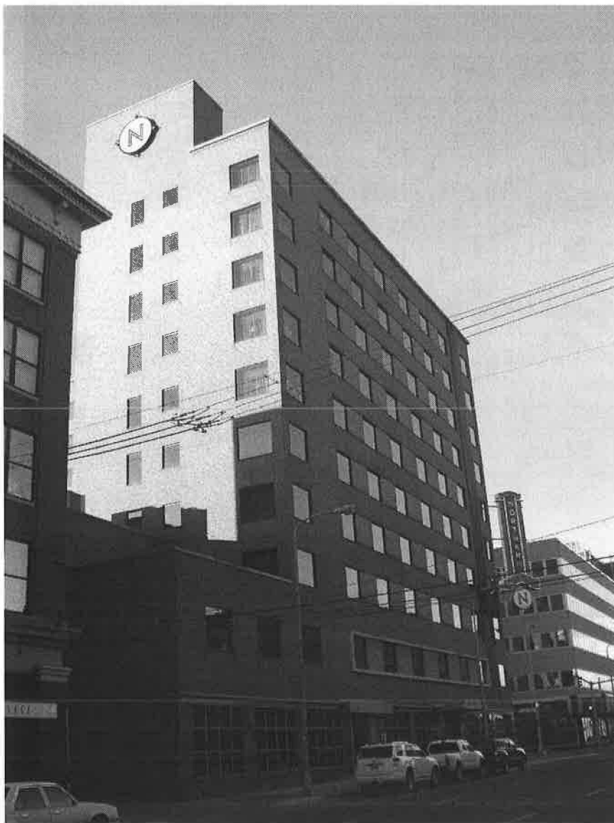
0005 of 0010. North and East sides, view to southwest
