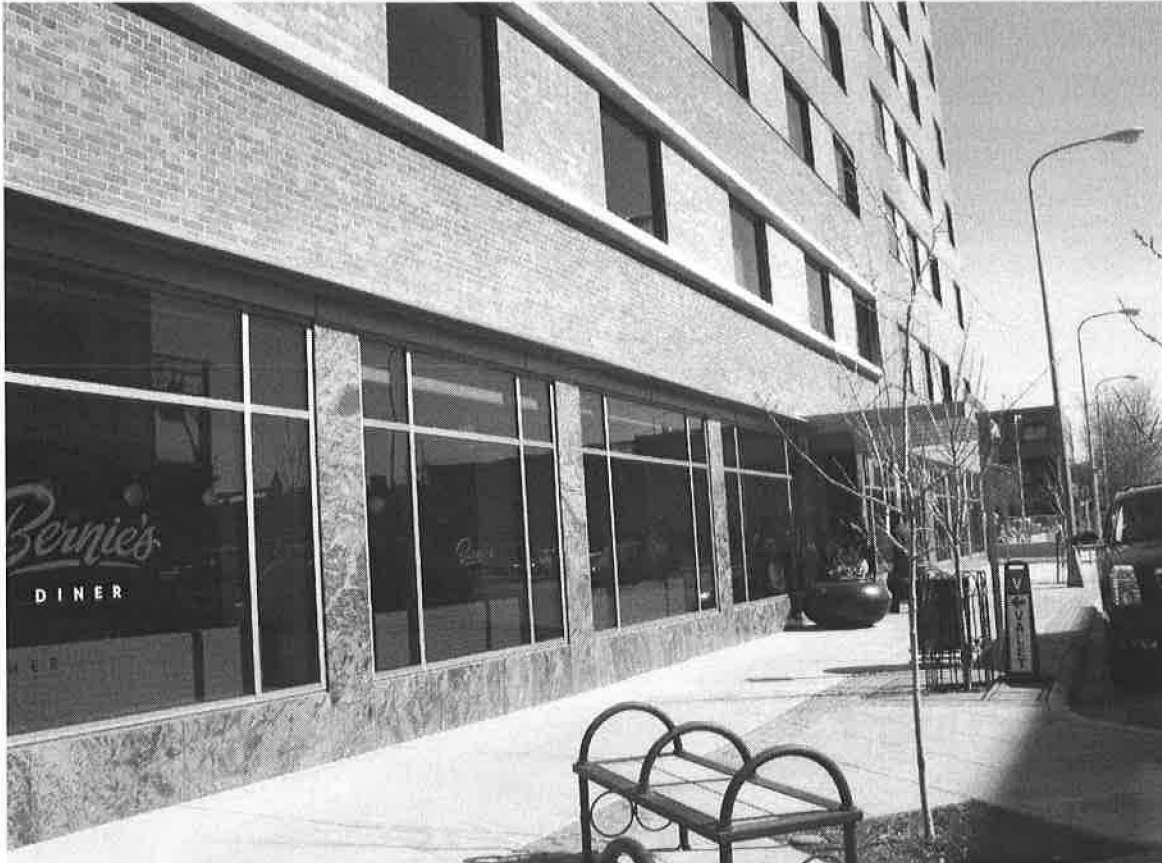
0010 of 0010. Facade North Broadway, view to south
