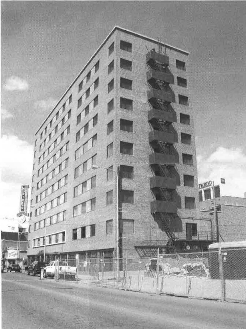
0003 of 0010. South and West sides, view to north
