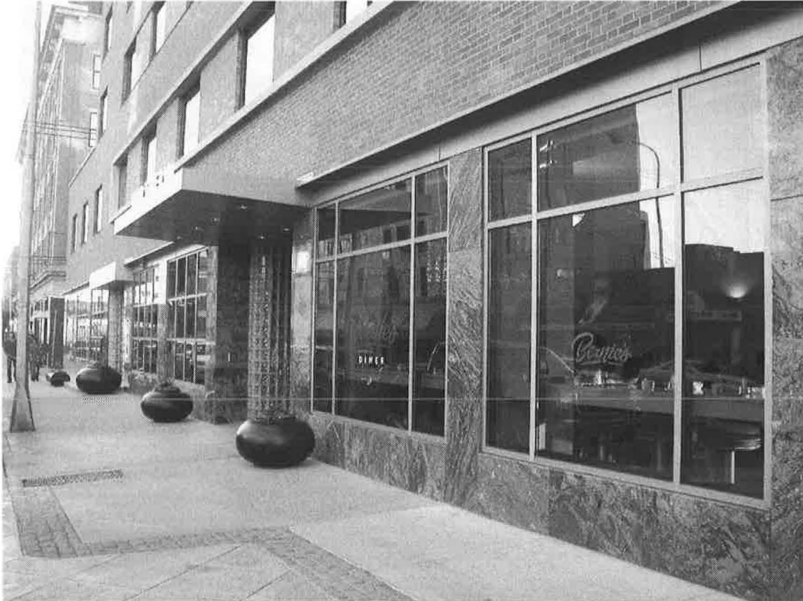
0009 of 0010. Facade 1st Ave North, view to east
