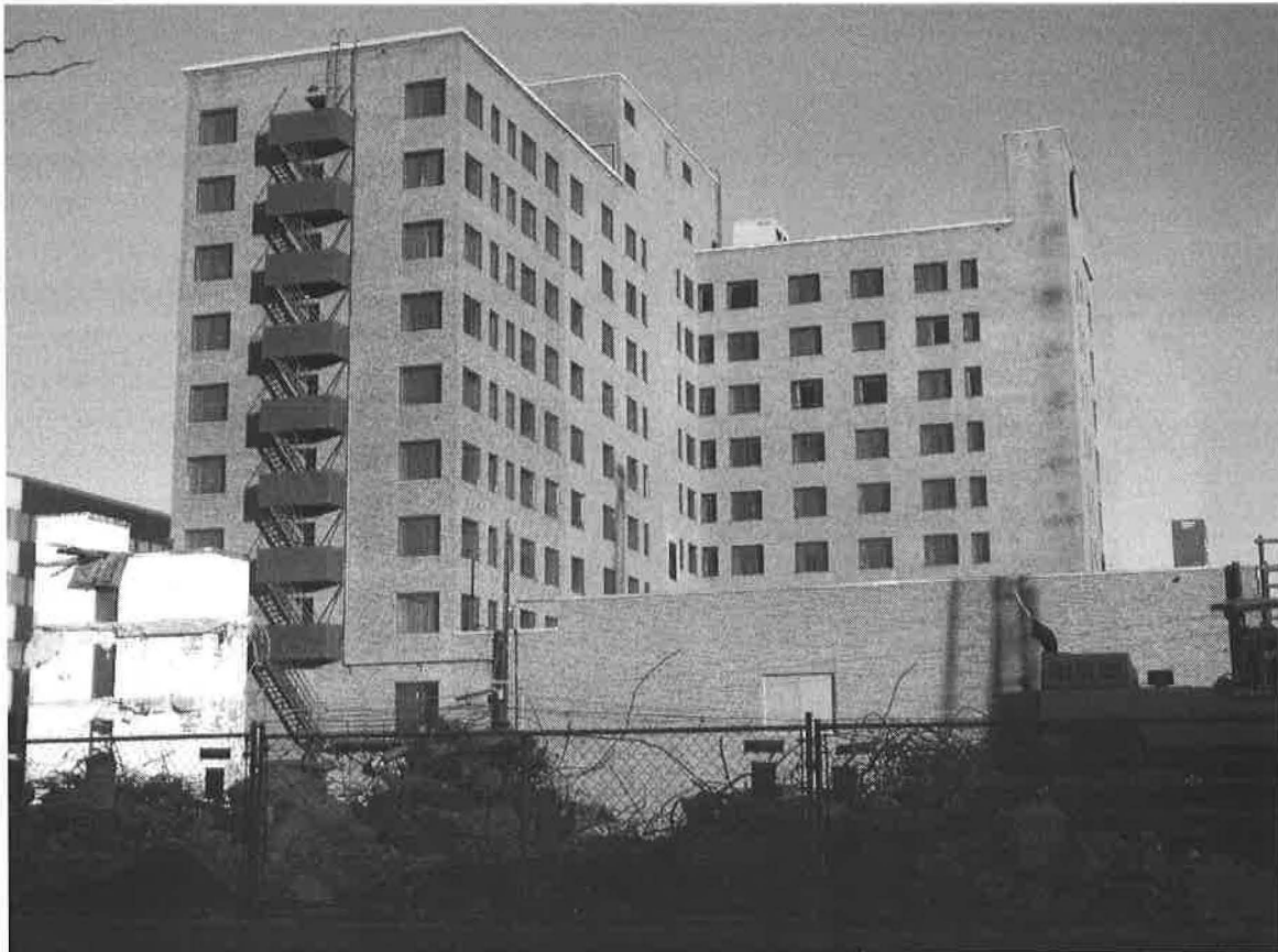
0004 of 0010. South and East sides, view to northwest
