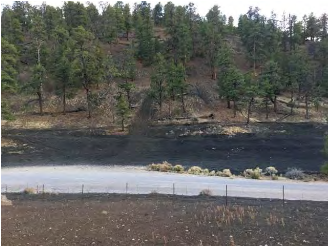
Fig. 51. View looking south across the non-contributing half of Station Five. Forest Service road 776 (gray gravel) is just beyond the USFS easement fence. Note the cinder disruption and tracks due to OHV use. (Photo by author. November 4, 2018).
