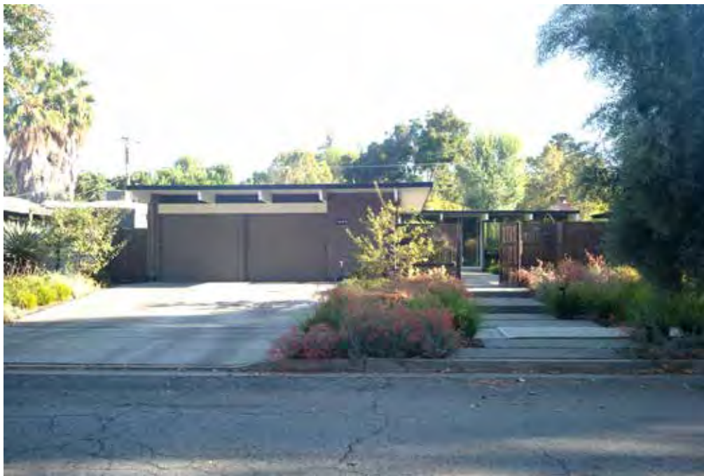
Fairglen Additions Santa Clara County, CA Photo 9 of 20 (SJ-1004) (196)
