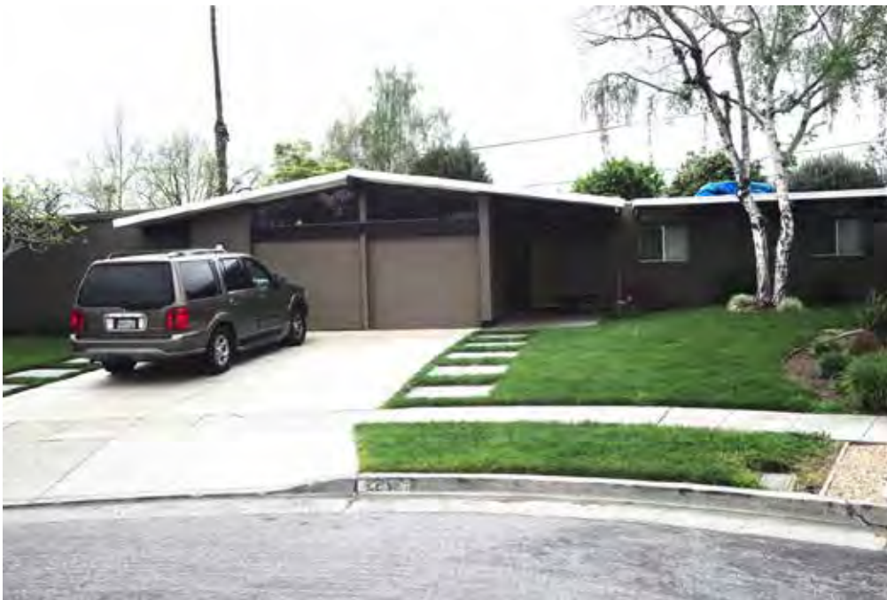
Fairglen Additions Santa Clara County, CA Photo 15 of 20 (SJ-733) (131)
