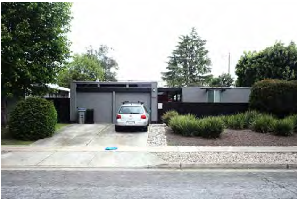
Fairglen Additions Santa Clara County, CA Photo 8 of 20 (SJ-1003) (98)
