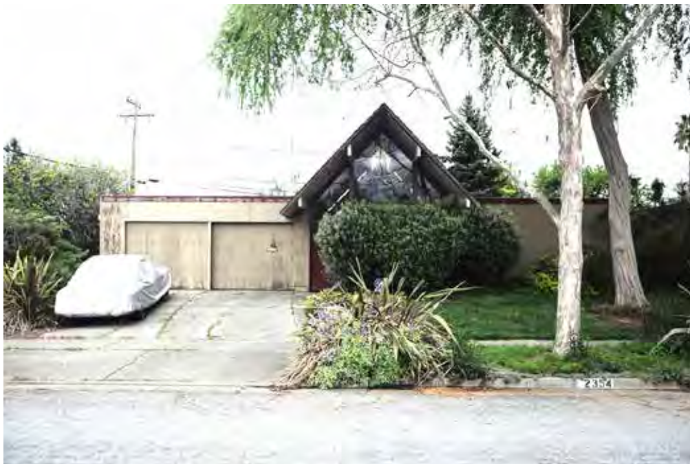
Fairglen Additions Santa Clara County, CA Photo 19 of 20 (SJ-4D) (76)
