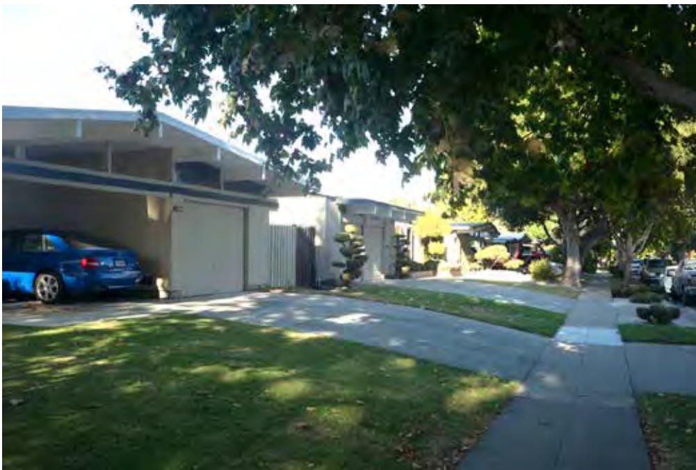
Fairglen Additions Santa Clara County, CA Photo 4 of 20 (Fairwood Ave)
