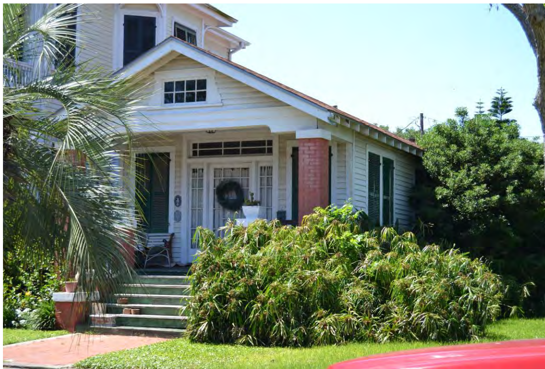
Photo No. 32. Oblique view of 1714 Avenue K (RID 698533). View facing northwest. April 2015.
