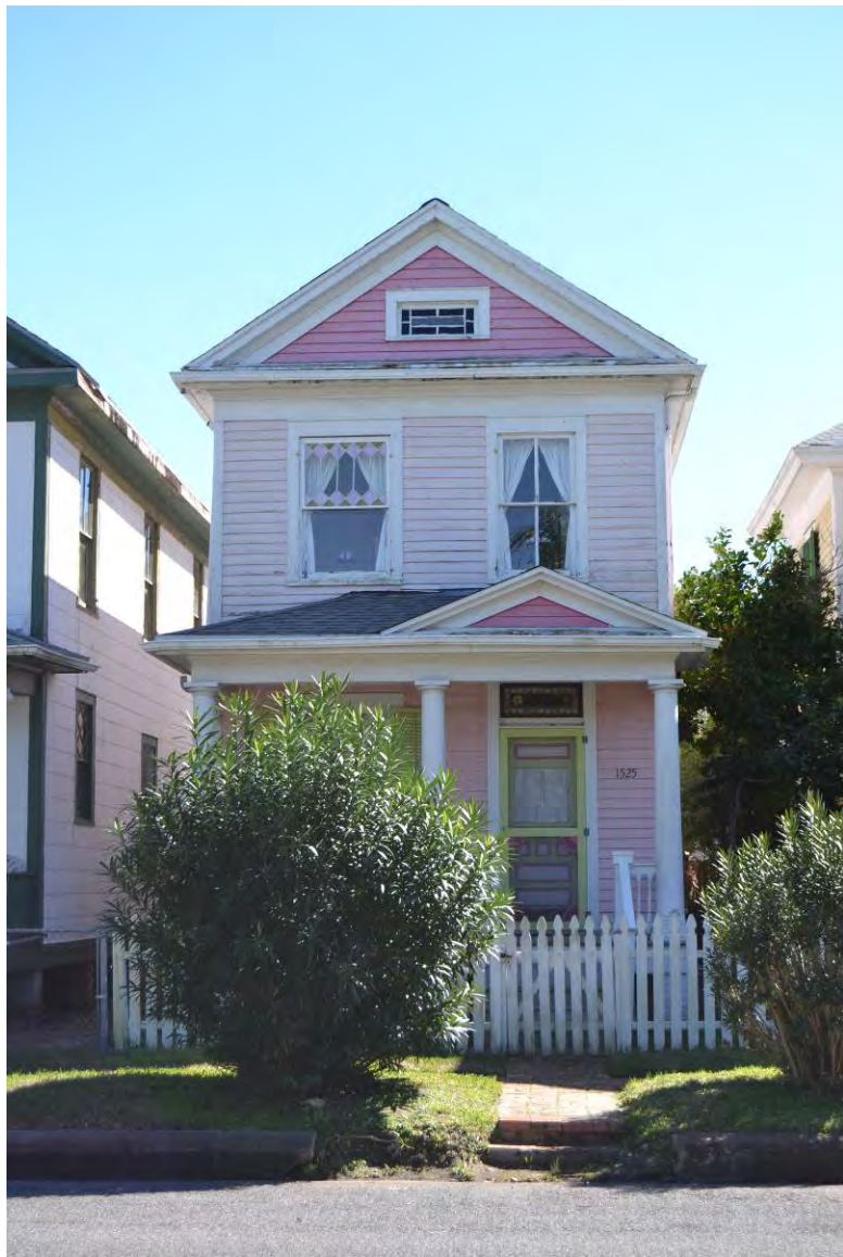
Photo No. 30. Façade of 1525 Avenue M (RID 688325). View facing south. February 2016.
