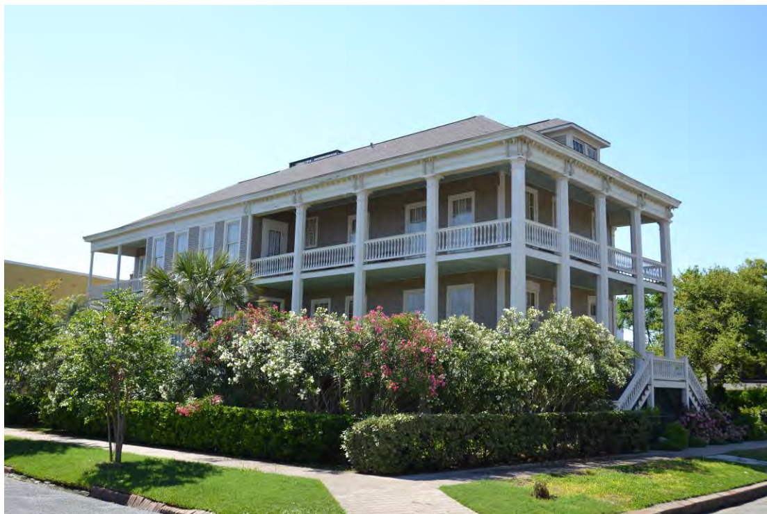
Photo No.13. Oblique view of 1019 16th Street (RID 689522). View facing northwest. April 2015.
