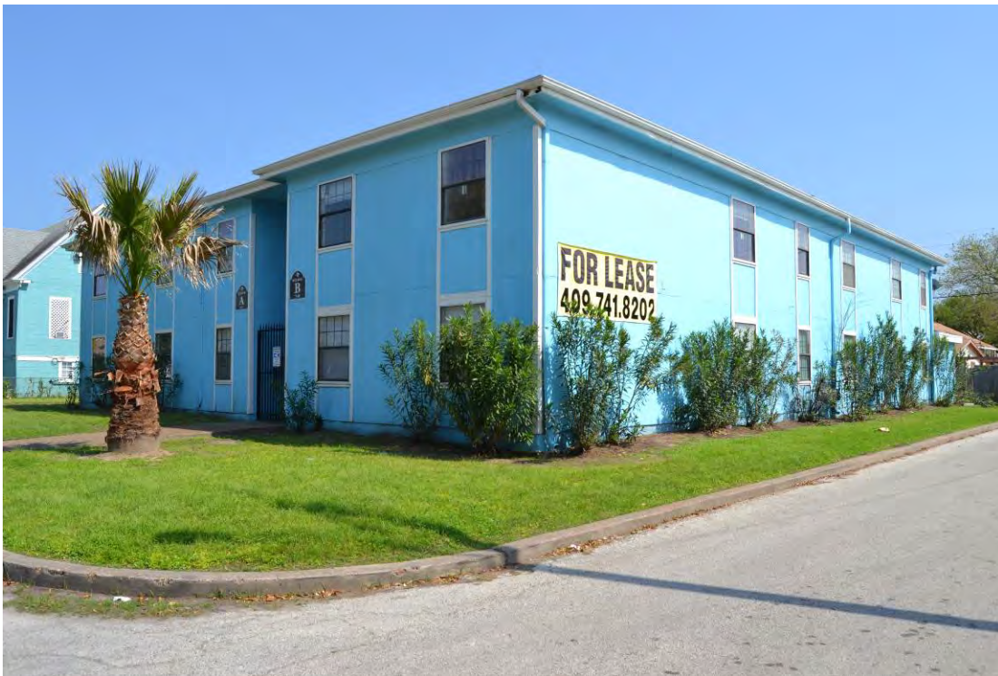
Photo No. 20. Oblique view of 1927 Avenue M½ (RID 688193). View facing southeast. April 2015.
