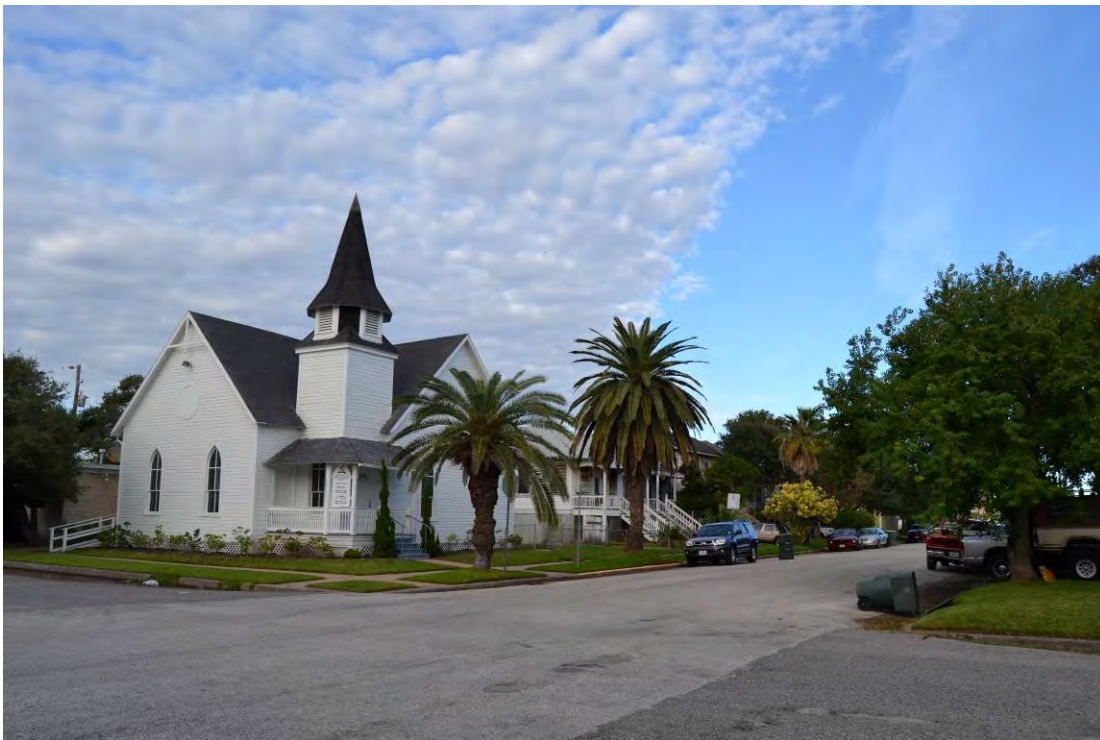
Photo No. 2. Oblique view of the church (RID 688300a) in the Lost Bayou Historic District. View facing northeast. November 2015.
