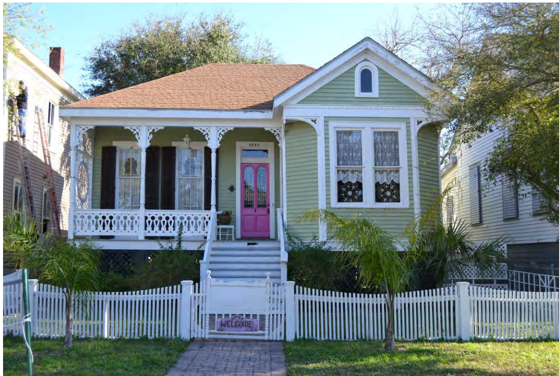
Photo No. 11. Façade of 1421 Avenue L (RID 6835). View facing south. February 2016.
