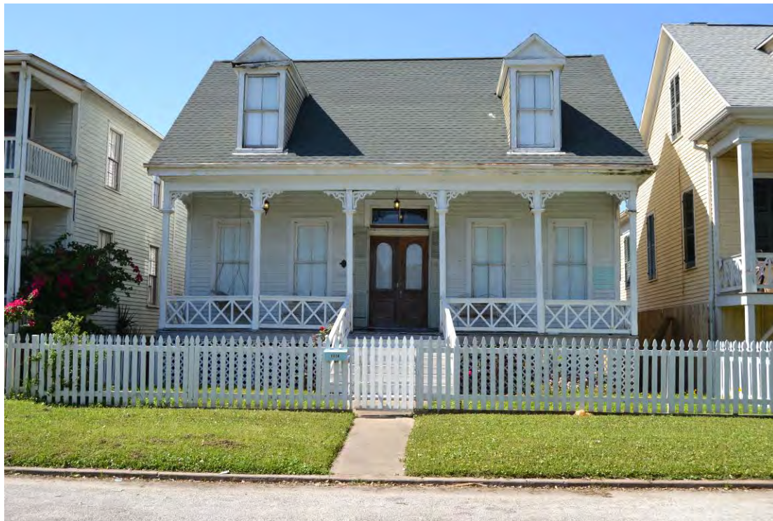
Photo No. 34. Façade of 1714 Avenue M½ (RID 688237). View facing north. April 2015.
