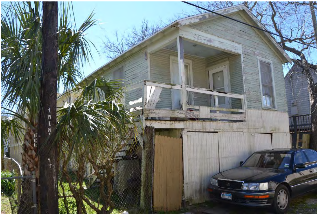
Photo No. 37. Oblique view of alley house at 1524 Avenue L (RID 689273b). View facing southwest. February 2016.
