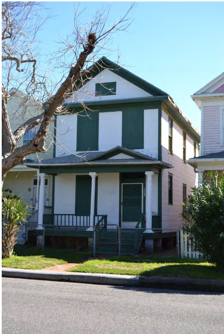
Photo No. 29. Façade of 1523 Avenue M (RID 688326). View facing southeast. February 2016.
