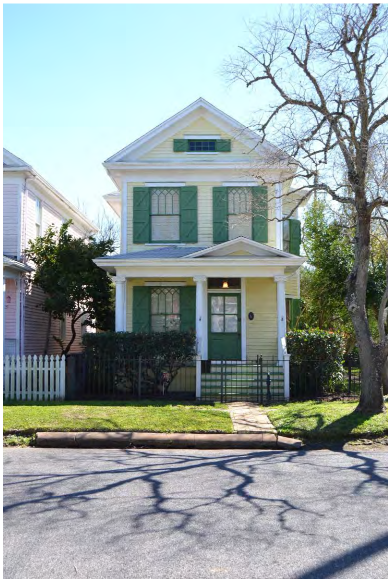
Photo No. 31. Façade of 1527 Avenue M (RID 688324). View facing south. February 2016.
