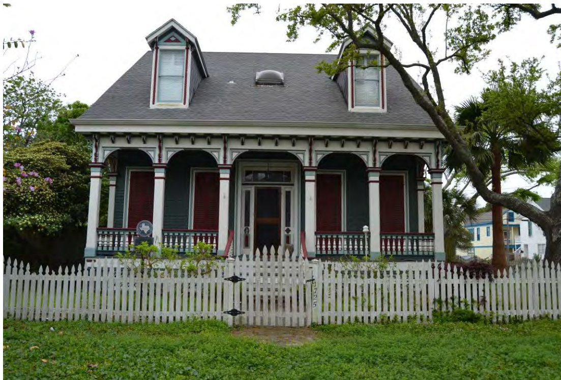
Photo No. 10. Façade of 1725 Avenue M (RID 688226a). View facing south. April 2015.
