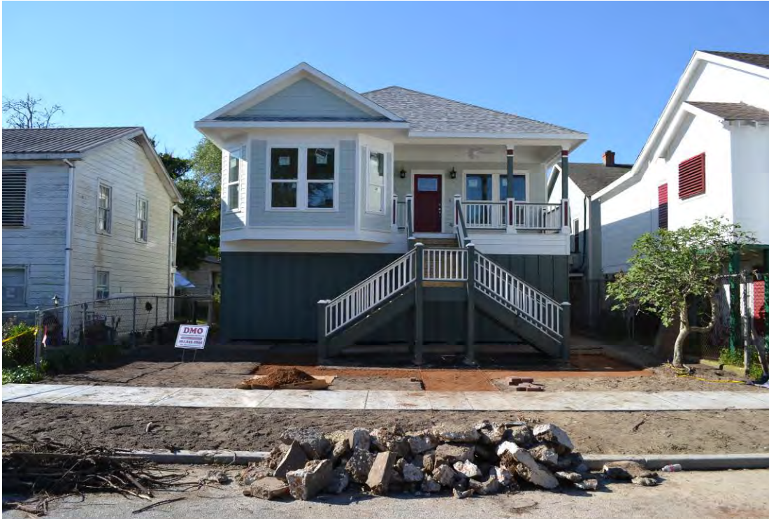
Photo No. 19. Façade of 1623 Avenue L (RID 683525). View facing west. April 2015.
