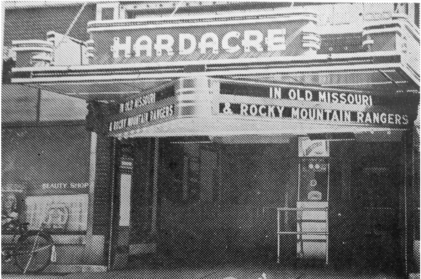
Figure 13. Hardacre Theater, 1940, during Beulah I. DeNune's proprietorship. Note the stainless steel ticket booth (extant) and the neon Streamline Moderne marquee (nonextant), two of many updates made by DeNune during her almost two decades as owner/manager, 1940.
