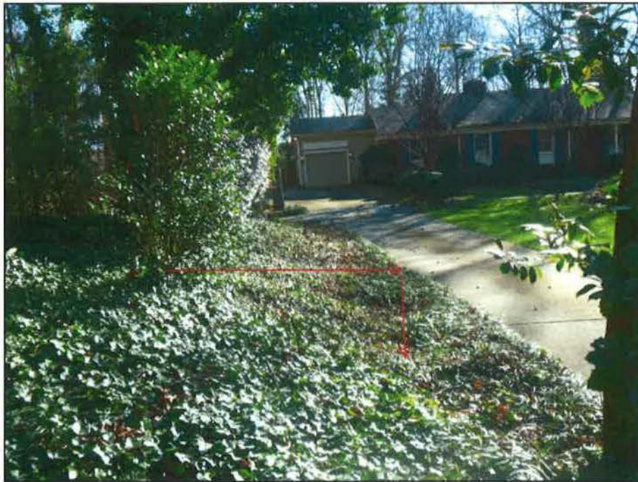
Figure 8: View of Northern Parcel Boundary, facing Southeast. Note elevation change along property line from grading during construction in the 1950s.
