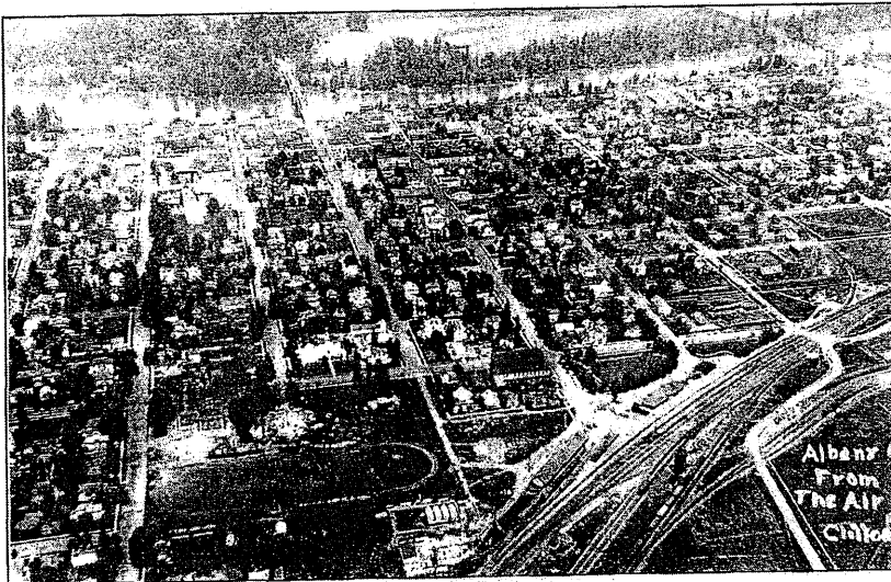
54) Looking north. Remains of demolition of old Albany College shown just above Central field. race track in lower left. Photo taken before construction of Pacific Boulevard. c. 1927
