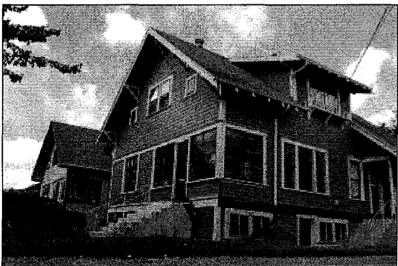
Photo 3: 10th and Maple, facing Northwest
