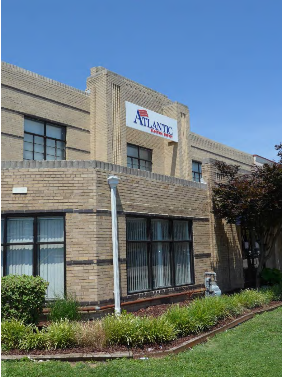
View looking northwest showing east façade from south 5 of 14
