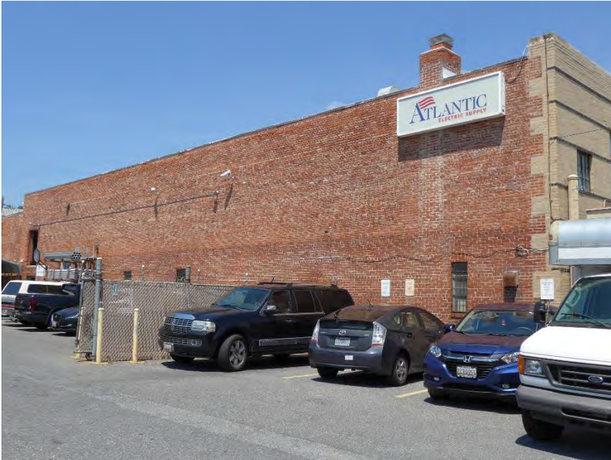
View looking northwest showing south elevation 4 of 14
