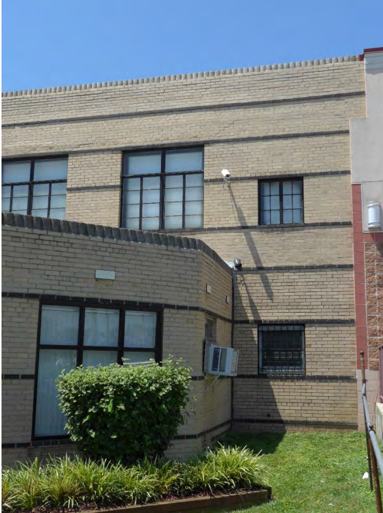
View looking west showing north end of east elevation 6 of 14
