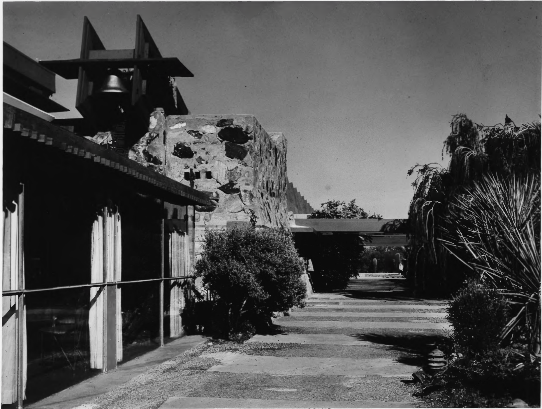
View northwest through the Pergola toward the Entrance Court (Dining Room, Kitchen, and Bell Tower to left).
