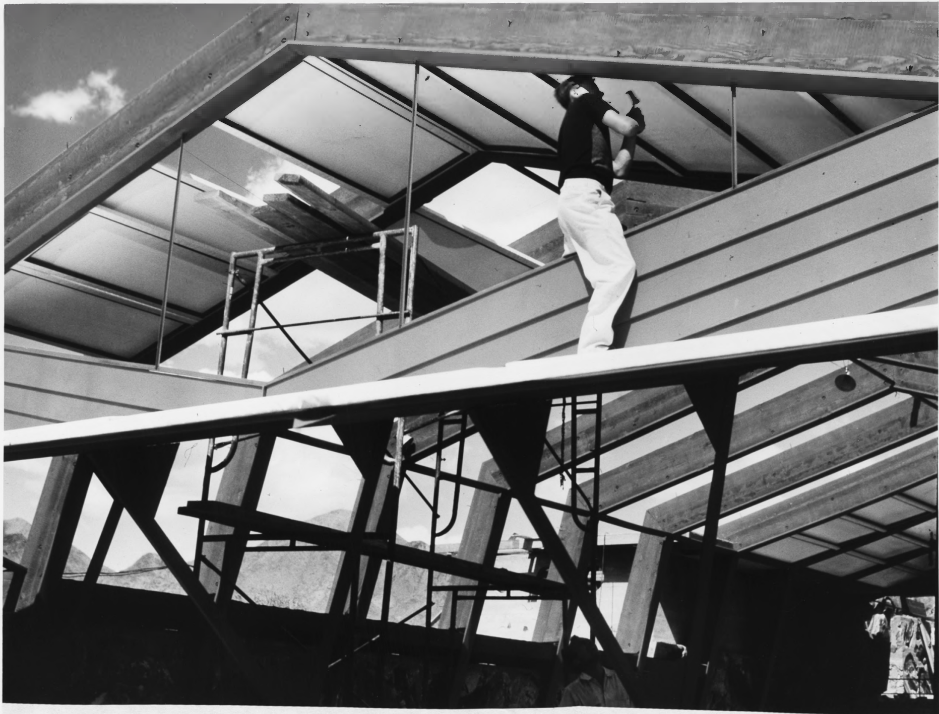
Construction Photo of Pavilion (1956).
