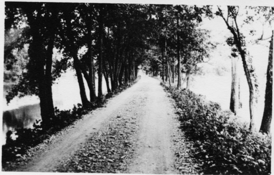
Tow Path Between Channahon and McKinley Woods (Contributed by SP-3)
