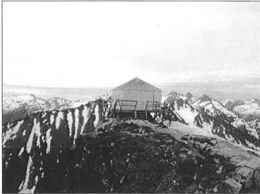
Figure 4. Green Mountain Lookout aerial view of south elevation and foundation damage, view to northeast, July 2, 2002. (HiLine Helicopters photograph).
