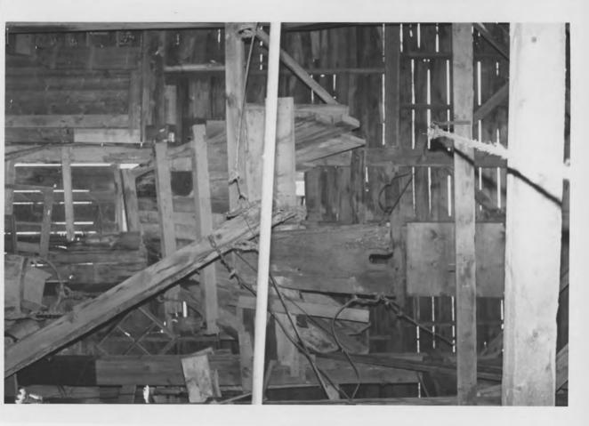
1. Snowbound Mine 2. Gold Hill, Colorado 3. Martha Poley 4. August, 1988 5. 2130 Vassar Drive, Boulder, Colo., 80303 6. Shafthouse interior showing head frame with notch for bailer chain, facing south Number 1
