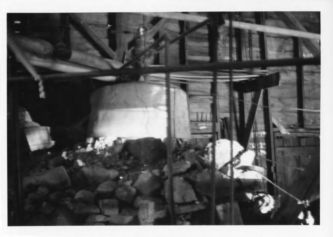
1. Snowbound Mine 2. Gold Hill, Colorado 3. Martha Poley 4. August, 1988 5. 2130 Vassar Dr. Boulder, Colo., 80303 6. Shafthouse interior showing insulation over boiler Number 1
